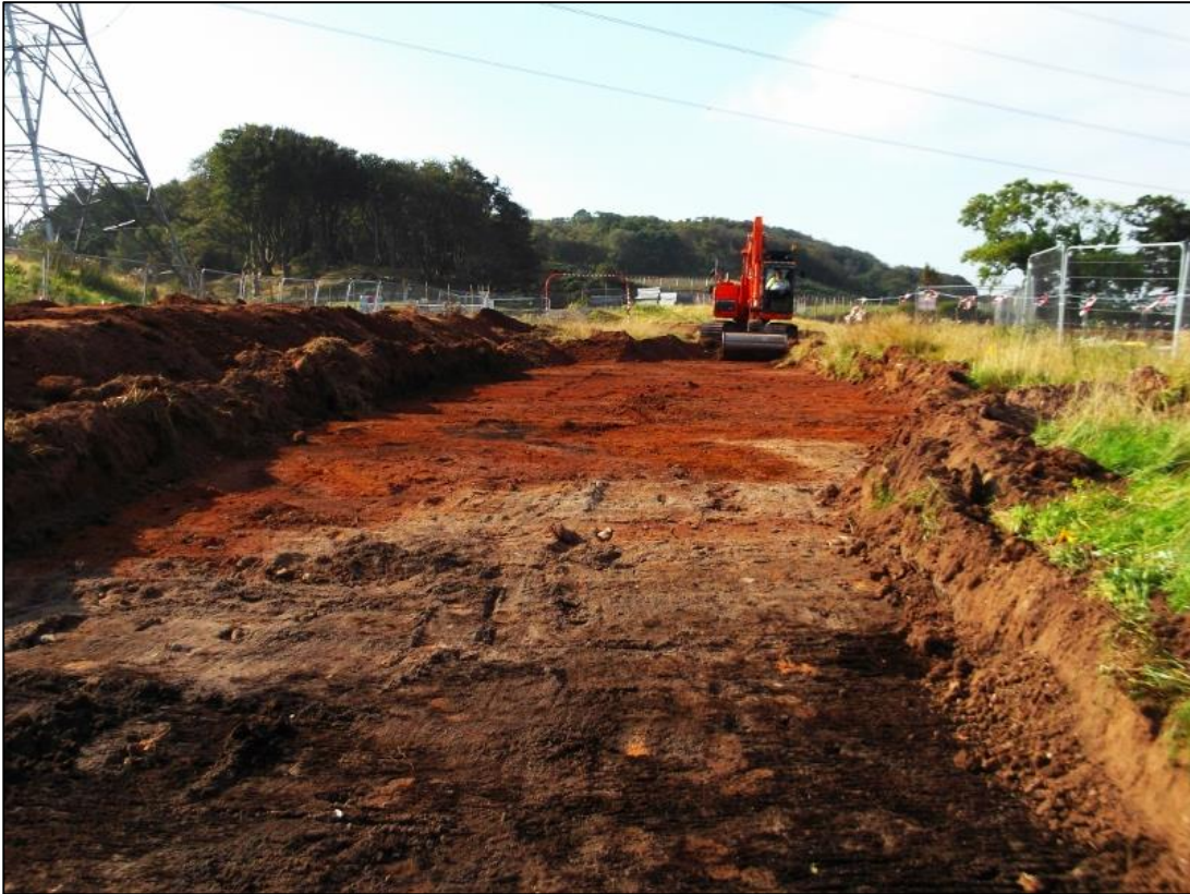
Figure 5: Area 1 under excavation. From the West
