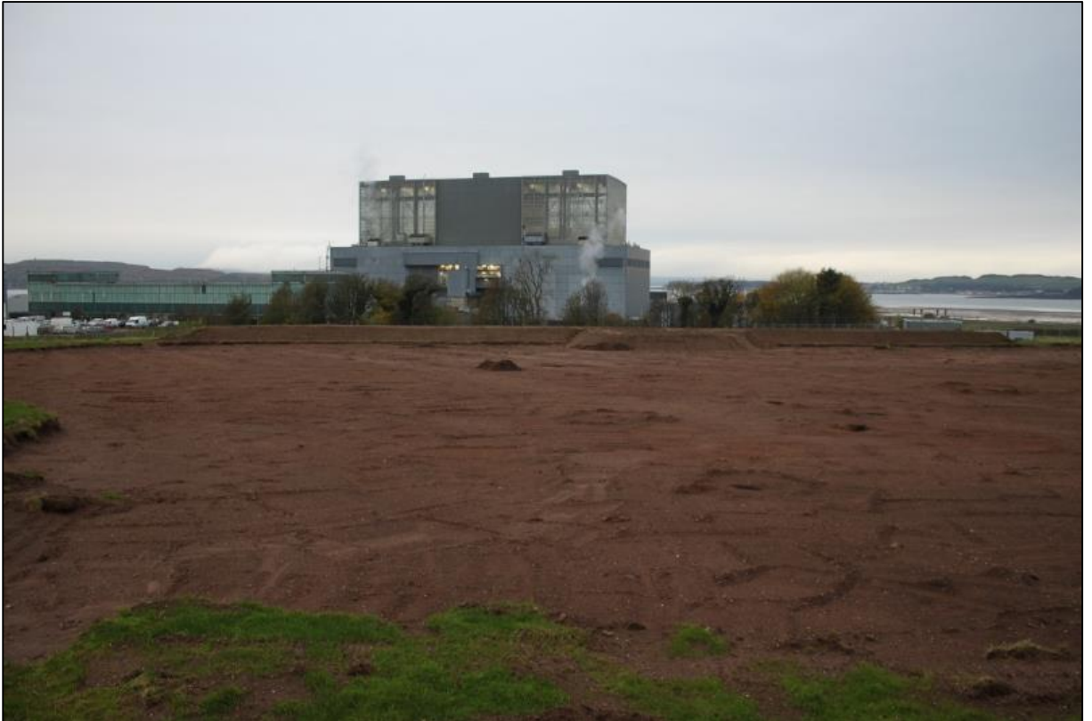
Figure 11: View of Area 2 after topsoil stripping from South West
