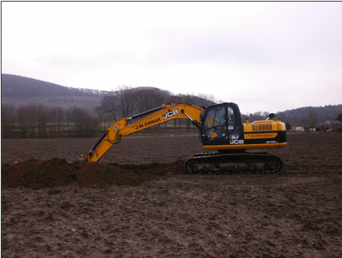
Figure 3a: Image showing the JCB160L excavating trench.
