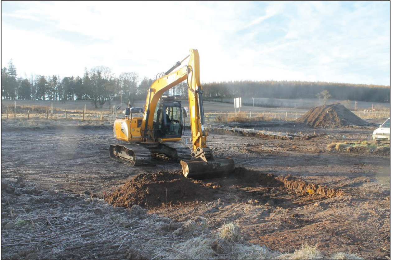
Figure 5a: Working shot of JCB145 excavating
