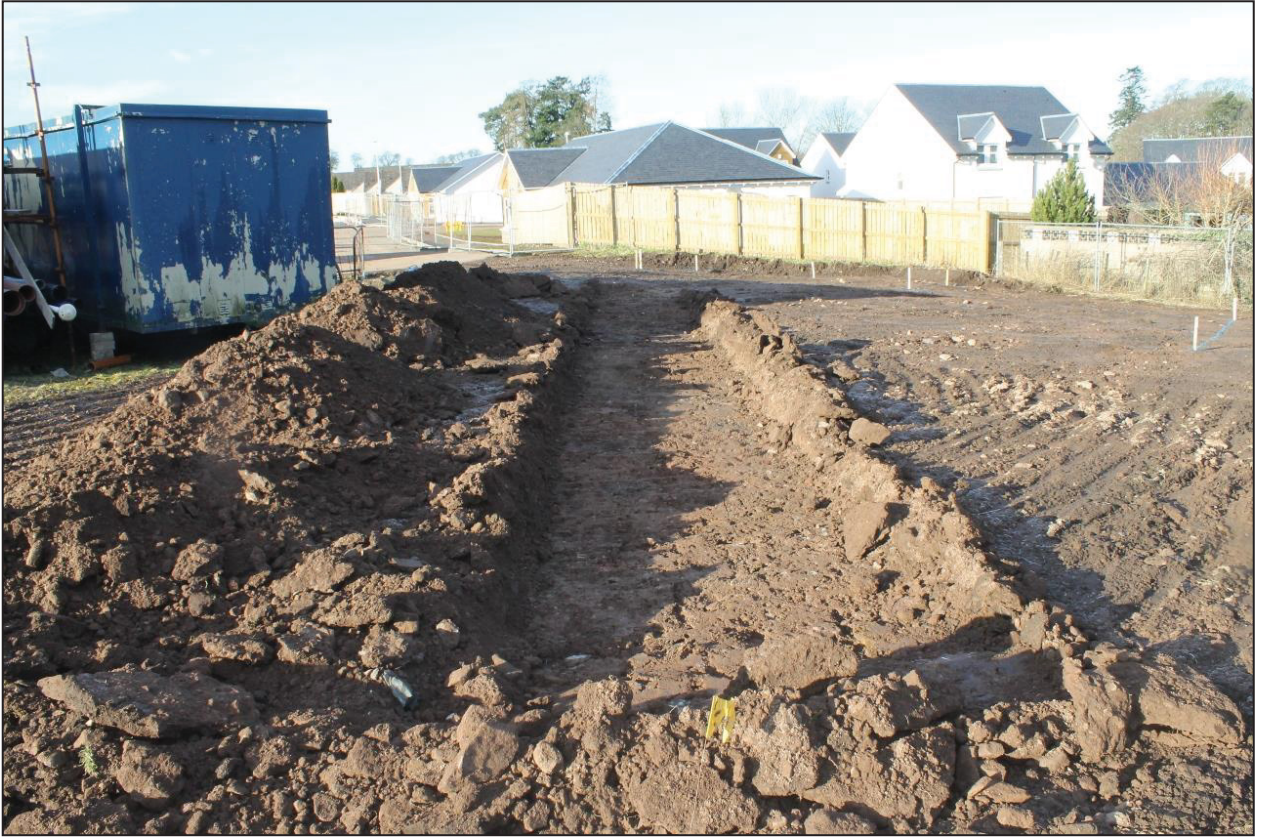
Figure 6a: View along Trench 1 demonstrating context (002)
