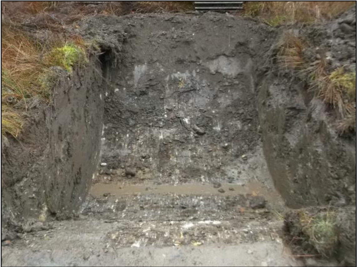
Figure 6a: Test Pit, south end Trench 50
