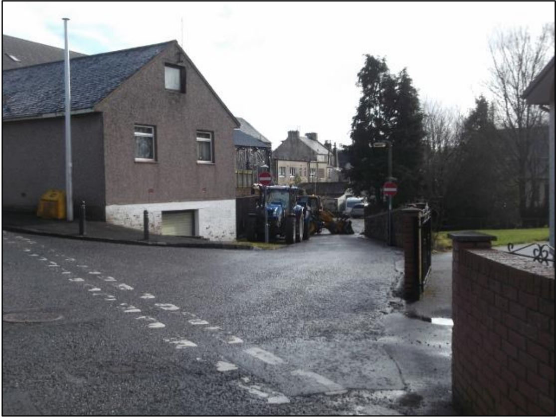
Figure 5a: Site Location, looking onto Castle Street (from WNW)
