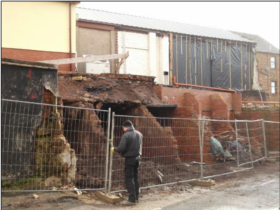
Figure 5b: Lock-ups, and rear of existing building (from W)
