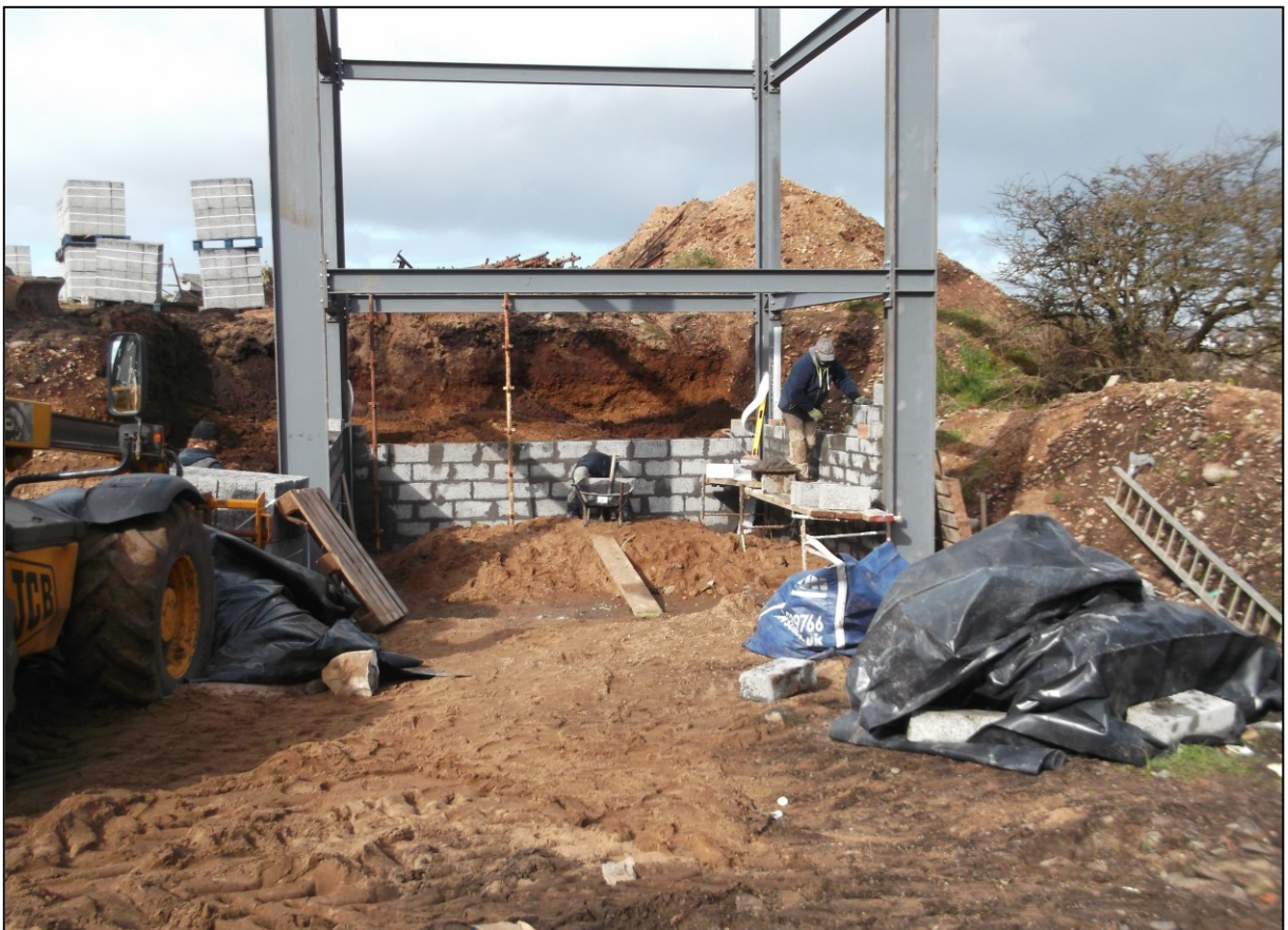
Figure 3b: Steel frame structure in the north-west corner
