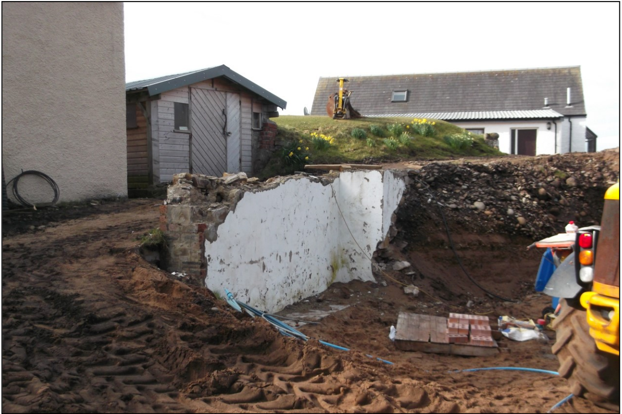
Figure 3a: Southern gable of demolished Dolphin Cottage
