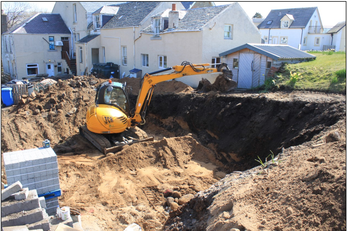
Figure 5b: Exposed subsoil (003)
