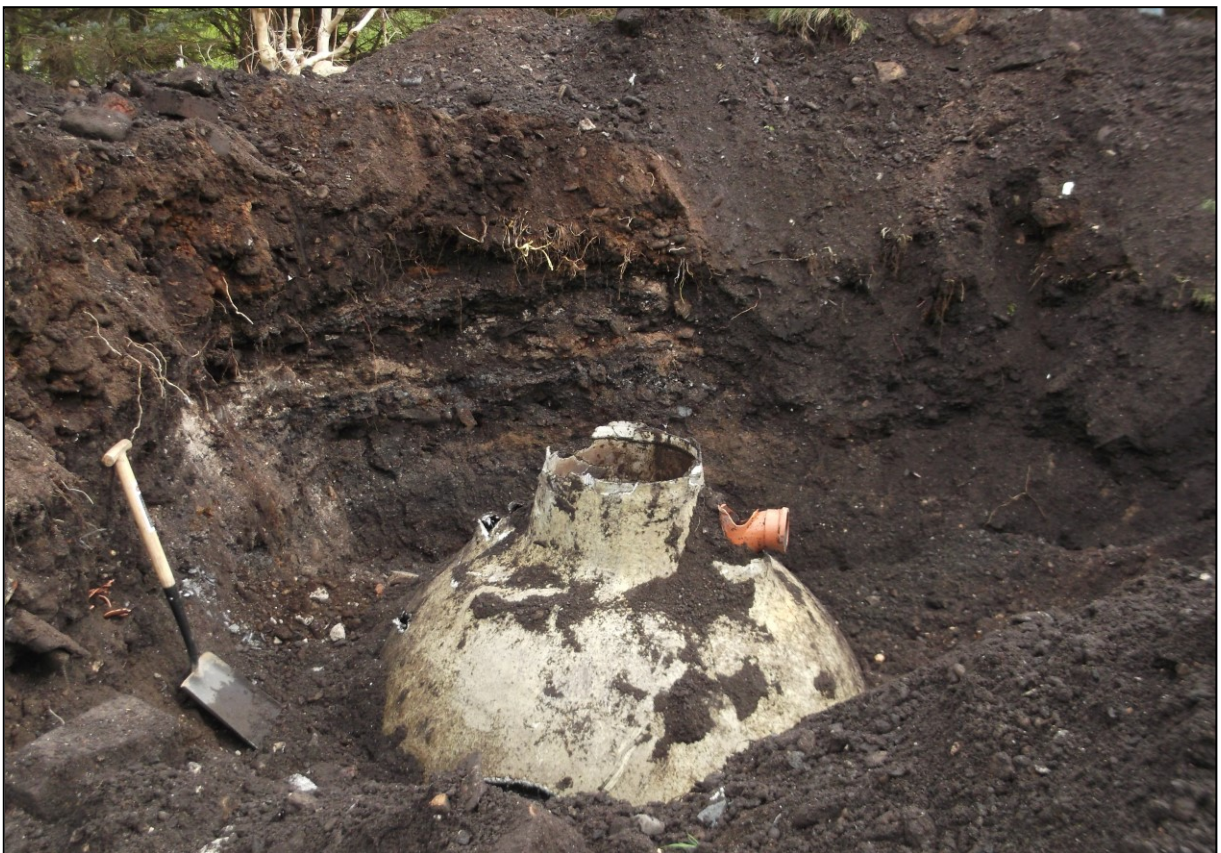
Figure 4b: Excavation for the removal of the existing septic tank
