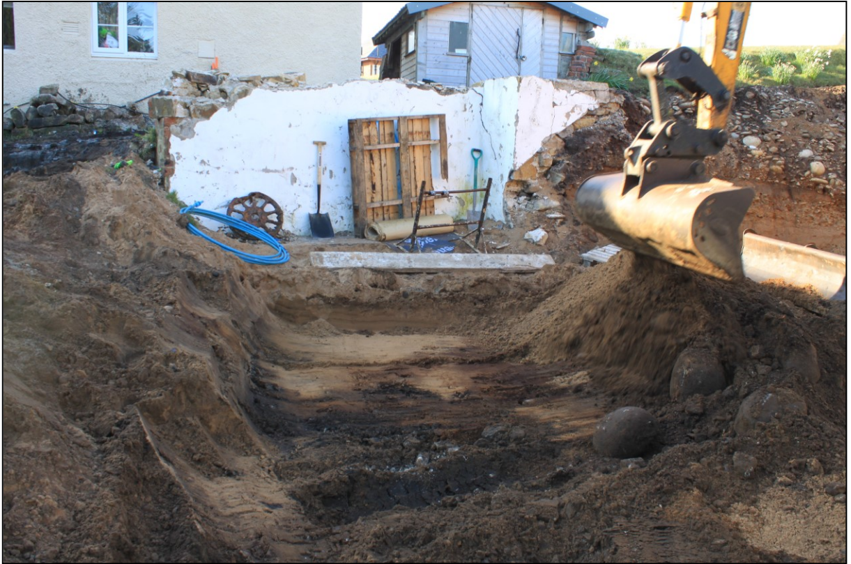
Figure 5a: Excavation in the footprint of the demolished Dolphin Cottage
