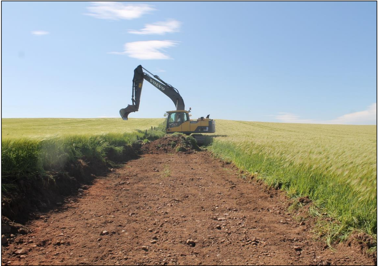
Figure 4a: Excavating the haul road showing context (001)
