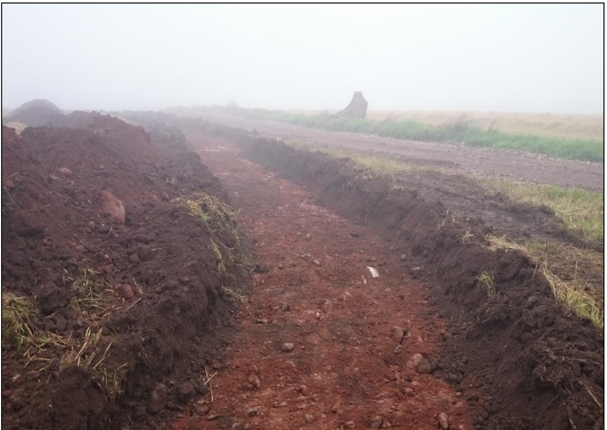
Figure 5b: Top WNW section of cable trench, showing context (002)
