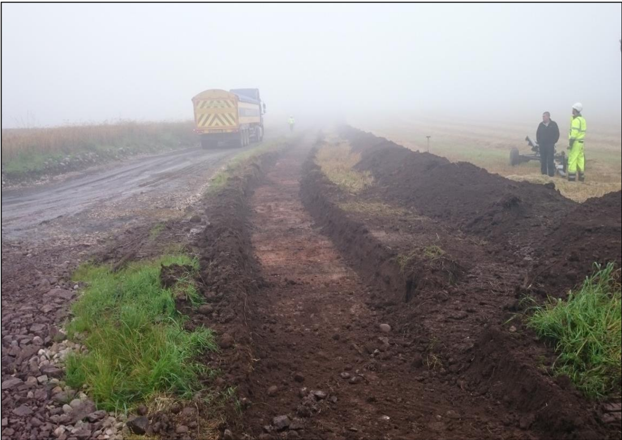
Figure 6b: Lower ESE section of cable trench
