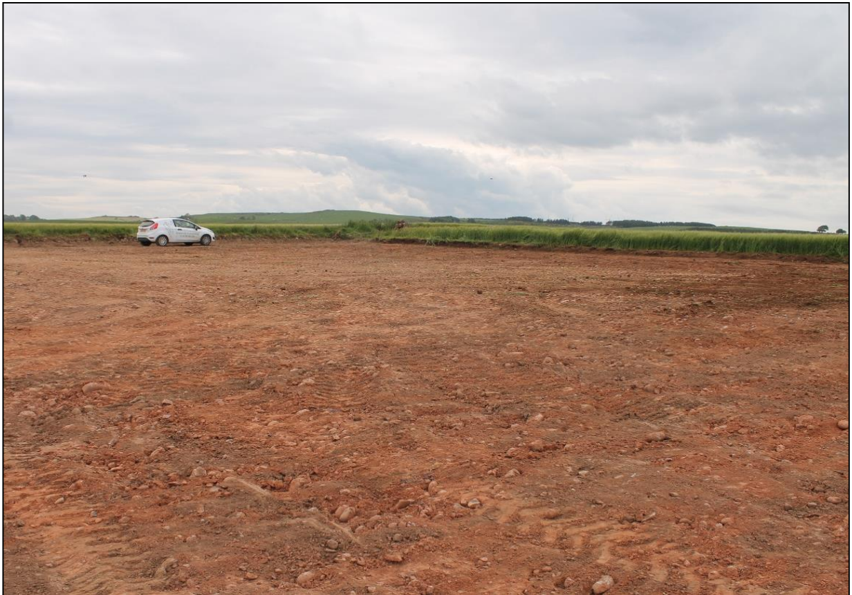
Figure 4b: Fully excavated crane pad area showing context (002)
