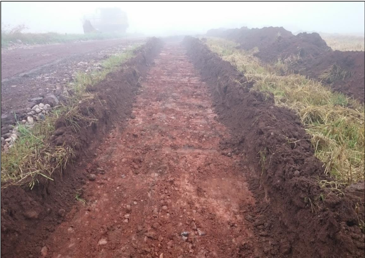
Figure 6a: Middle section of cable trench, showing context (002)
