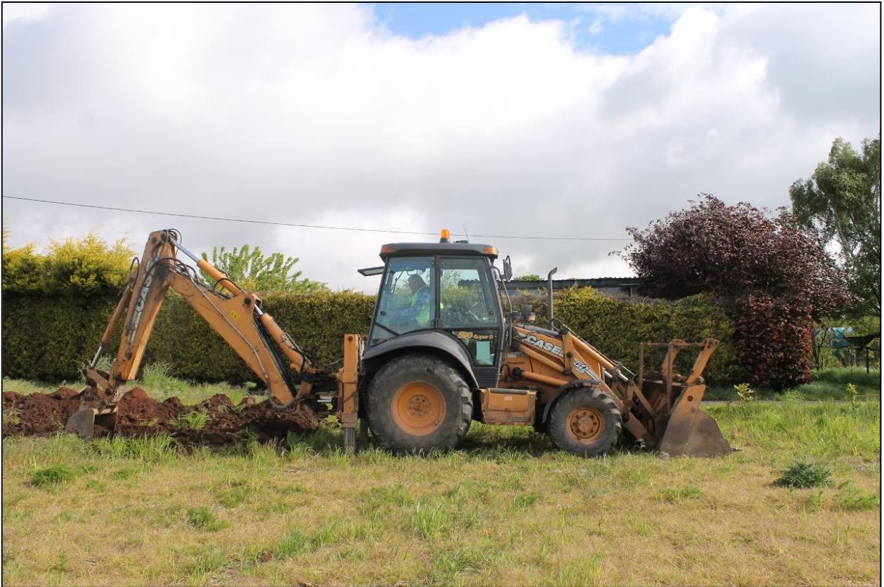
Figure 3a: CASE Series 2 (Super 590 R) excavating trench
