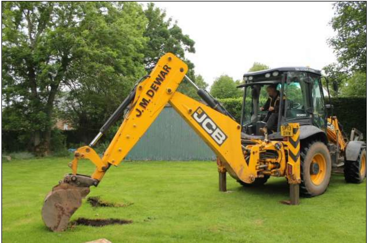
Figure 2a: Working shot of JCB 3CX excavating
