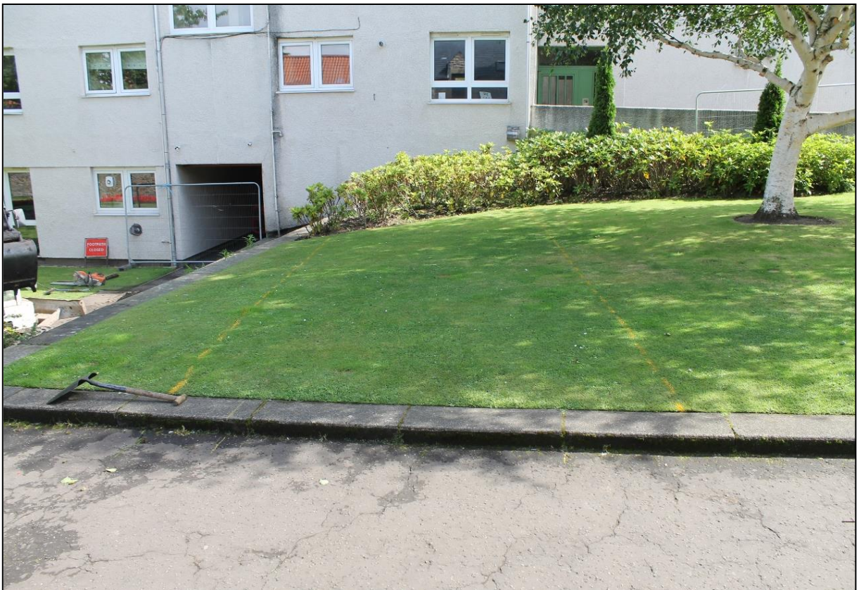
Figure 4b: Route of the upper southern area of the ramp
