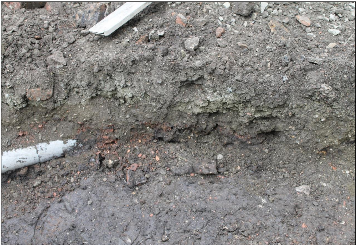
Figure 8b: South facing section of the north side foundation trench
