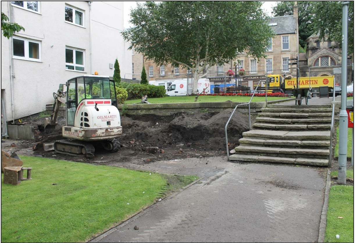
Figure 4a: Removal of the modern retaining wall and flower bed
