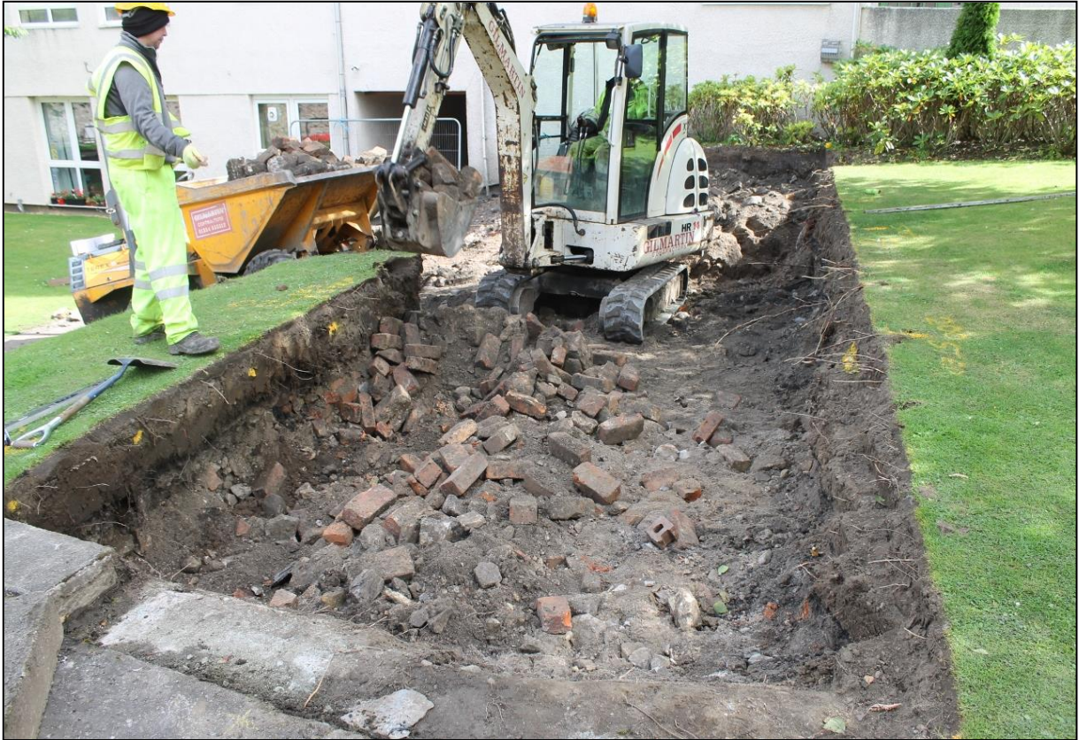
Figure 5a: Demonstrating the substantial quantity of red brick in the underlying deposit
