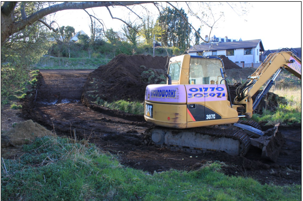
Figure 4b: Access road stripped to topsoil
