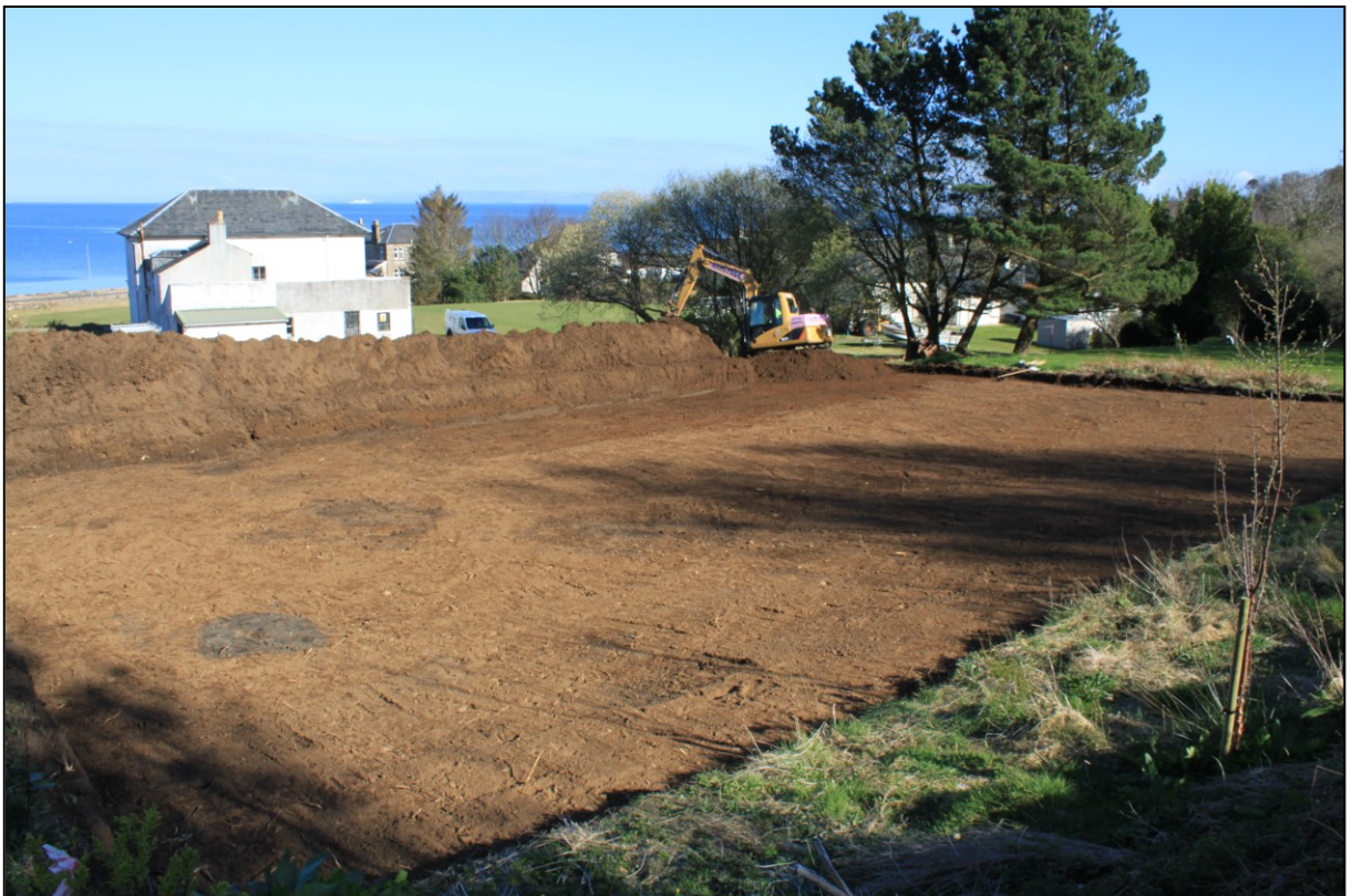
Figure 3b: The development area stripped to subsoil
