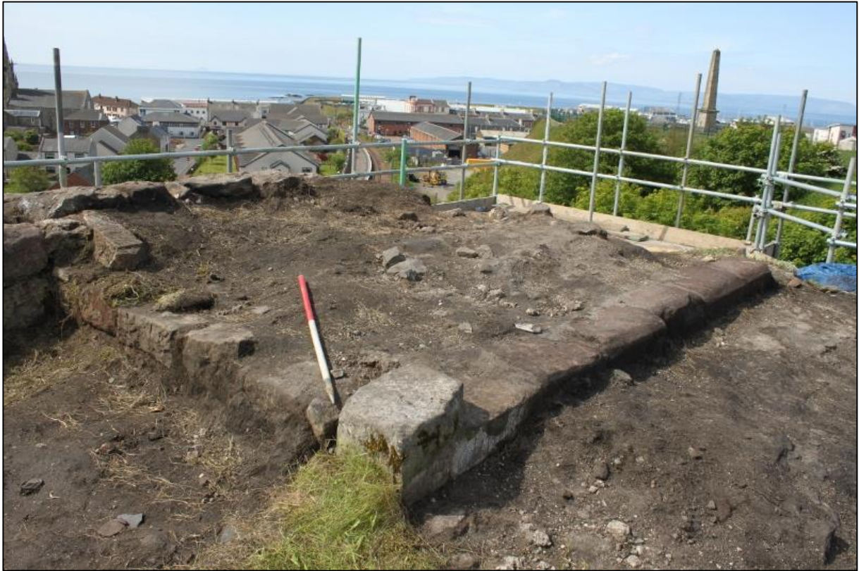
Figure 2a: Vegetation stripped, revealing walls [002] to right and [003]/[007] to left, containing overburden (005)
