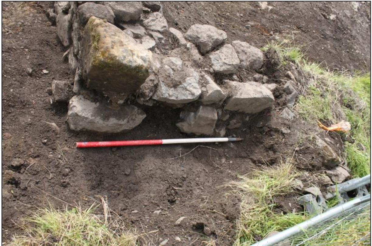
Figure 37: Structure E – External northwest facing elevation
