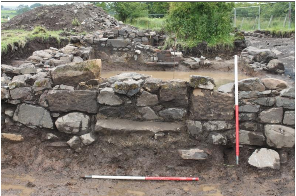
Figure 31: Structure B.2 – Blocked doorway in wall [033] from the northeast
