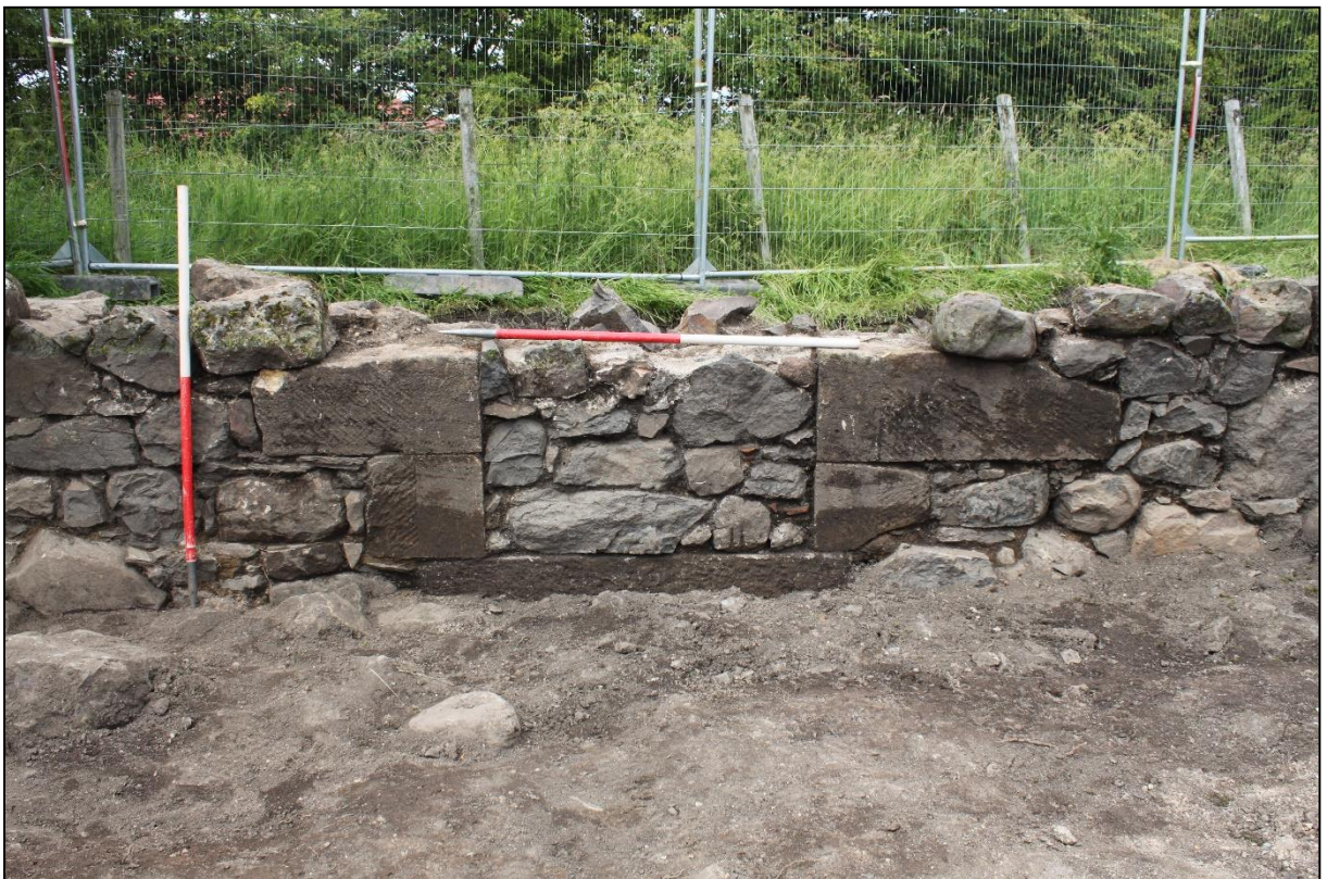
Figure 10: Structure A – Blocked doorway in wall [005]
