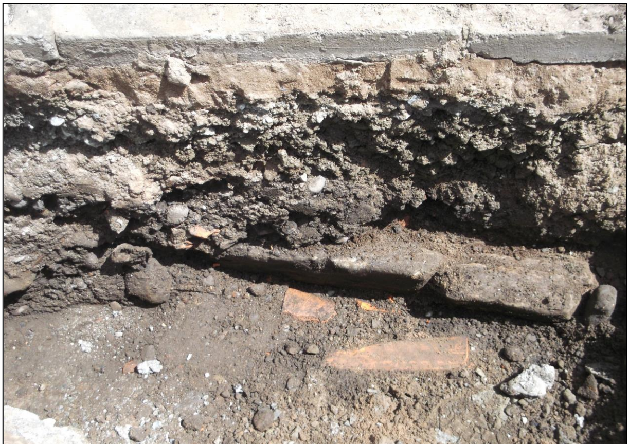
Figure 7: The eastern face of culvert (005) with tile drain within, note made ground over
