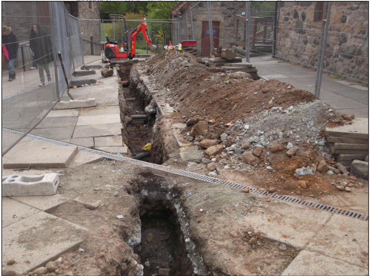
Figure 6: Service track excavated showing multiple existing services
