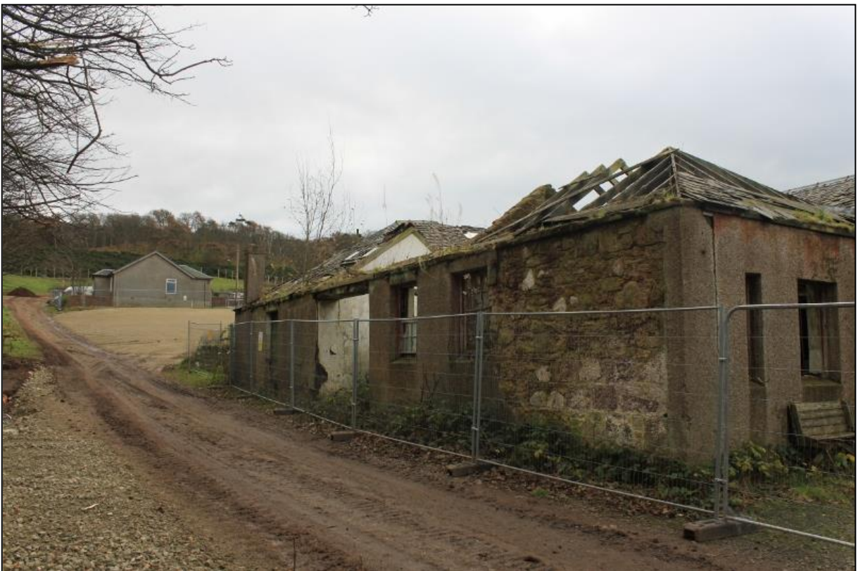
Figure 8b: NE Elevation, structure 'j'
