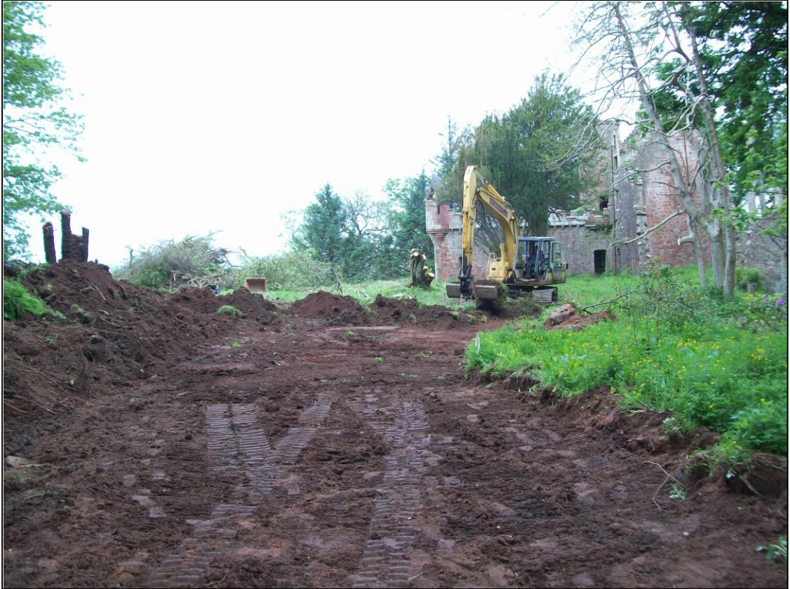
Figure 2a: Looking west along line of access road, post-excavation
