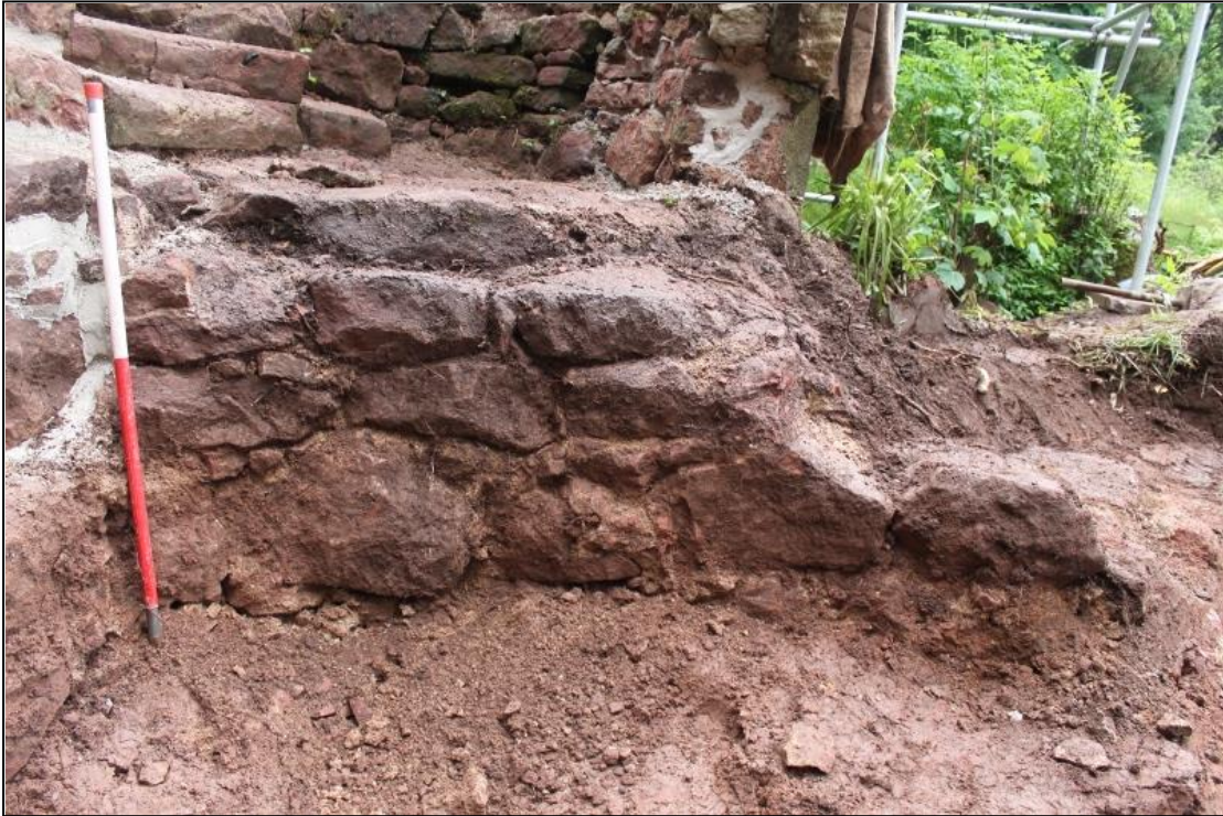
Figure 8a: SW-Facing Revetment of NE Stair Tower, showing Mortared Mass (211) ('Consolidation Later') overlying earlier wall (212)
