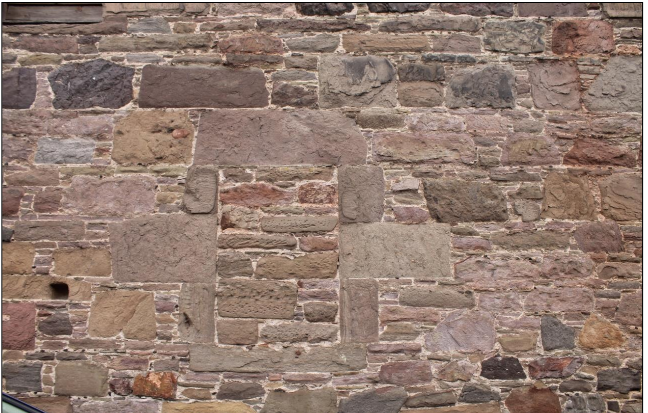
Figure 5b: Window (i) West elevation
