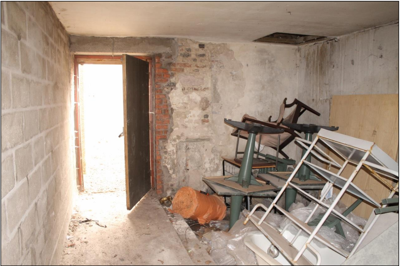
Figure 10a: Store room
