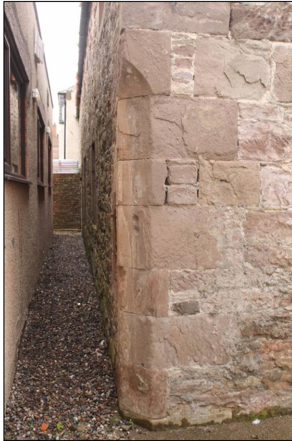
Figure 7a: Detail on the east corner of the North elevation
