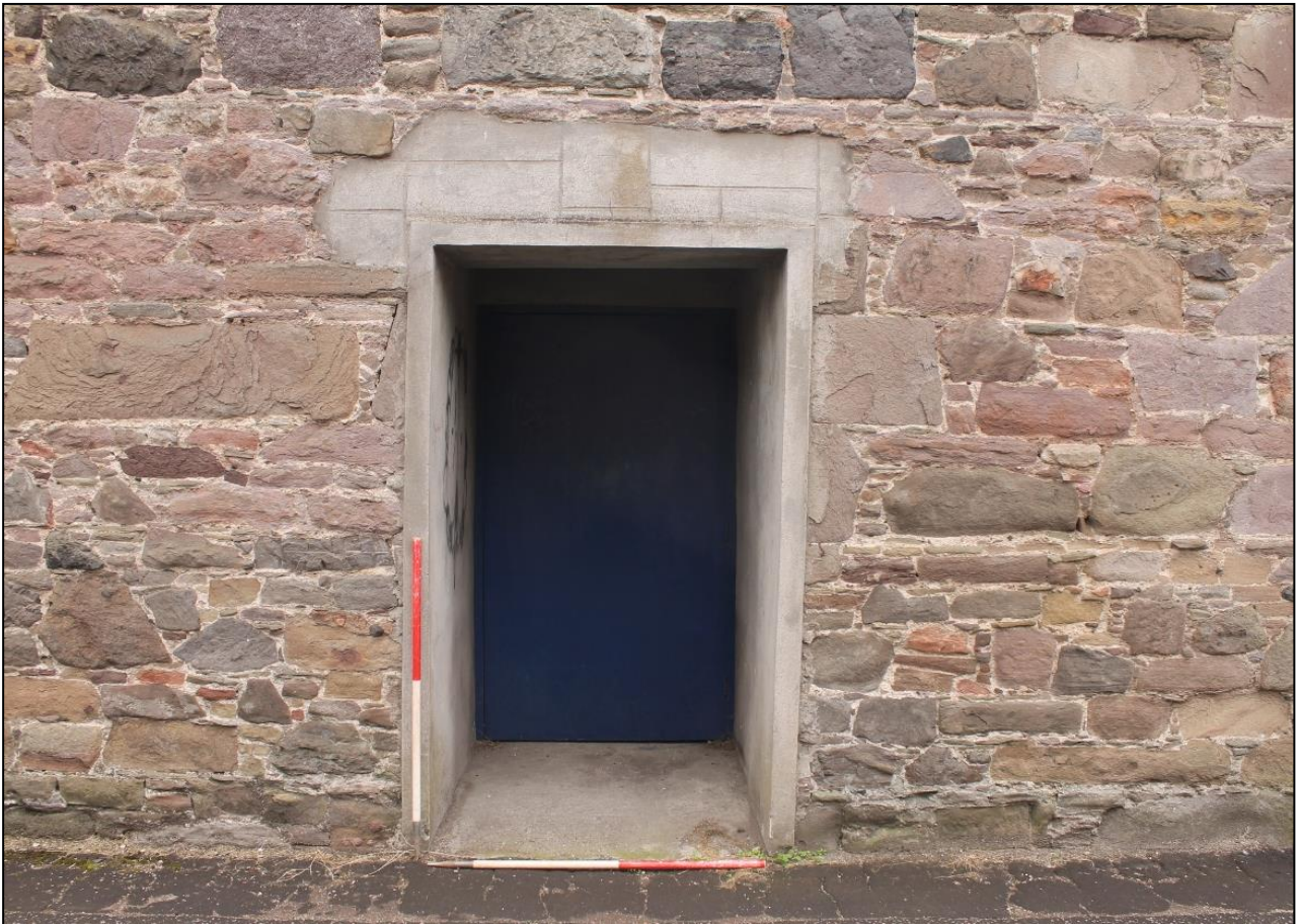
Figure 6a: Doorway (iii) West elevation
