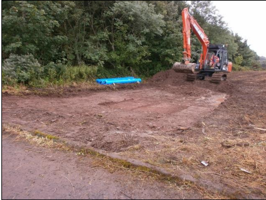
Figure 2a: Eastern stripped area of Siemens Compound Strip
