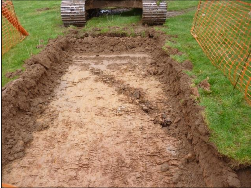
Figure 4a: Field drain [3006], Test Pit 10, Area 3
