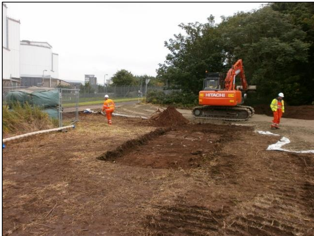
Figure 2b: Showing two smaller areas stripped to the west (Siemens Compound)
