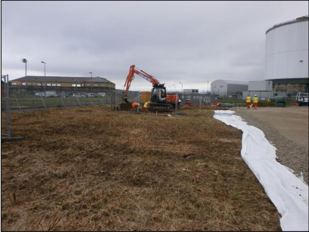
Figure 3a: General shot of compound area & location of investigative trench
