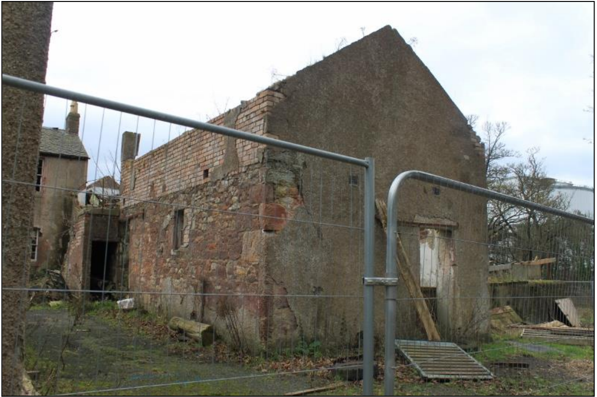
Figure 6a: Structure 'e:' Detail of quoins on E elevation taken from the W
