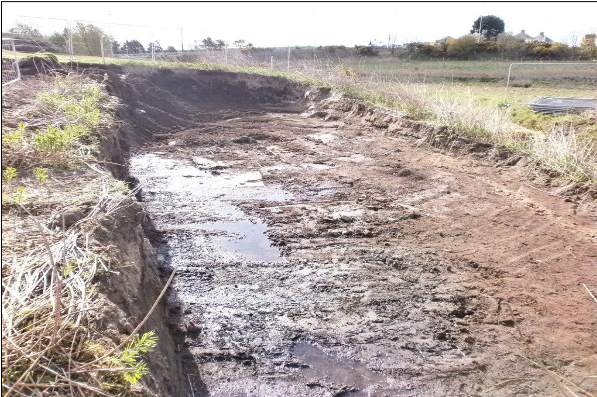
Figure 5b: Working shot of excavation in strip 1 (phase 2)
