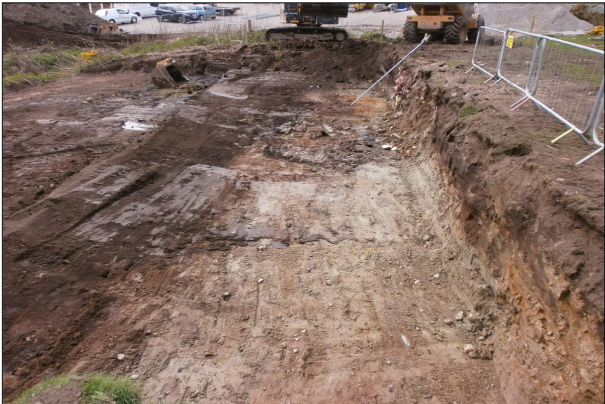
Figure 7b: Working shot of excavation in strip 2 (phase 2)
