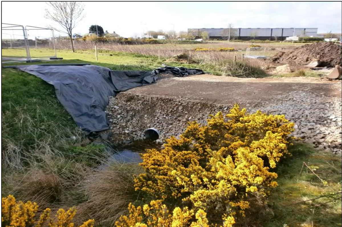
Figure 5a: Working shot of culvert construction (phase 1)
