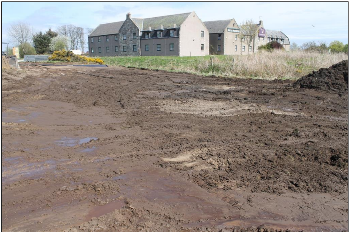
Figure 4b: Working shot of completed area stripping at N end (phase 1)
