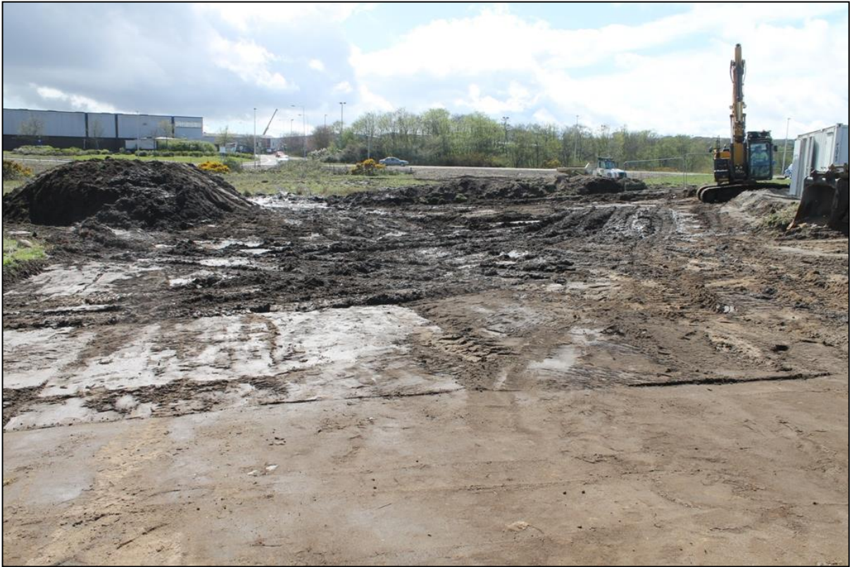
Figure 4a: Working shot of completed area stripping at S end (phase 1)
