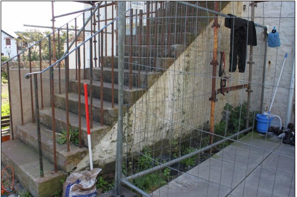
Figure 5b: Base of External stair, showing cast iron handrail
