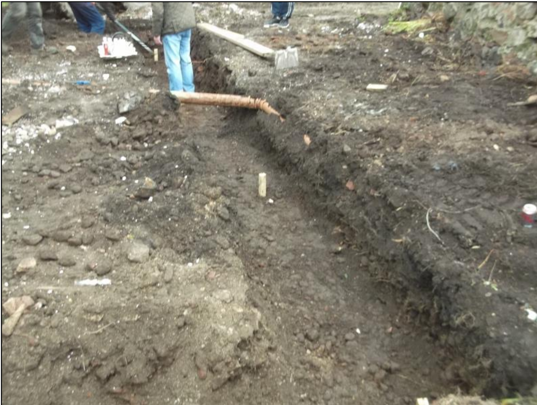
Figure 9b: (003) at base of trench in 'b'
