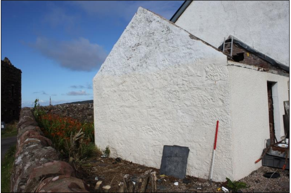
Figure 3a: Looking NW towards S extension ('Room a'), prior to demolition
