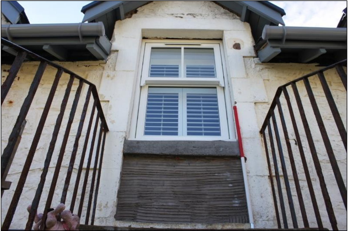
Figure 6a: Blocked doorway at first floor level, central bay, E elevation
