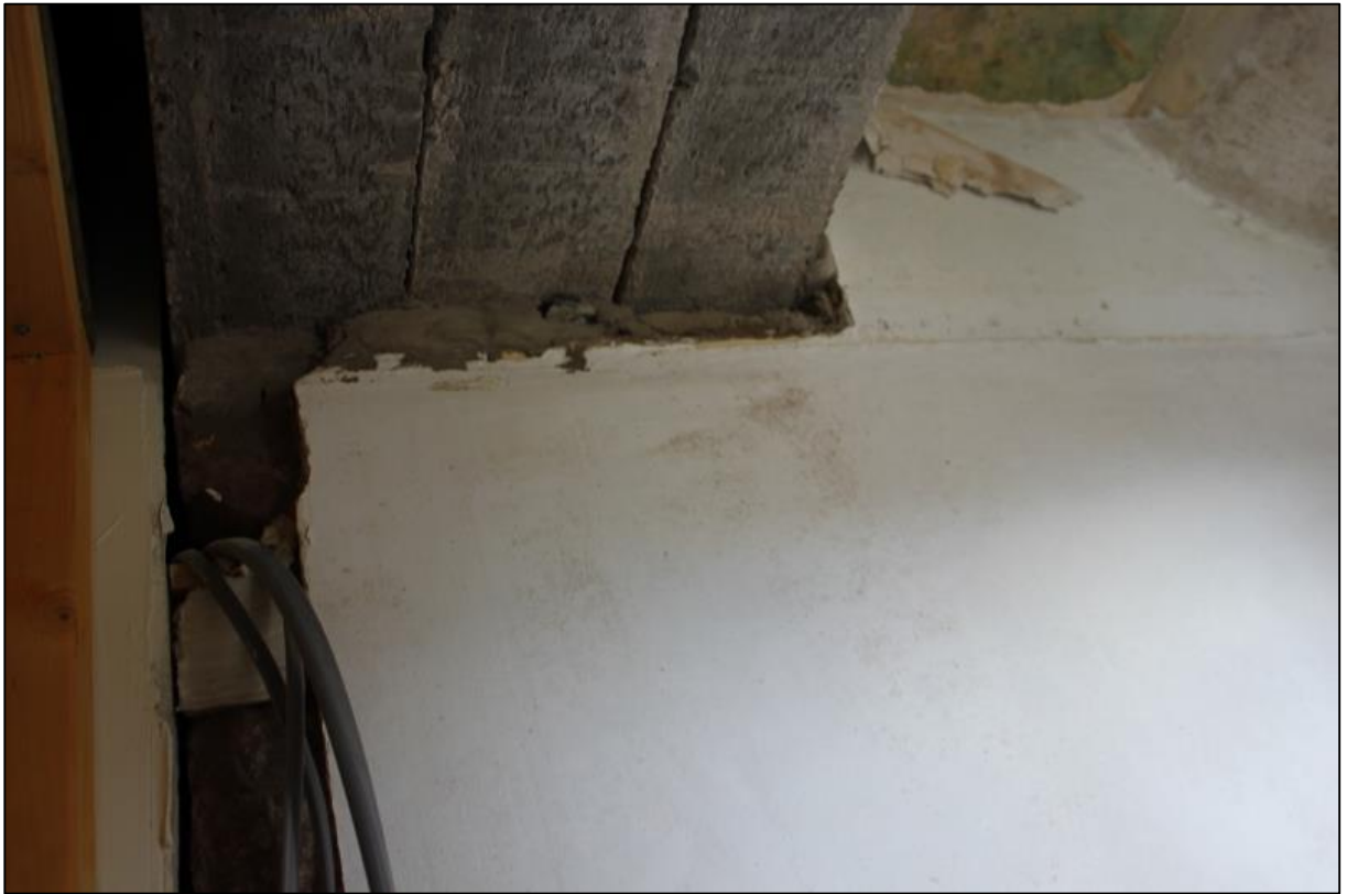
Figure 7a: Concrete lintels consolidating external stair at junction with main building
