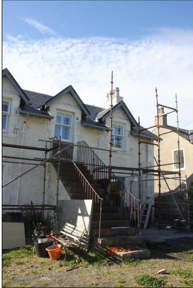
Figure 5a: External Stair abutting rear E elevation of house
