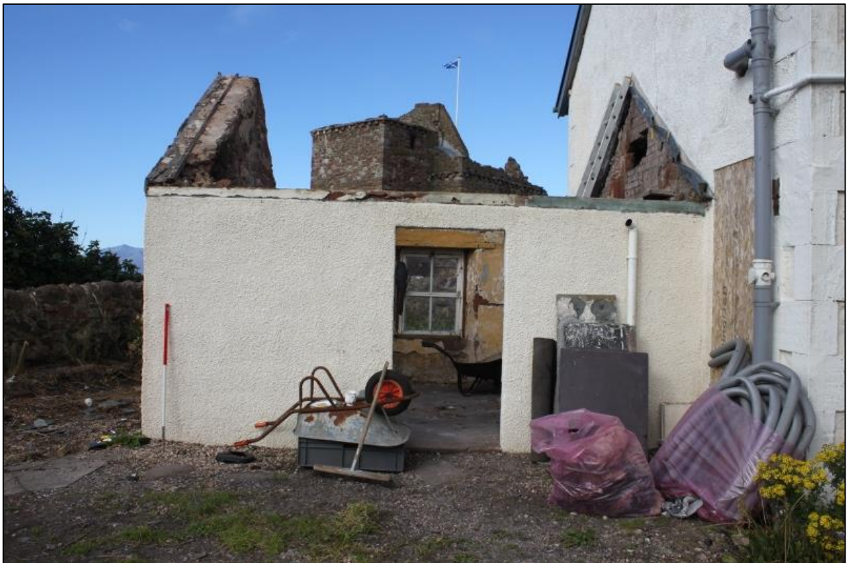
Figure 2b: Looking W towards S extension ('Room a'), prior to demolition
