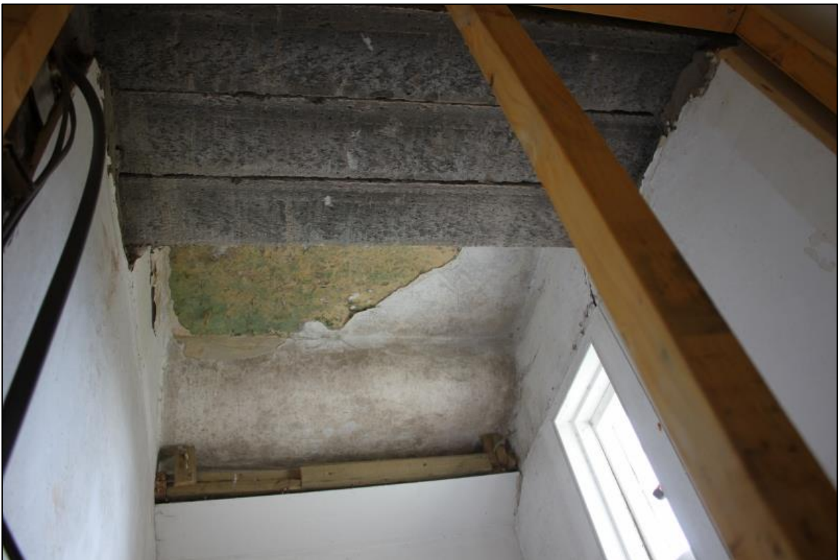
Figure 6b: Concrete lintels consolidating external stair at junction with main building
