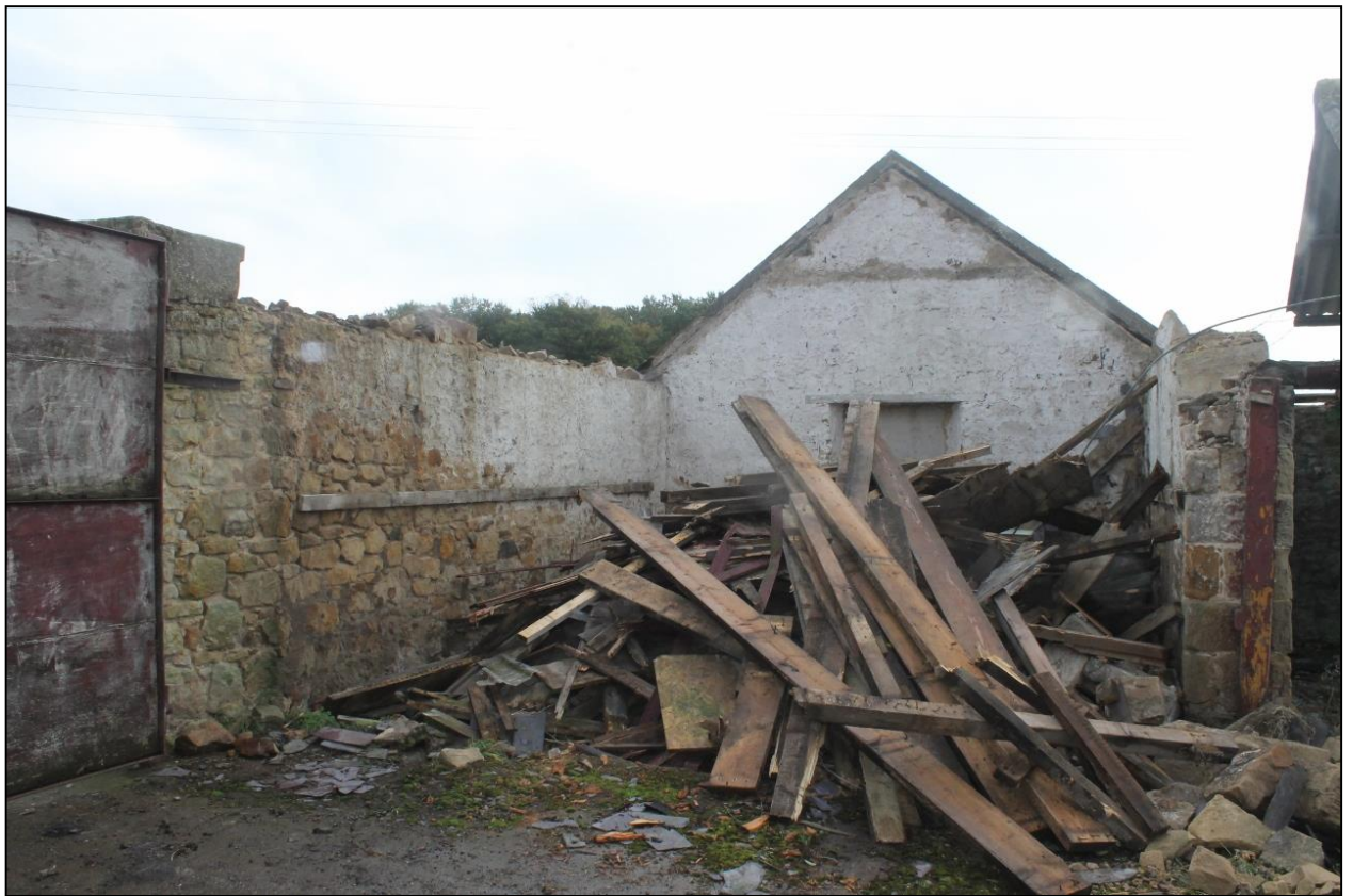
Figure 6b: Building A; interior
