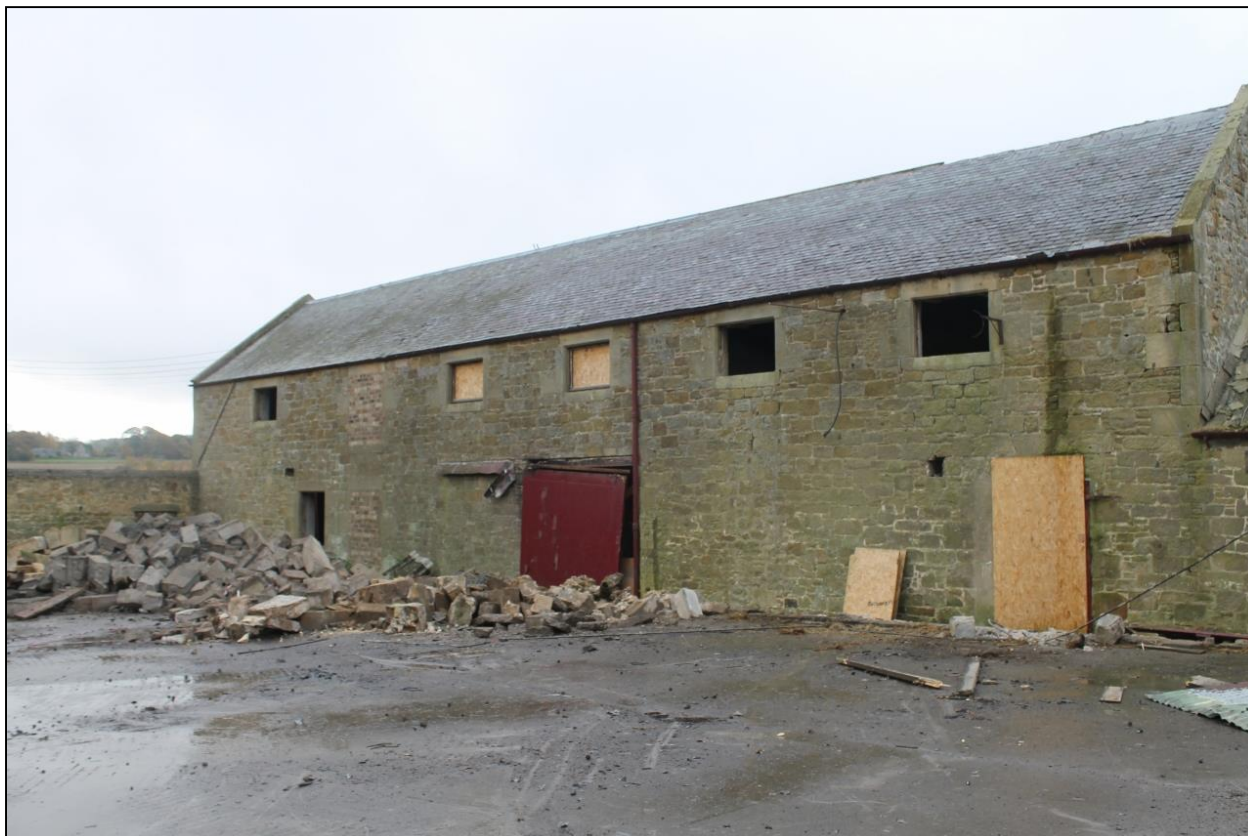
Figure 8a: Building E, East elevation
