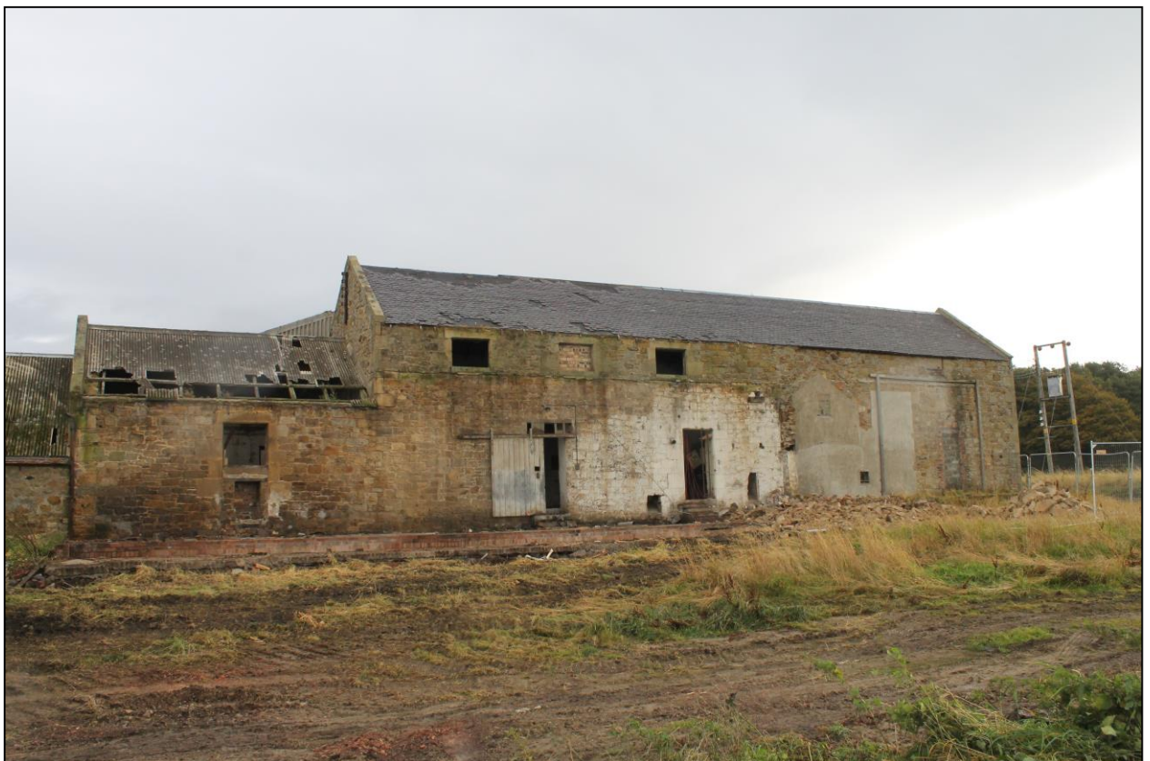
Figure 7b: Building E; West Elevation
