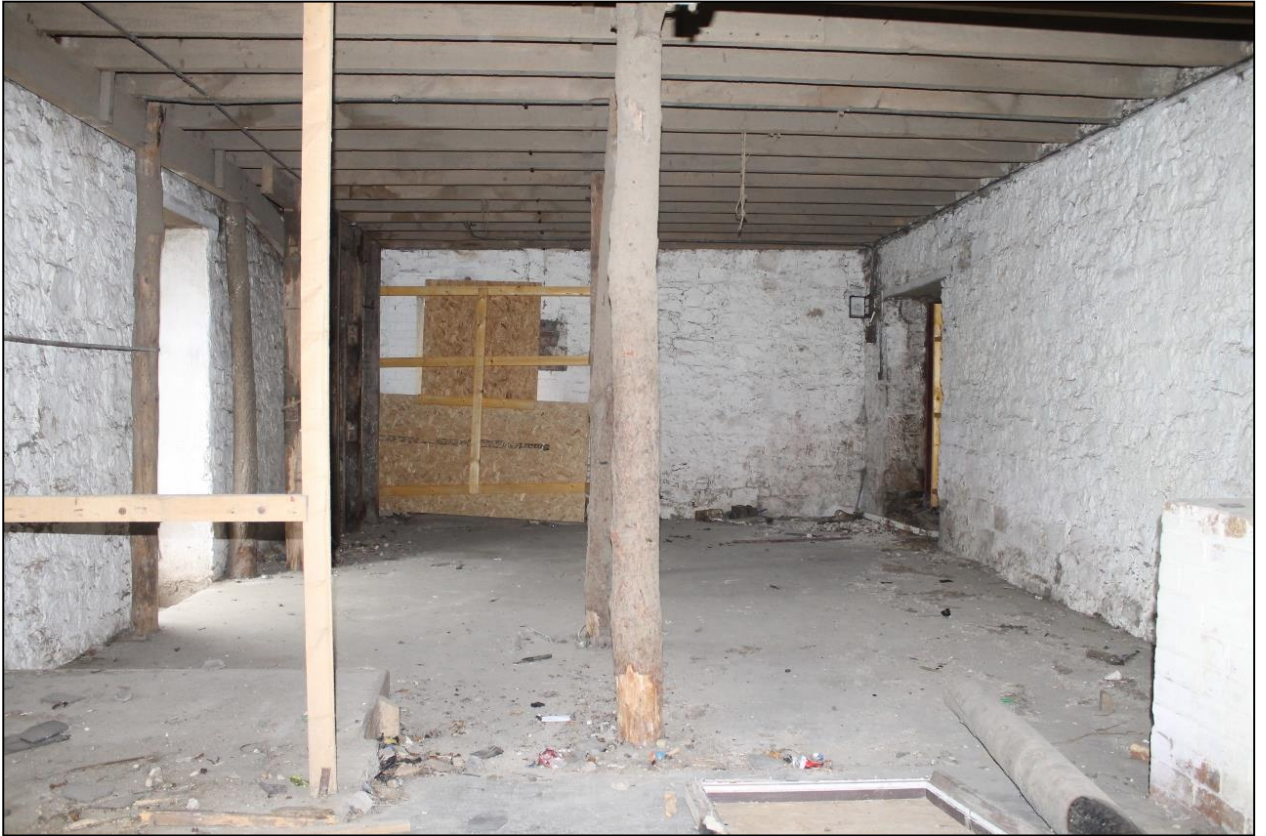
Figure 9a: Room 2, Building E; view to the northern end
