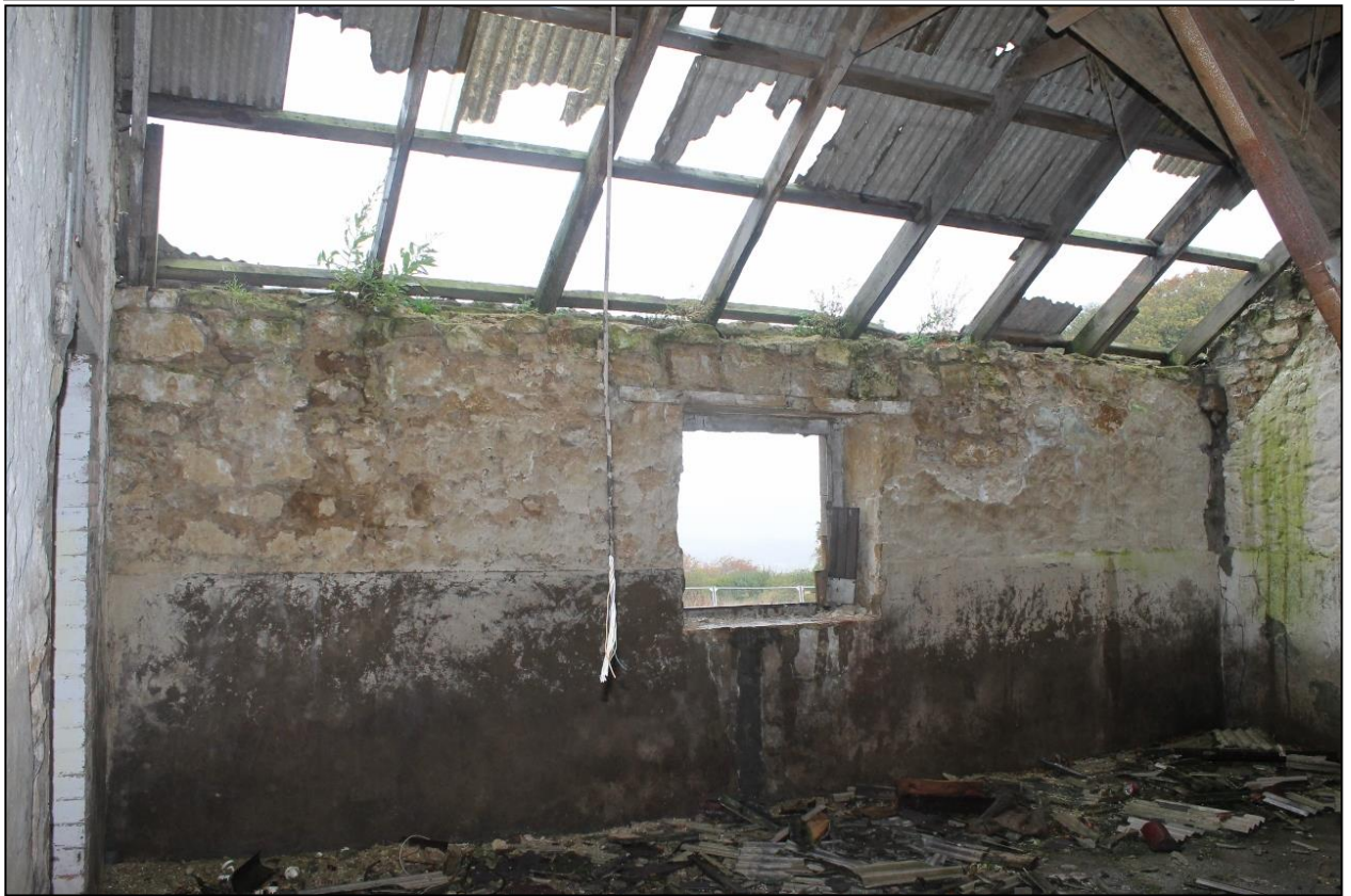
Figure 10a: Building F; west elevation
