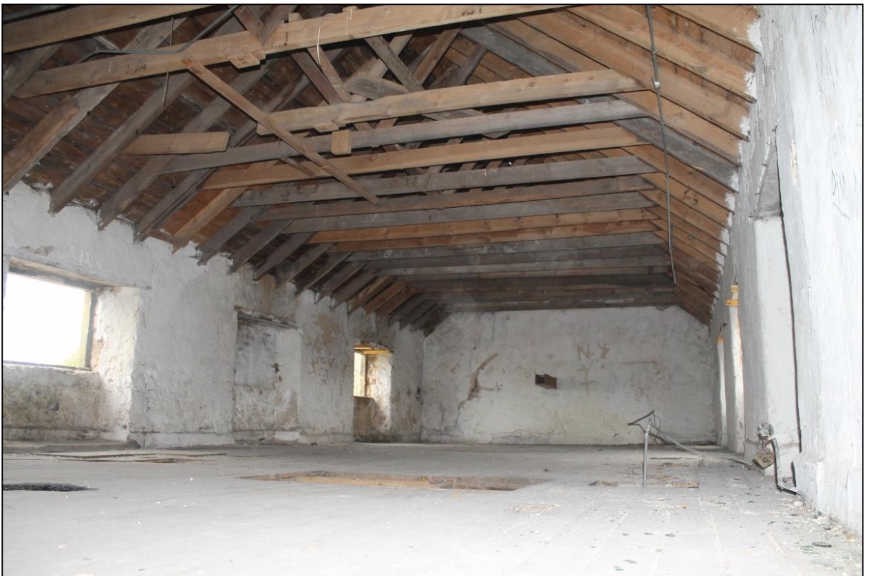
Figure 9b: 1 st floor of Building E
