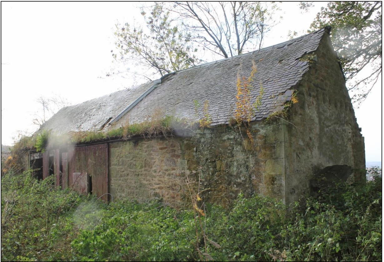
Figure 14a: Building O; east elevation
