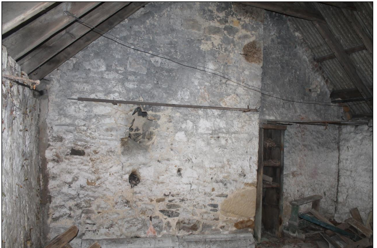
Figure 10b: Building G; chimney breast in south room
