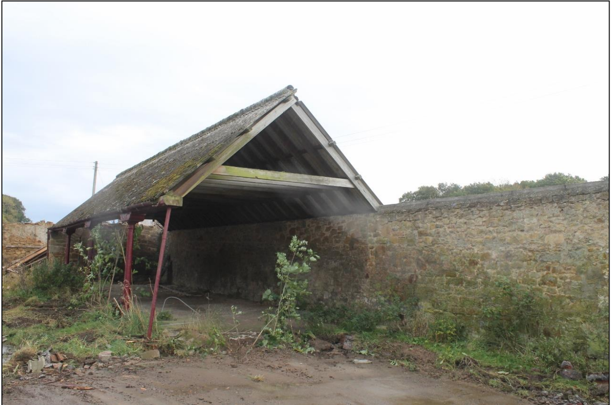
Figure 7a: Building B
