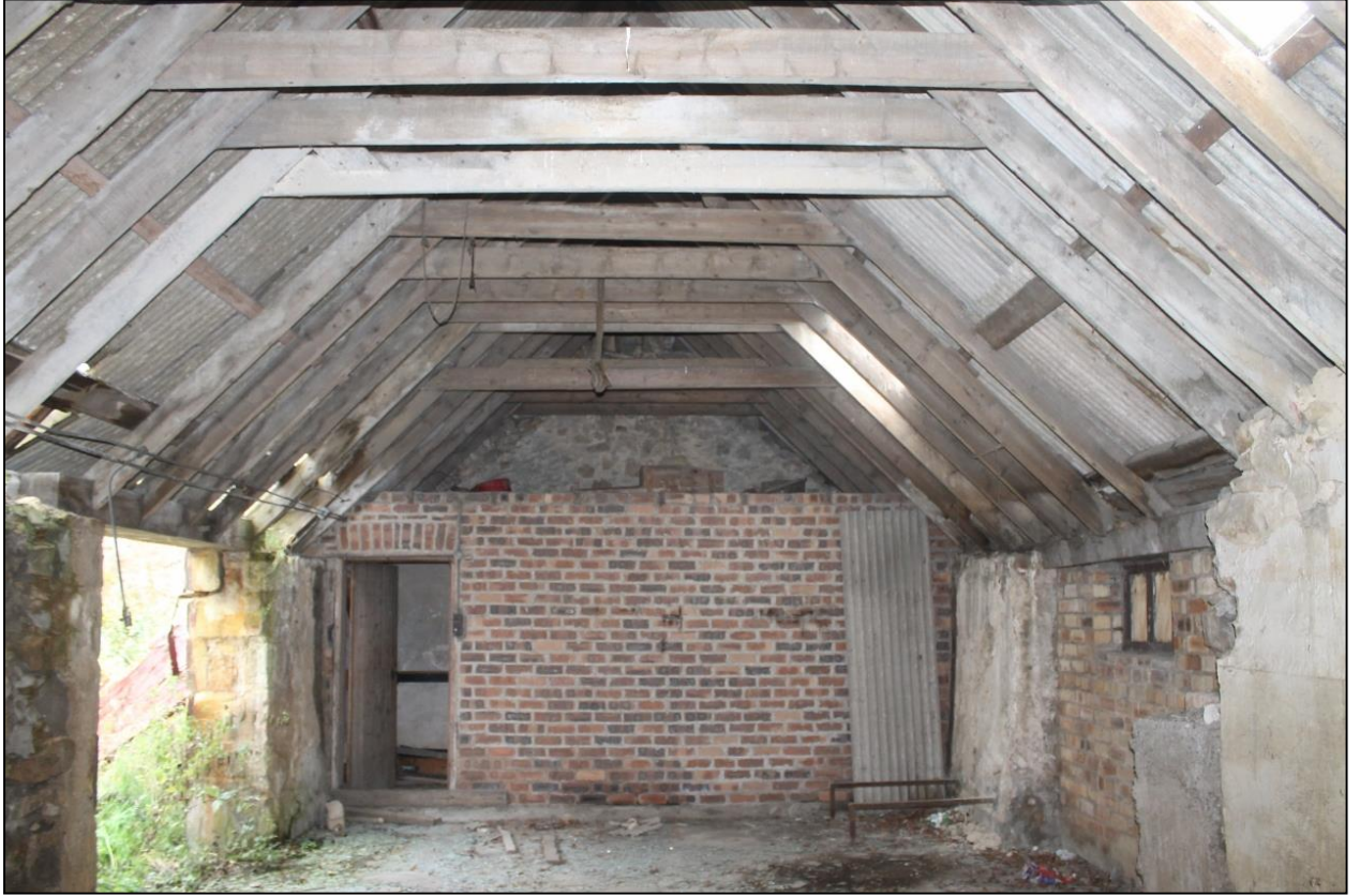
Figure 11a: Building G; north room showing modern brick dividing wall
