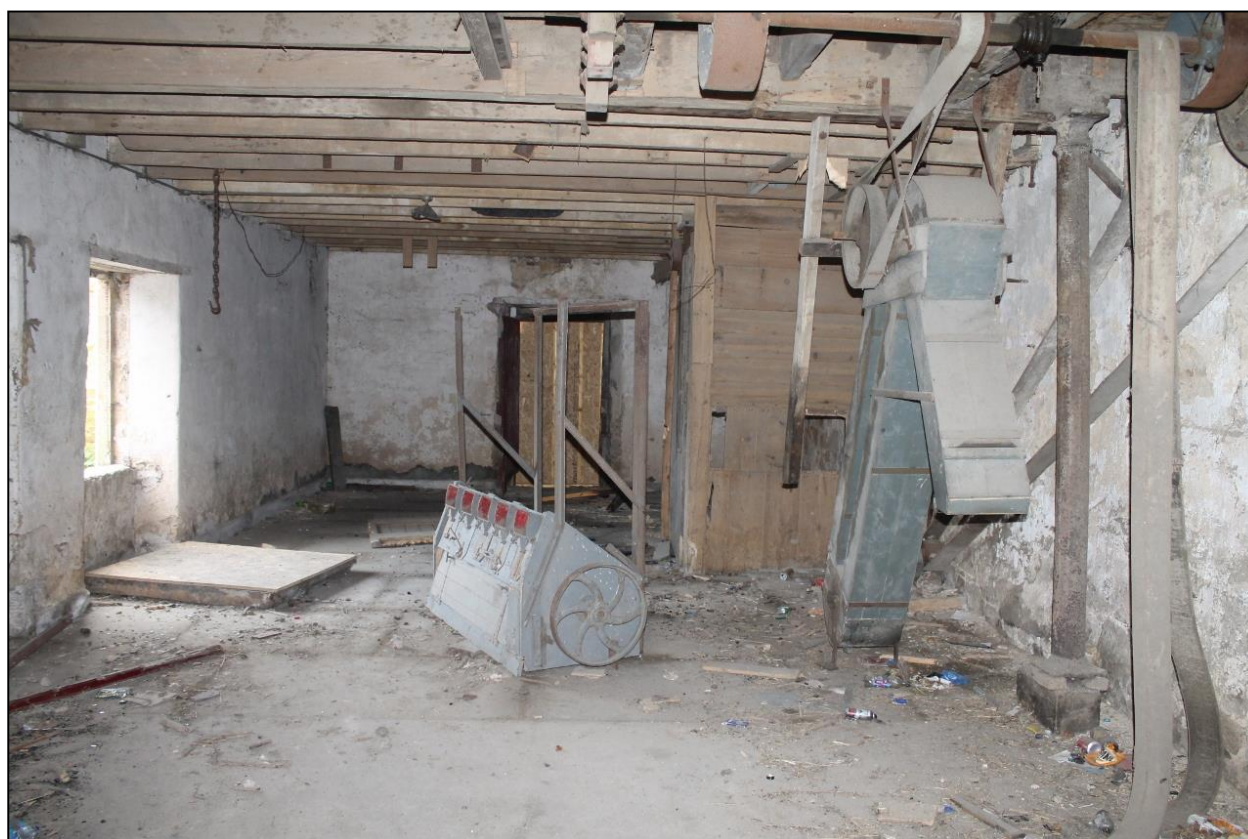
Figure 8b: Room 1, Building E; view to the southern end
