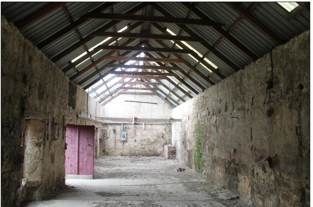
Figure 12b: Building K; view to the west end of the building
