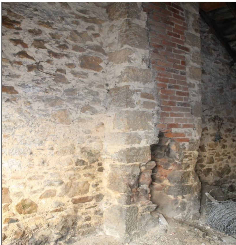
Figure 13b: Building O; chimney in central room
