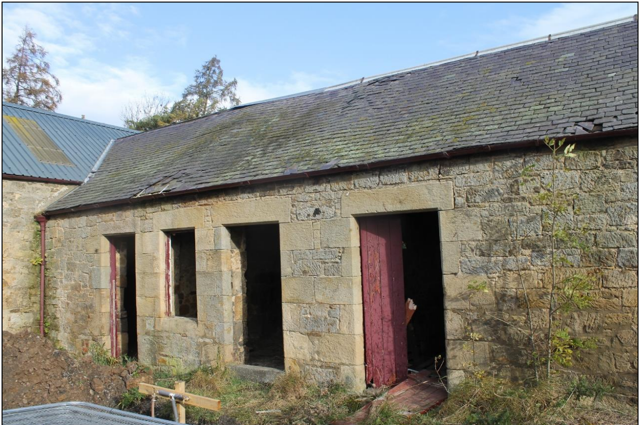
Figure 13a: Building L; west elevation
