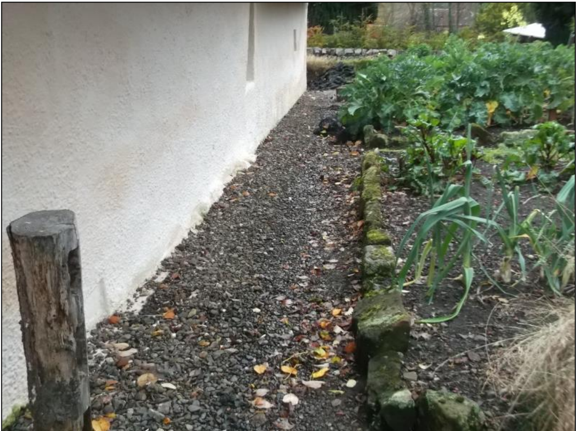
Figure 2b: Pre-excitation shot of walkway/soil beds along northwest side of cottage from the northeast, where pipe trench located
