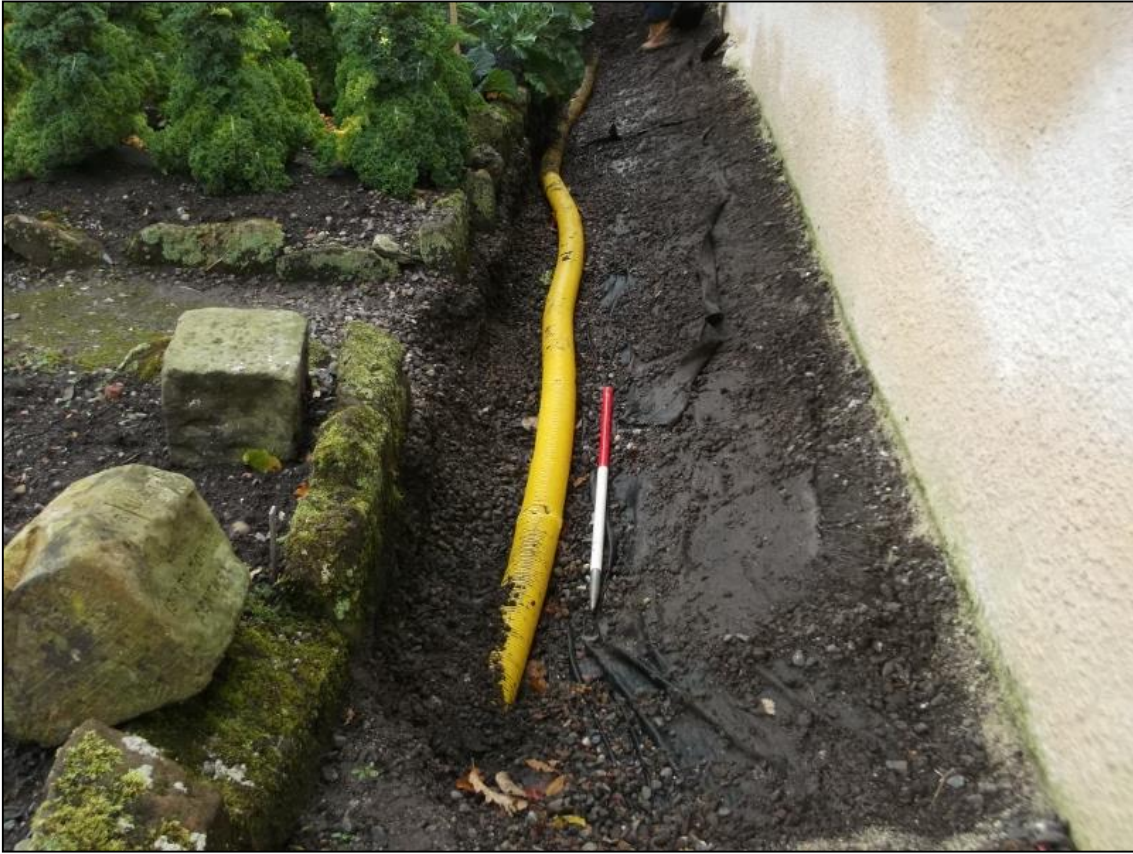
Figure 3a: Drain [004] from the southwest
