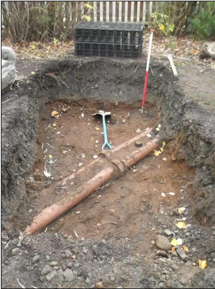
Figure 5a: Trench for northeast soakaway from the west-north-west showing ducts [011]
