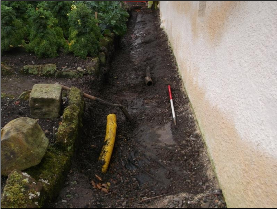
Figure 4a: General shot of pipe trench from the southwest
