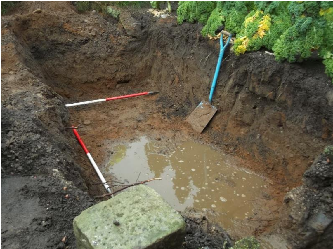
Figure 5b: Trench for southwest soakaway from the south
