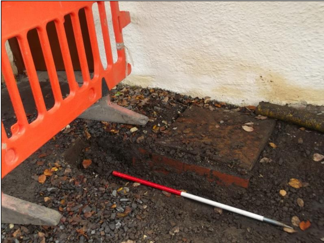
Figure 4b: Manhole [005] from the northwest
