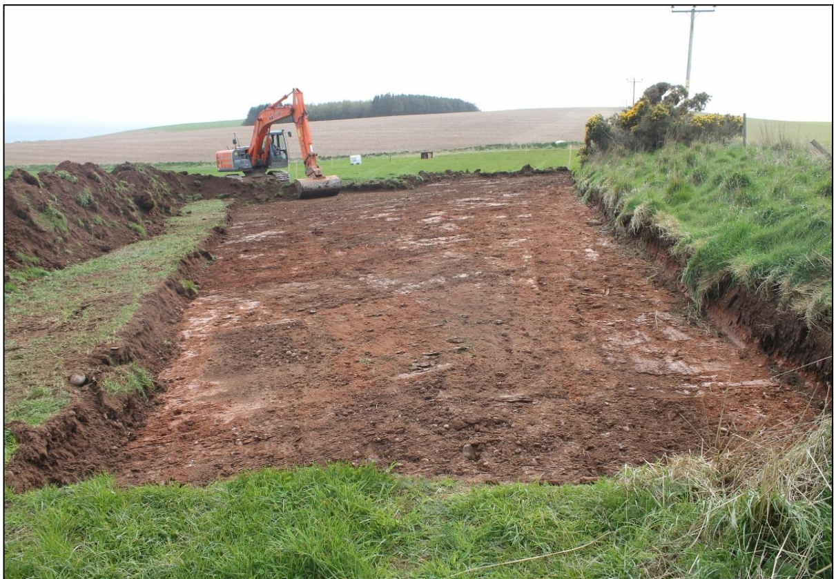
Figure 2b: Northern edge of turbine storage and crane pad area.
