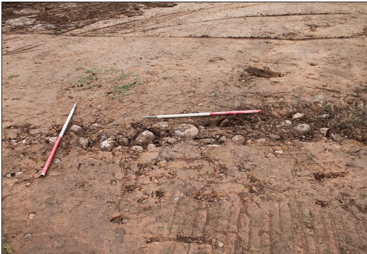
Figure 5b: Feature (003, rubble field drain in located in the north-western area of the turbine area. Showing the last 2-2.5m.
