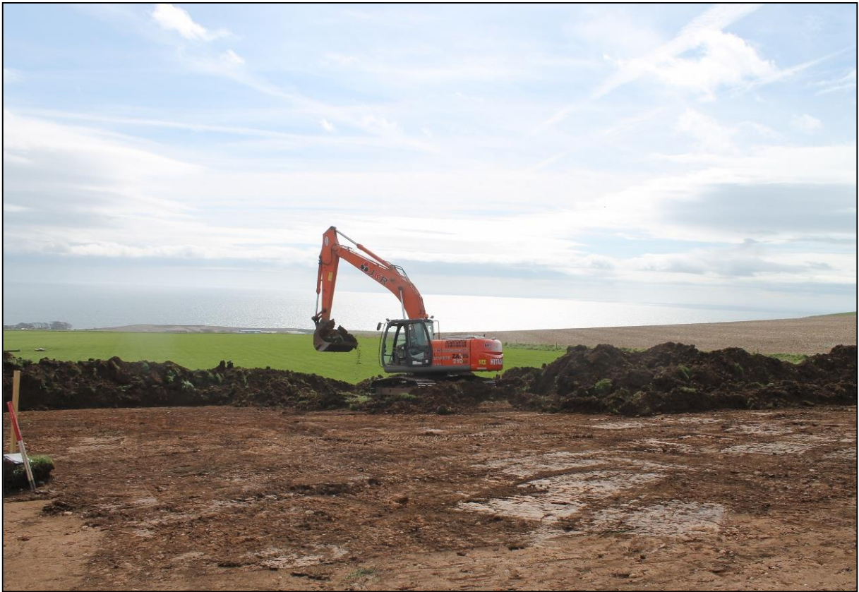
Figure 3a: Excavating turbine storage and crane pad area.
