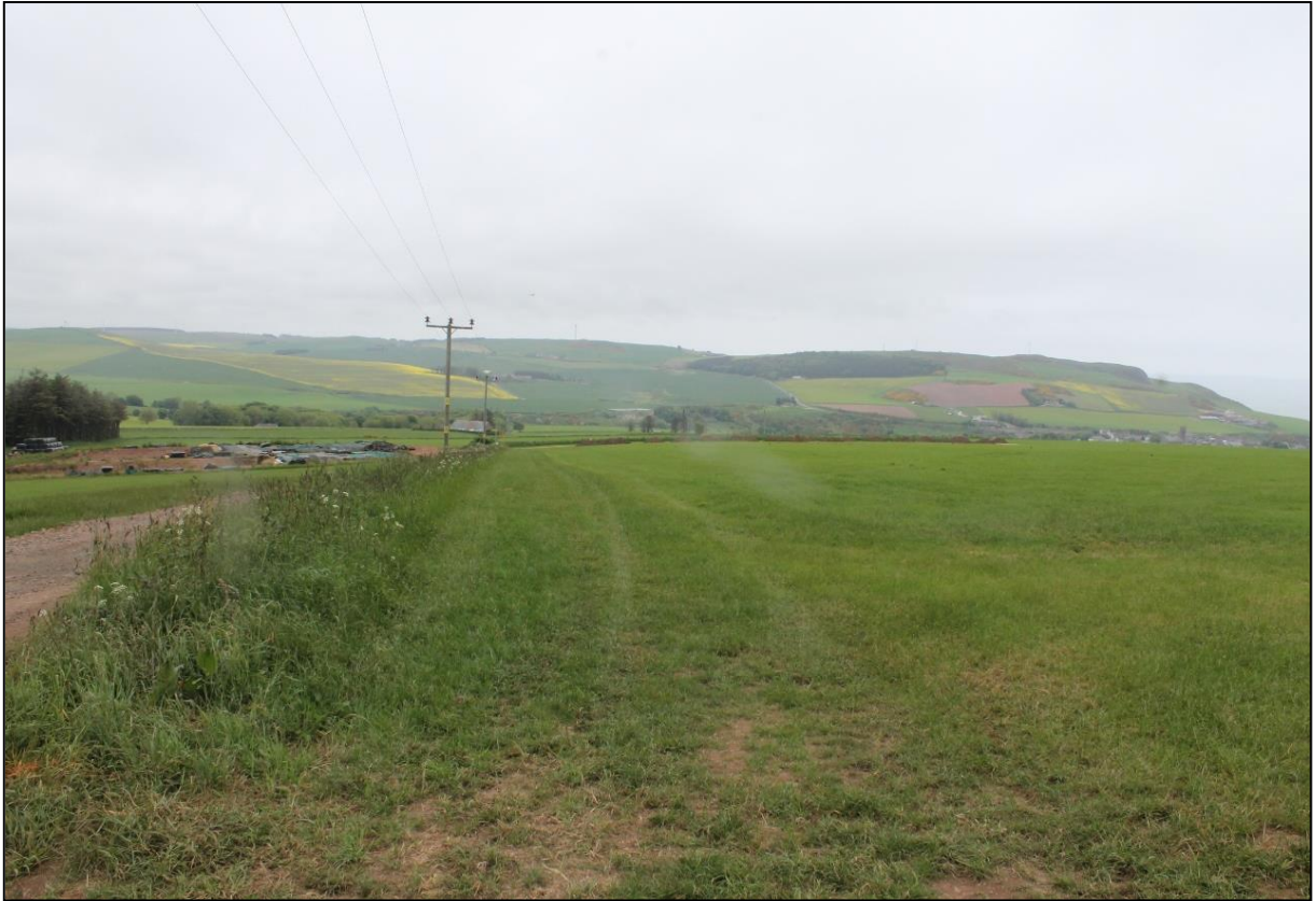
Figure 10a: Post excavation of the upper southern section of the 11kv cable trench.
