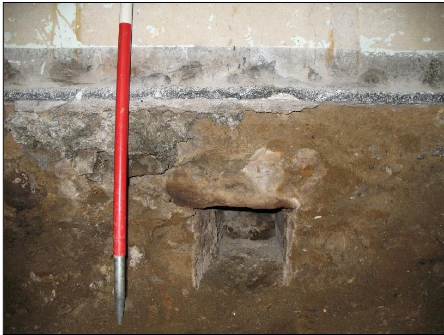
Figure 6a: In situ boulder course at base of S wall, Room 023
