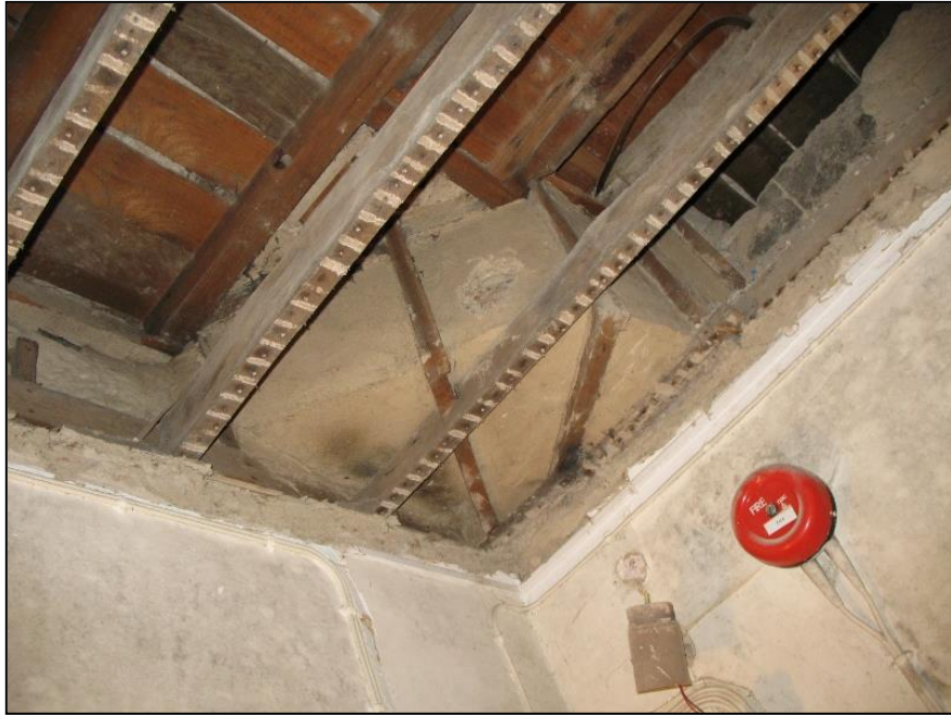
Figure 17a: Stone plinth for fireplace in SW corner of Room 221, viewed from below
