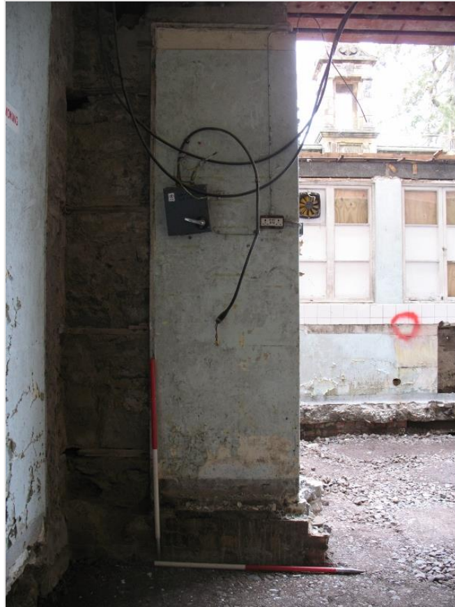
Figure 8a: Line of earlier E-W walling originally forming external N wall of house
