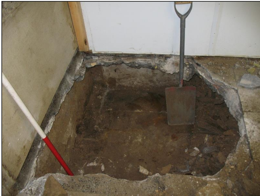
Figure 9b: Sandstone flagged floor revealed beneath modern terrazzo layer, Room 033
