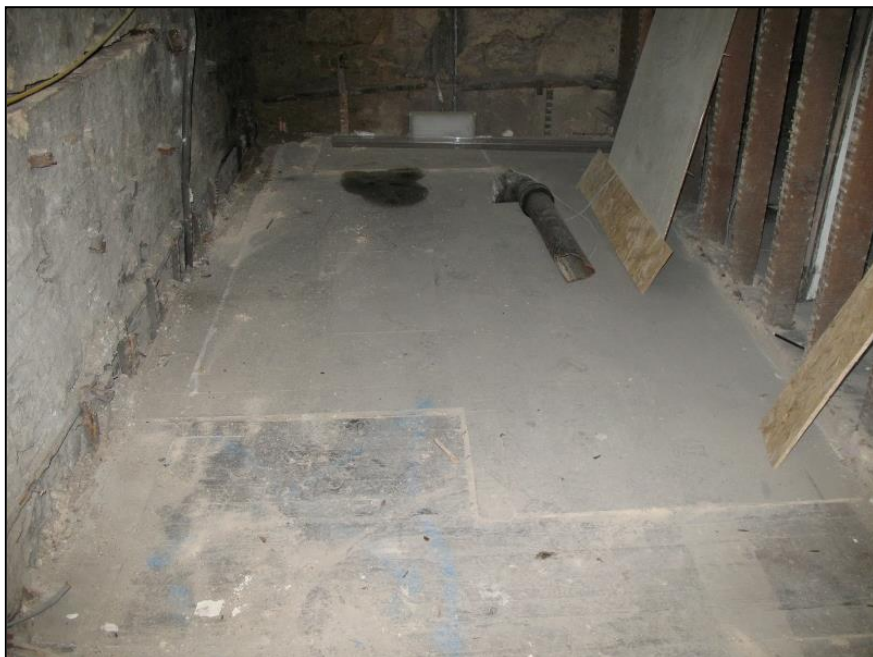
Figure 19b: Inserted floor over site of stair in S end, Room 308
