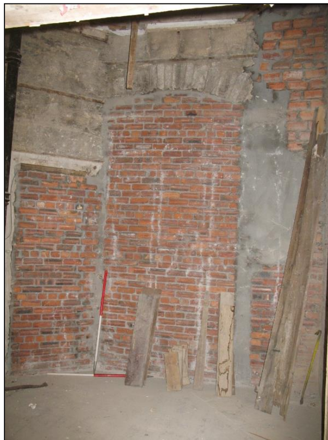
Figure 11b: Room 106 – View of W wall, seen from NE corner
