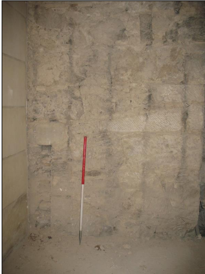
Figure 12a: Relict Fireplace in E wall, Room 114
