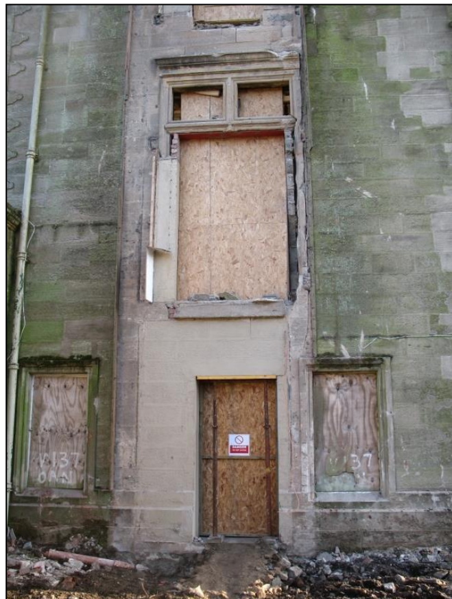
Figure 2b: N Elevation – W Bay following removal of external stair
