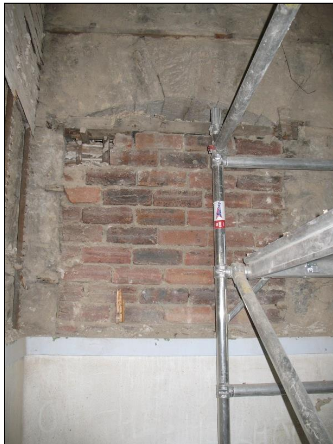
Figure 17a: Stone plinth for fireplace in SW corner of Room 221, viewed from below
