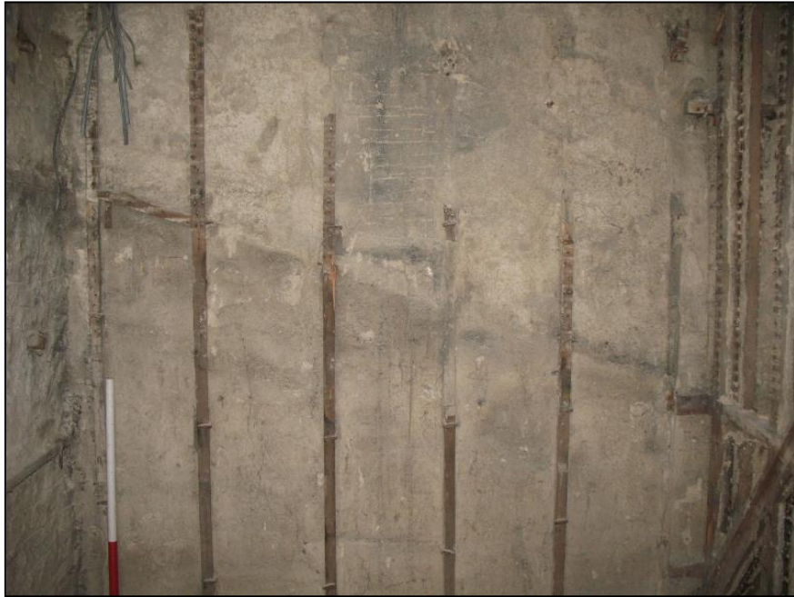
Figure 15a: W wall of Room 113, showing line of former stair
