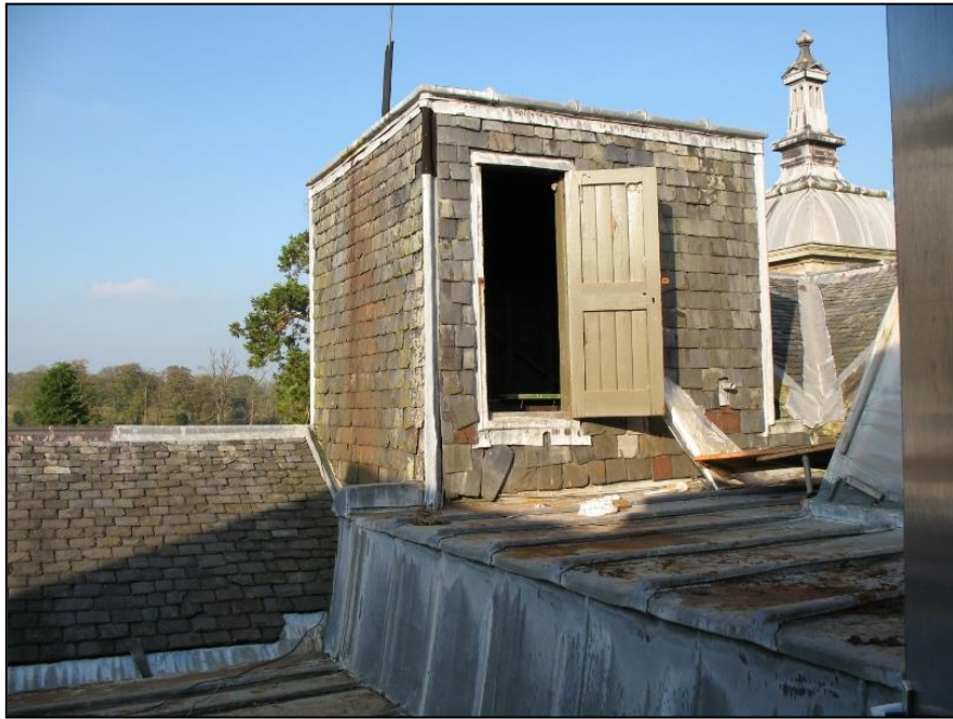
Figure 19a: Inserted caphouse projecting above original roofline
