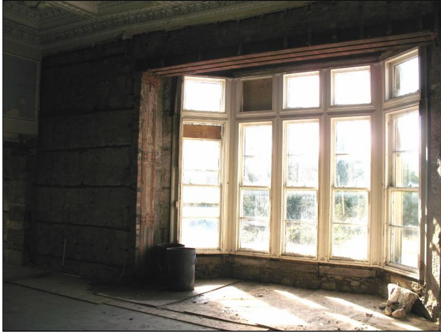
Figure 13a: 1930s reinforcement of bay window, Room 103
