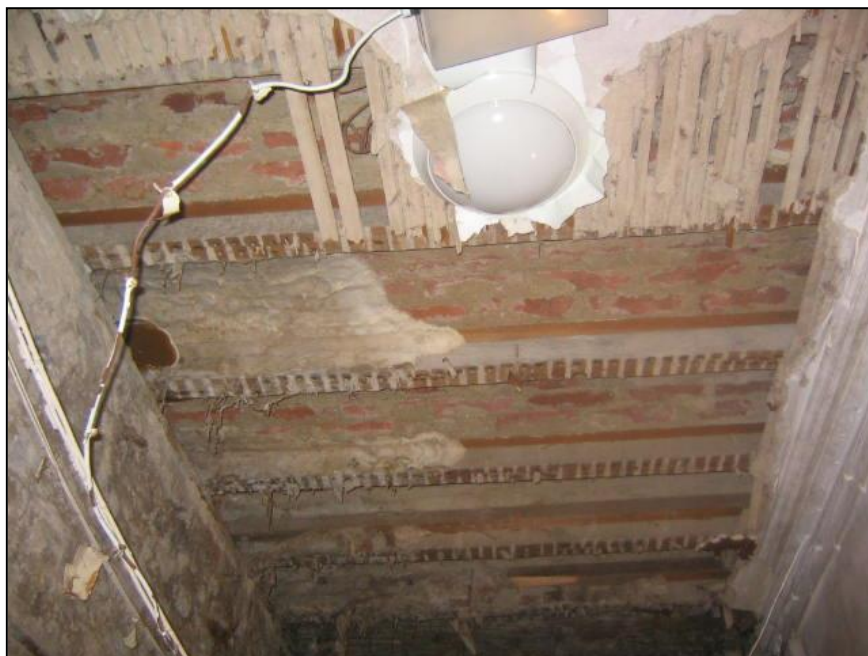
Figure 5a: External view of lift shaft, viewed from Room 014, showing hole punched through original masonry and then infilled with brick following insertion of lift
