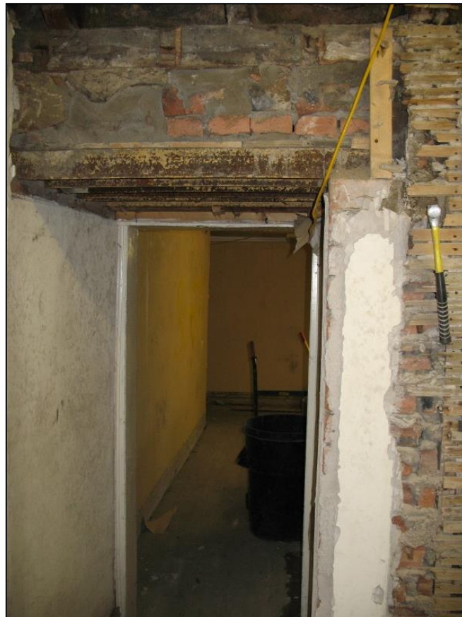
Figure 20b: Inserted doorway between modern Room 303 and Corridor 311
