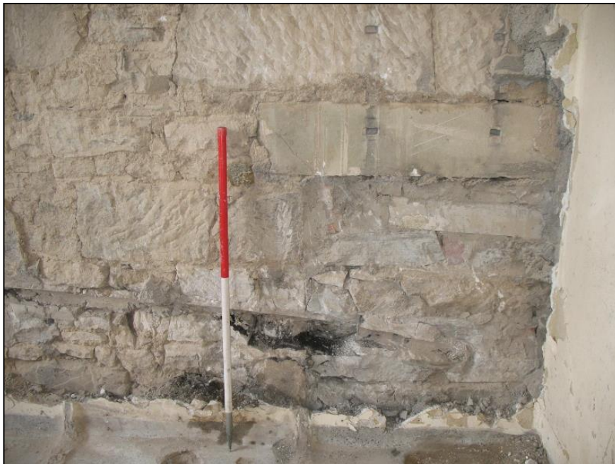
Figure 12b: Relieving arch at low level, S wall of Room 115
