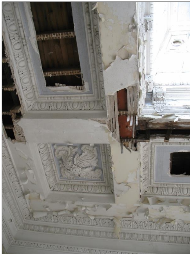
Figure 18a: Upper level of Atrium 201 – 1930s consolidation works revealed
