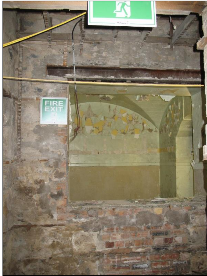
Figure 7a: Site of blocked doorway accessing Room 009 from Corridor 005 (N end)
