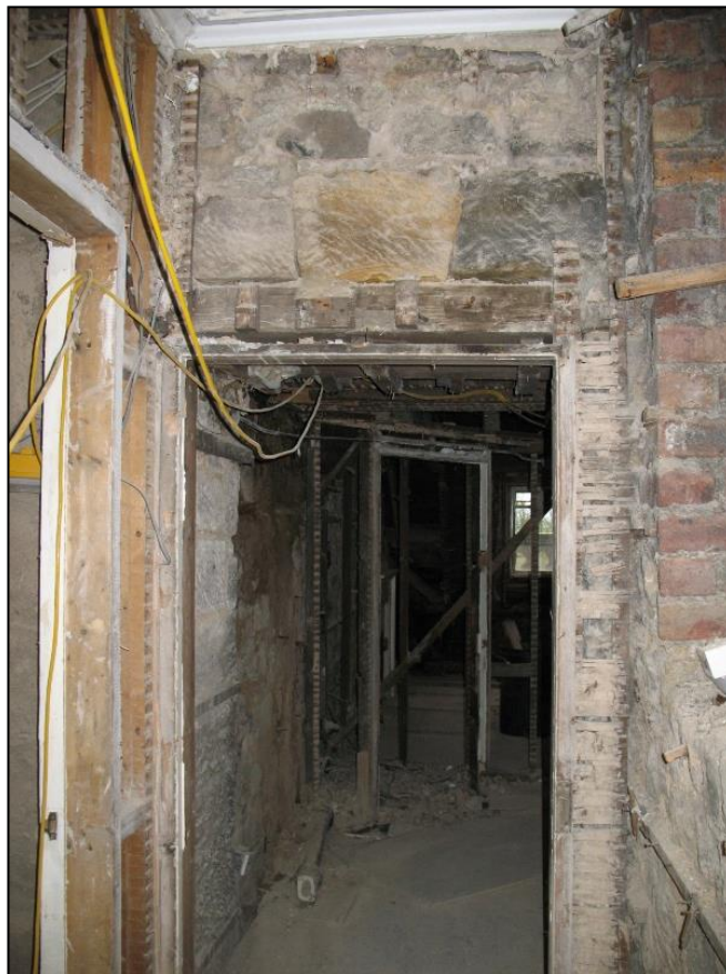
Figure 21b: Flat arch lintel, Corridor 304
