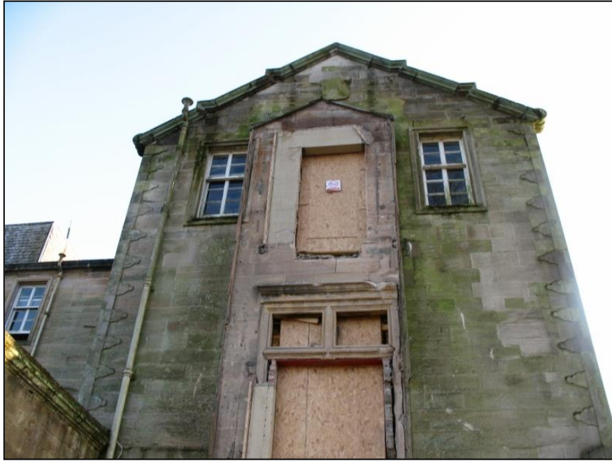
Figure 2a: N Elevation – W Bay following removal of External Stair (Upper)
