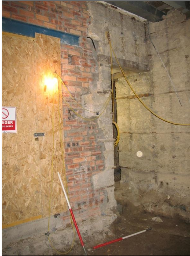
Figure 5a: External view of lift shaft, viewed from Room 014, showing hole punched through original masonry and then infilled with brick following insertion of lift
