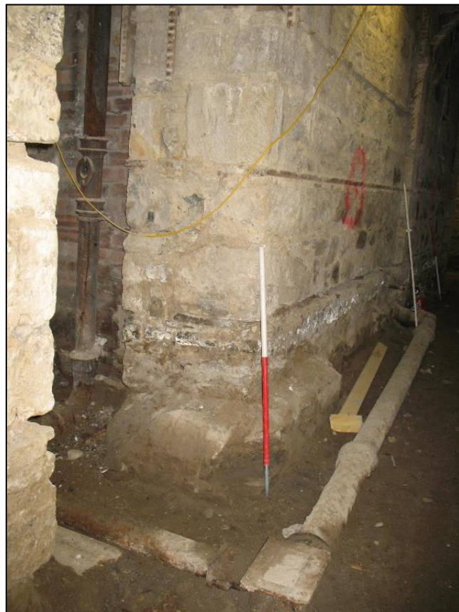
Figure 22b: Cast iron drainage pipe revealed during ground reduction in Corridor 008
