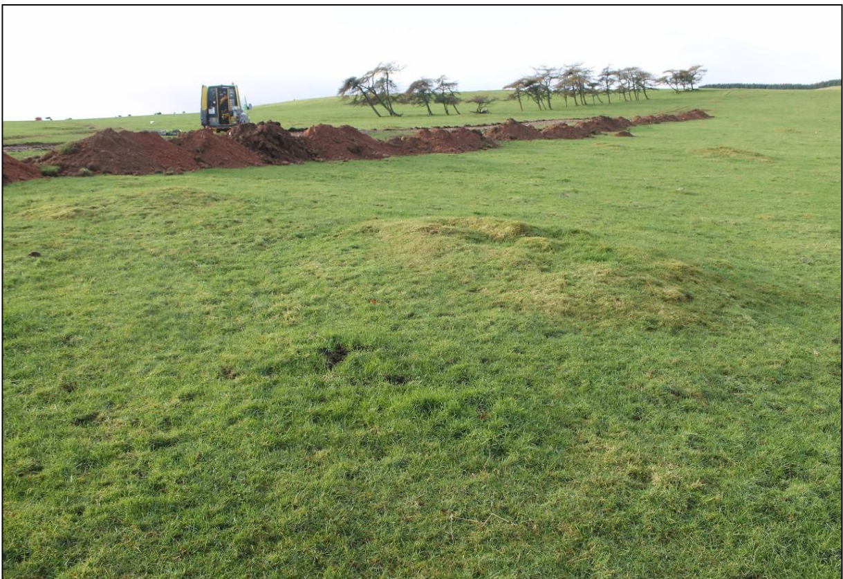
Figure 5b: Demonstrating possible clearance cairn 3
