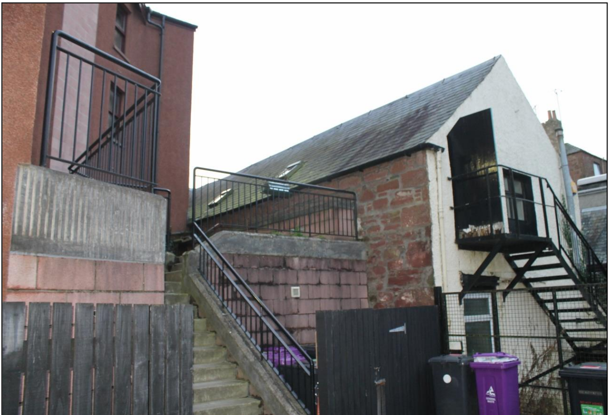
Figure 7b: Demonstrating the snecked red sandstone construction of the east elevation
