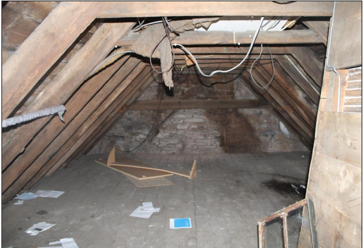
Figure 10a: East side of the Attic/Roof space
