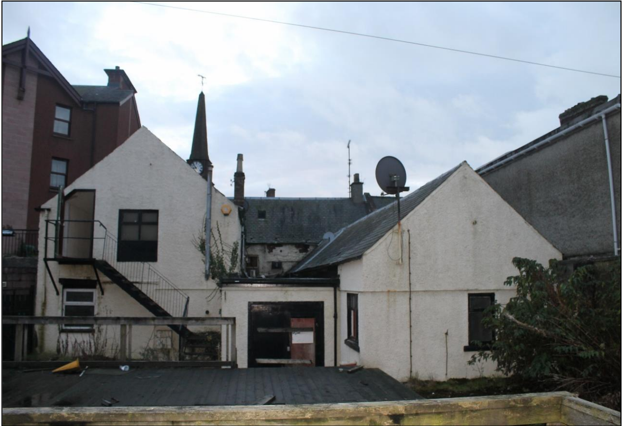
Figure 6a: North/Rear elevation and showing the modern central in-filling
