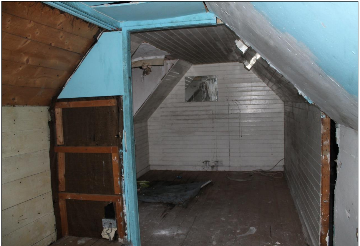
Figure 10b: West side of Attic/Roof space
