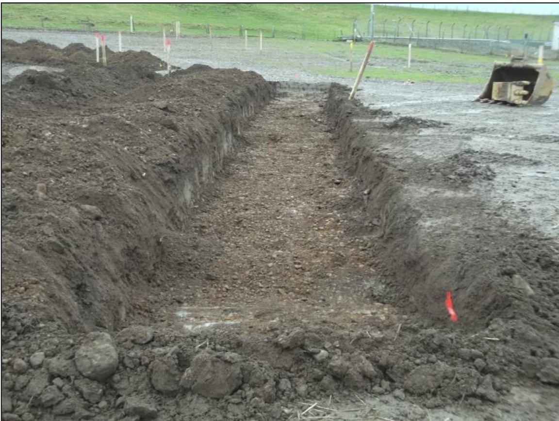
Figure 5: Trench 3 from the north-northwest showing subsoil (002)
