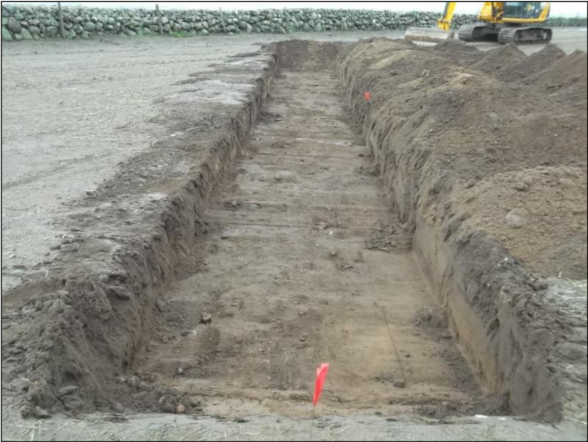
Figure 6: Trench 1 from the south-southeast showing subsoil (004)
