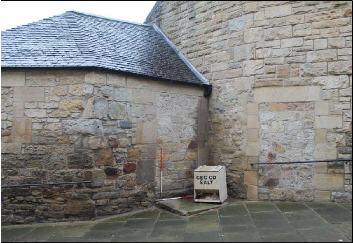
Figure 10a: Historic structural elements on the south elevation showing infilled doors.
