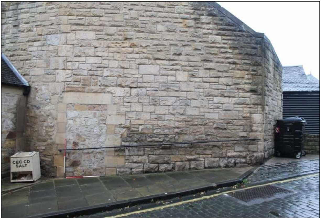
Figure 9b: Historic structural elements on the south elevation showing infilled doors.
