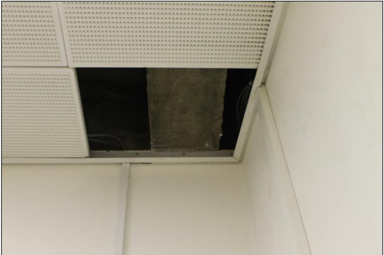
Figure 8a: Showing the modern concrete structural beam.
