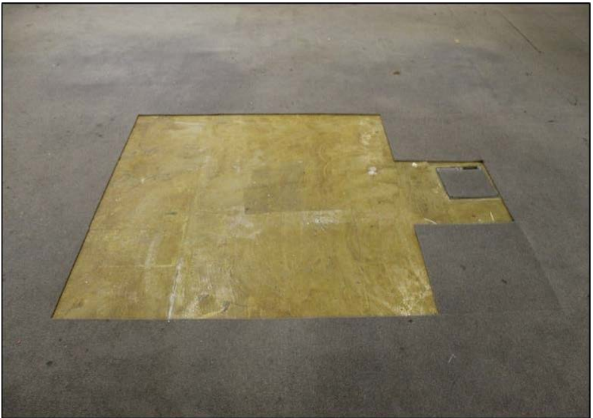
Figure 8b: Showing concrete flooring.
