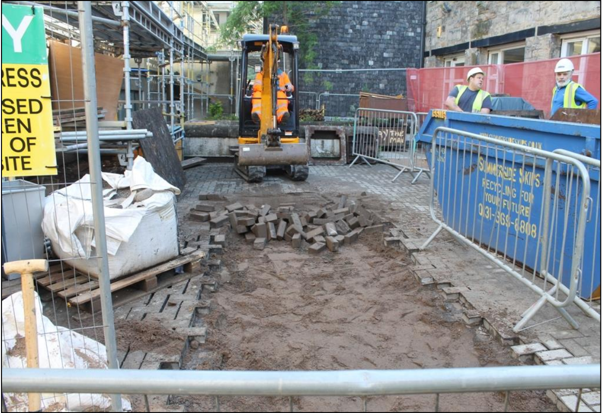
Figure 18a: Courtyard Trench
