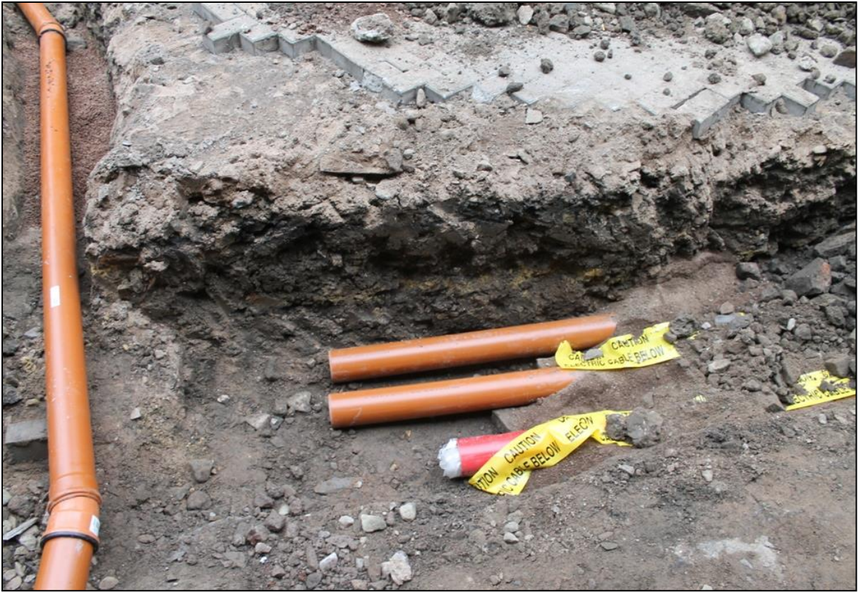
Figure 16a: Garage Block Trench context (010)
