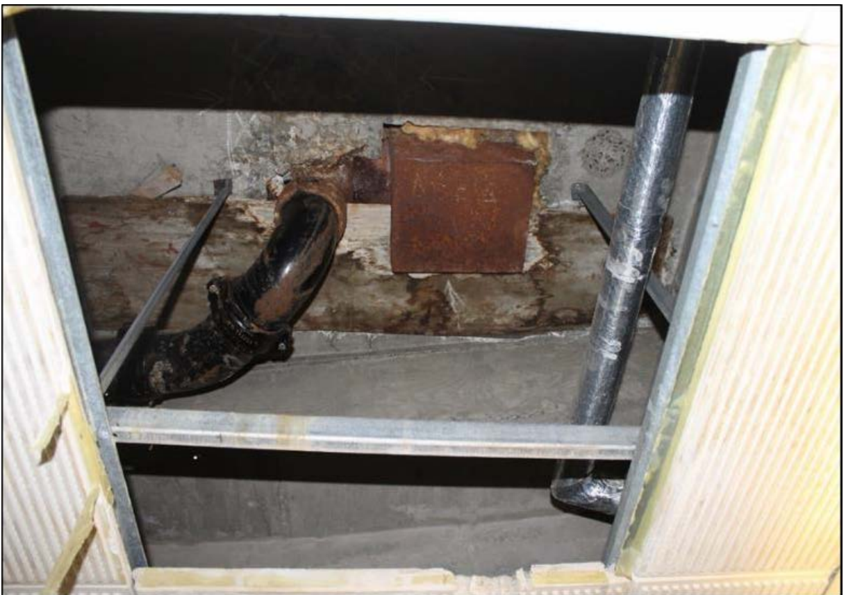
Figure 7b: Showing the modern concrete ceiling.
