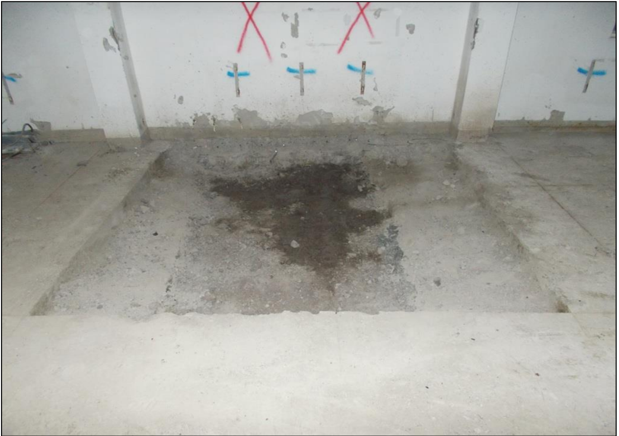
Figure 15a: Internal Test Pit 4.
