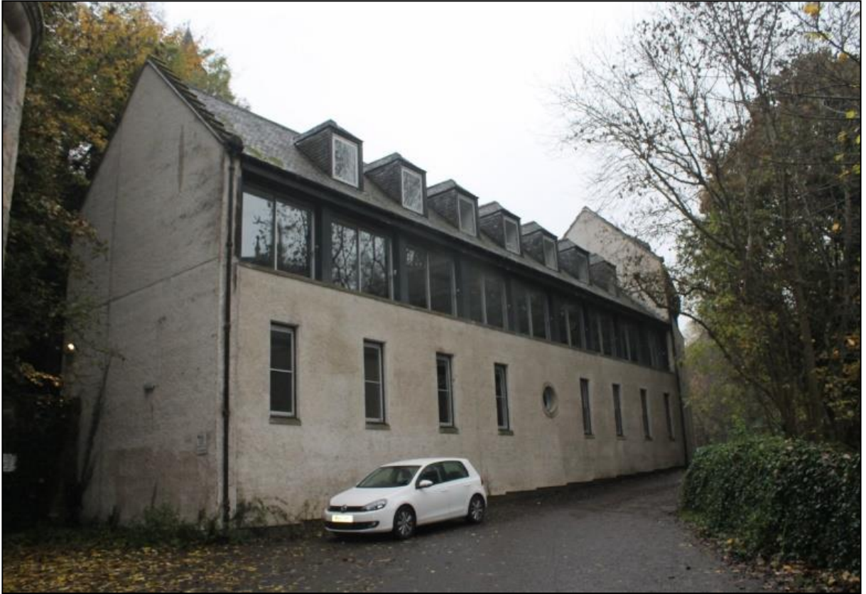
Figure 4a: East end of No.10 Bell's Brae, note brick basal courses under render.
