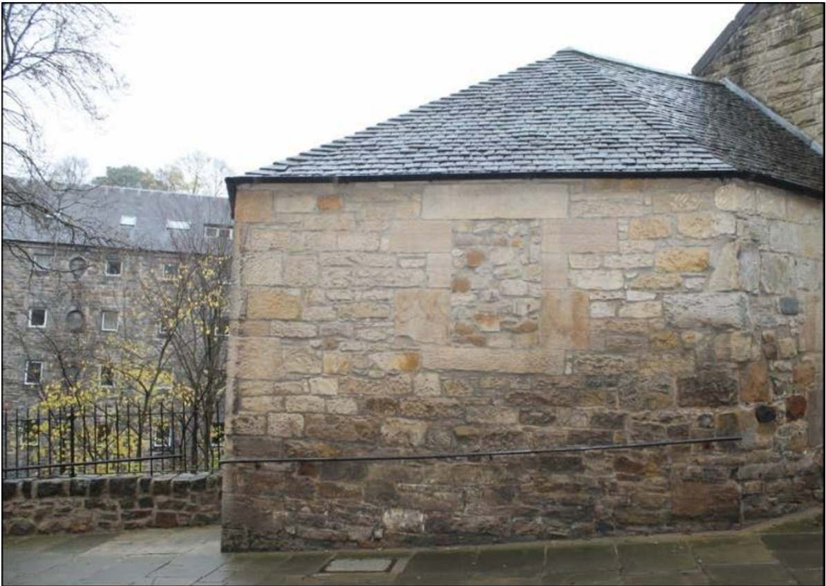
Figure 10b: Historic structural element on the southwest corner showing infilled window.
