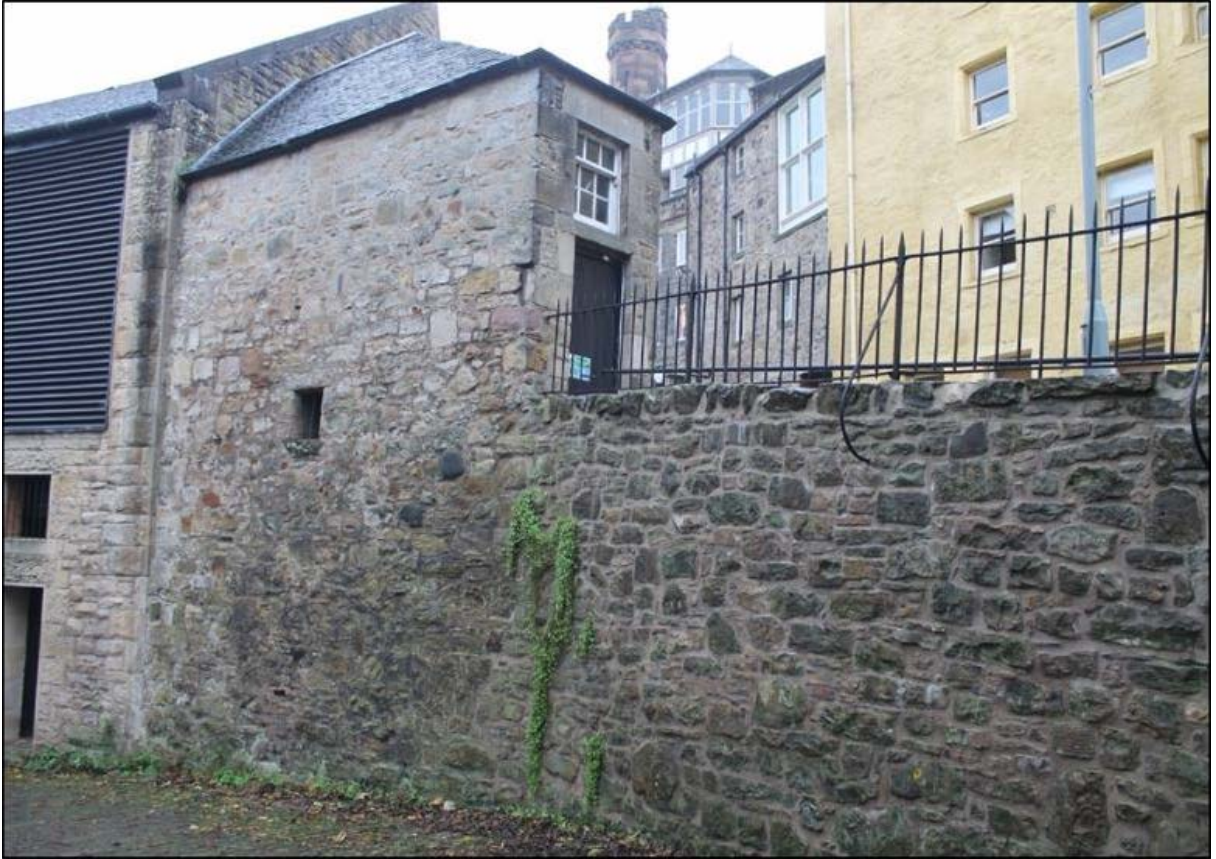
Figure 11a: Historic structural element on the southwest corner of garage/office building.
