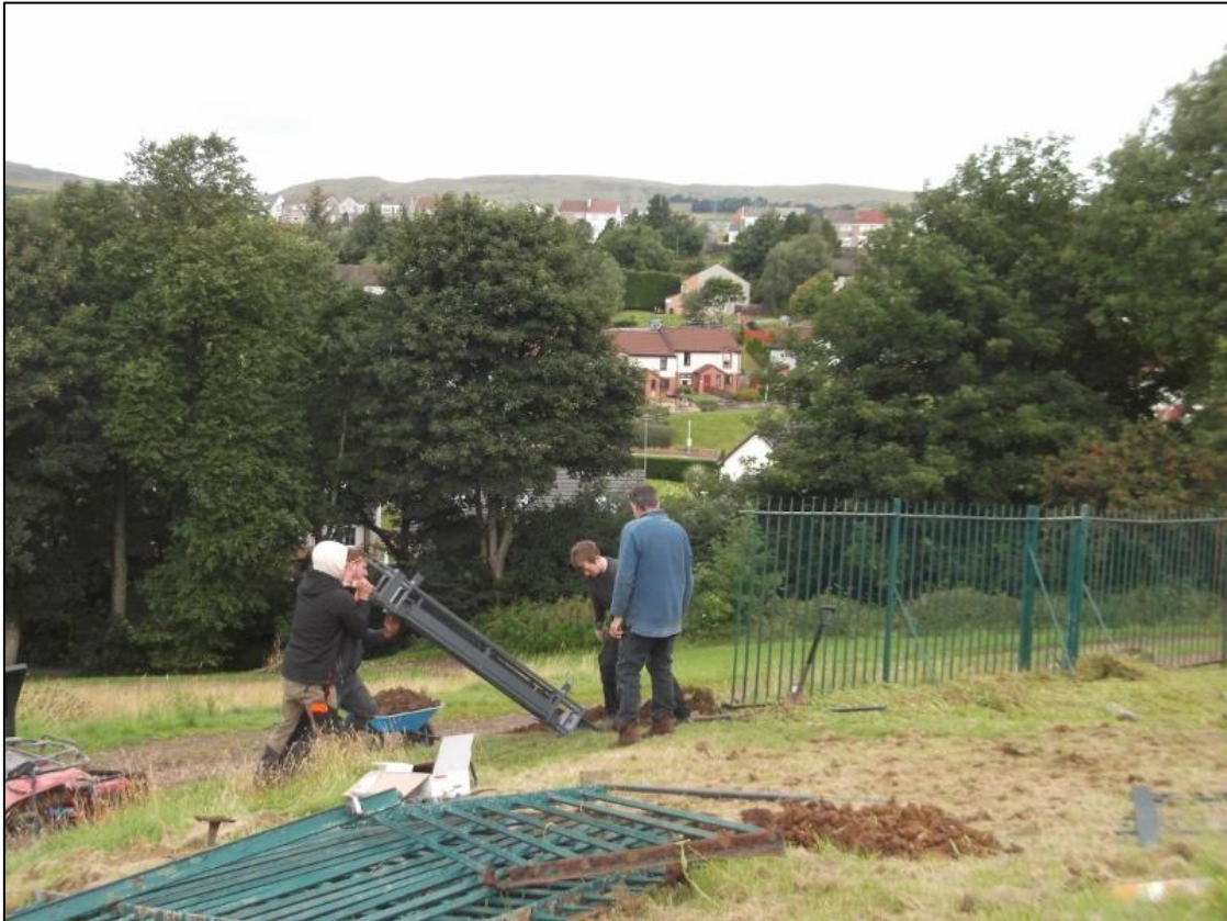
Figure 2a: View of new enclosure fence being erected. From SSE.
