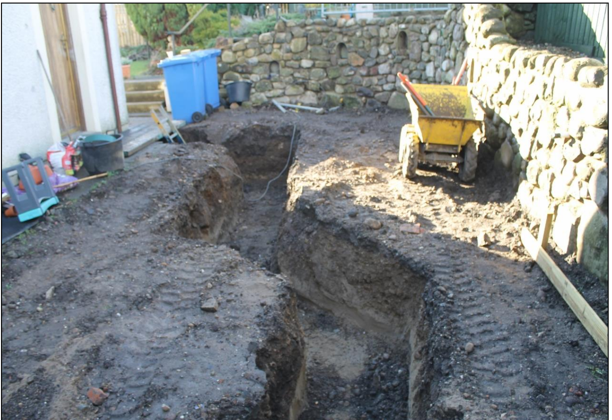
Figure 4b: Looking west along foundation trench
