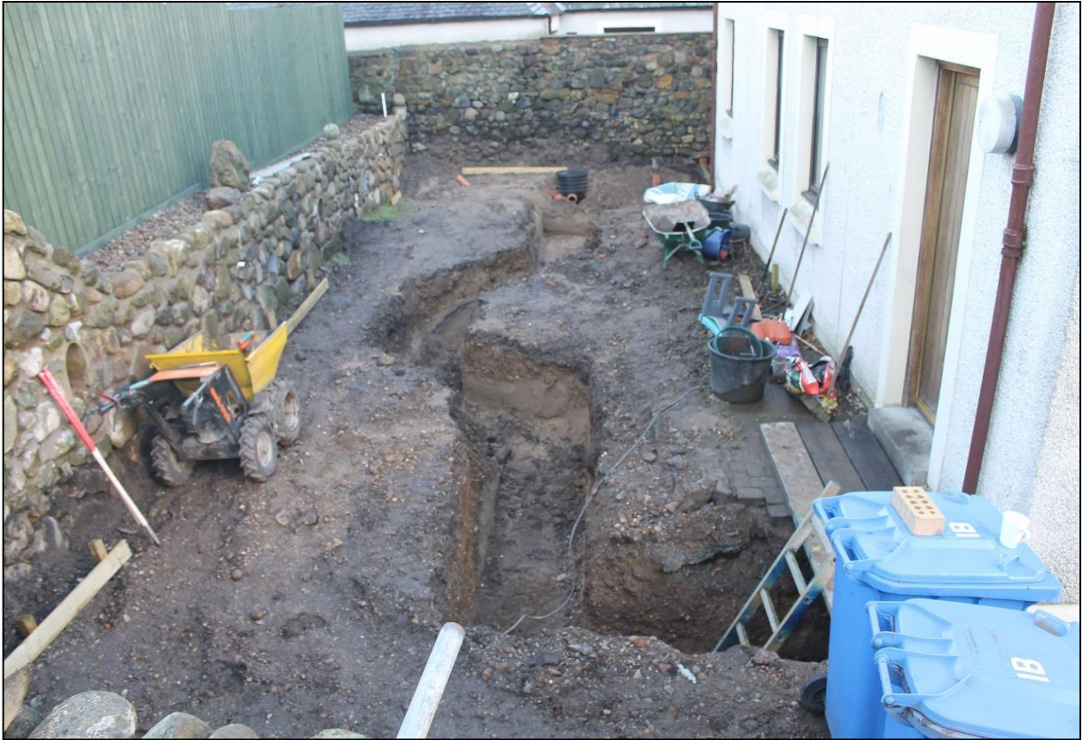
Figure 4a: Looking east along foundation trench
