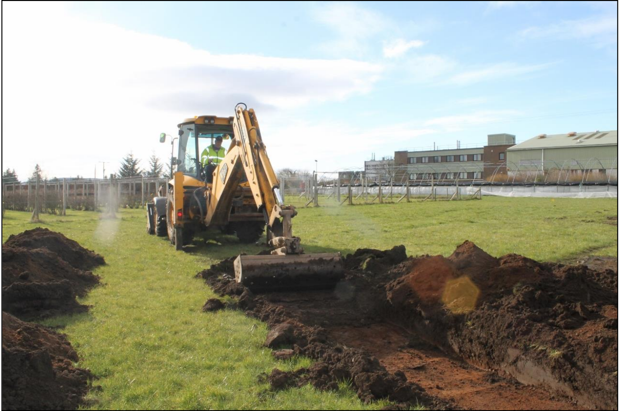
Figure 4a: A JCB 3cx was used to excavate the trenches
