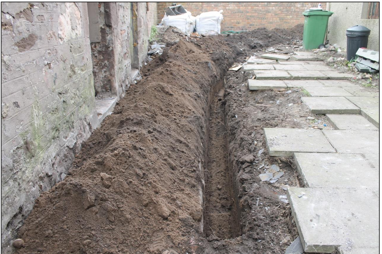
Figure 6b: Service trench excavated
