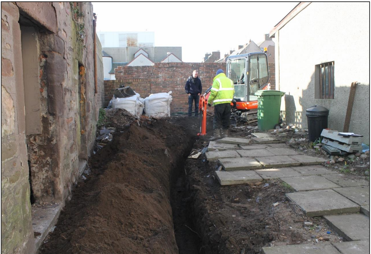
Figure 4b: Excavation for the service trench
