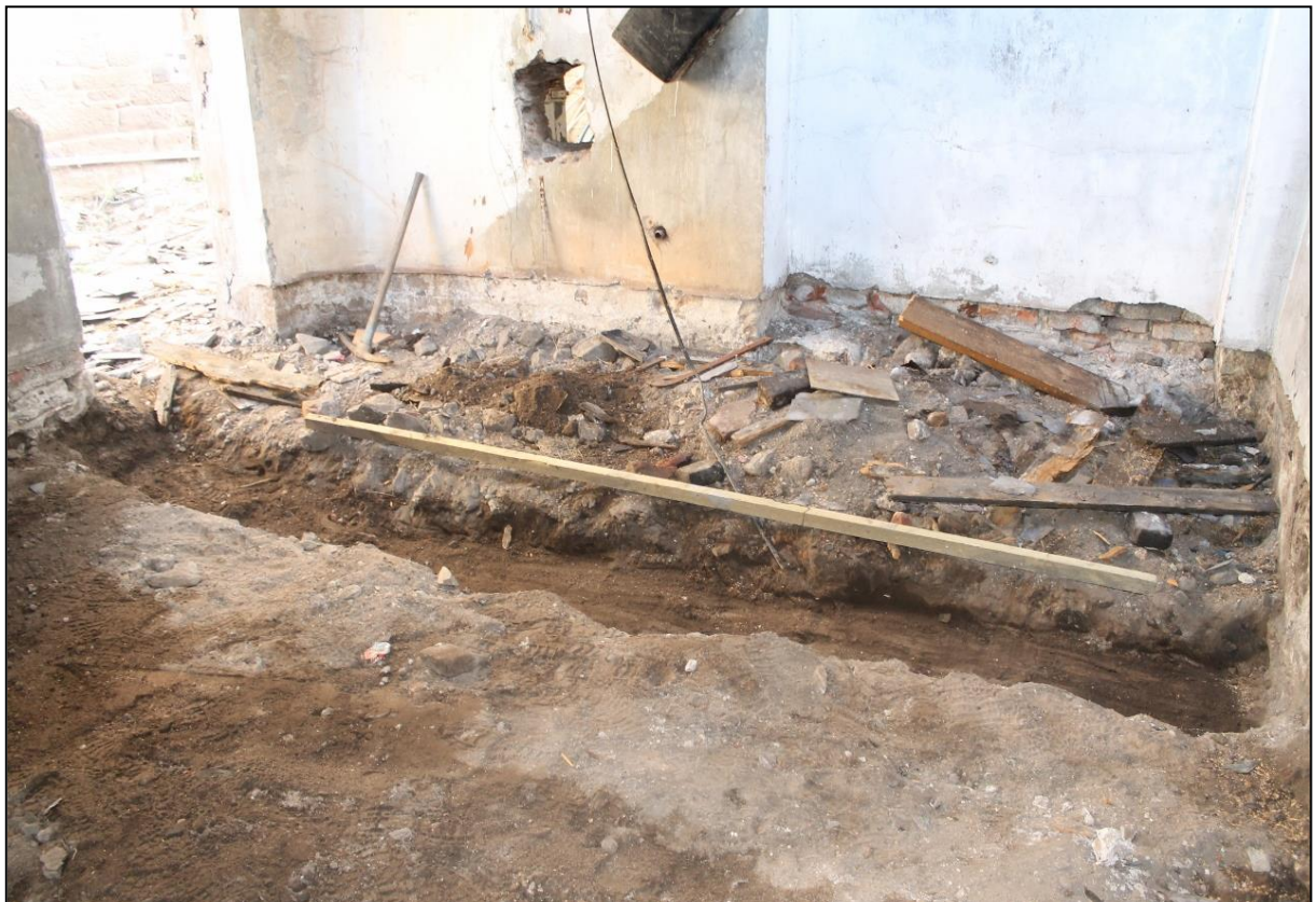
Figure 5b: Service trench at the east end of the redundant store
