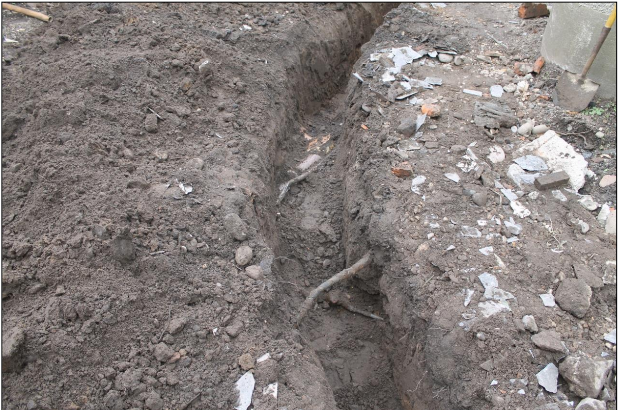
Figure 7b: Demonstrating disturbance from previously laid services
