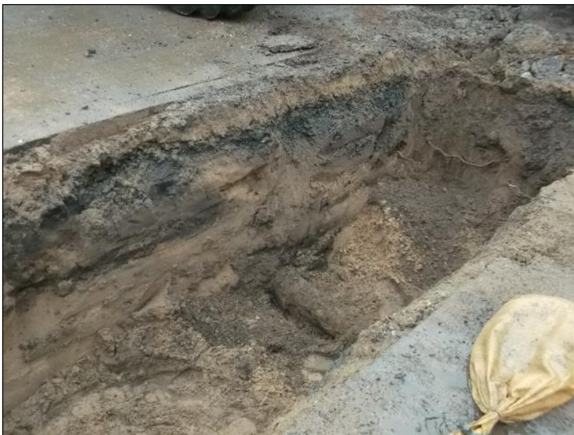
Figure 1b: ESE facing section of trench showing water mains pipe [5011] / (5012)
