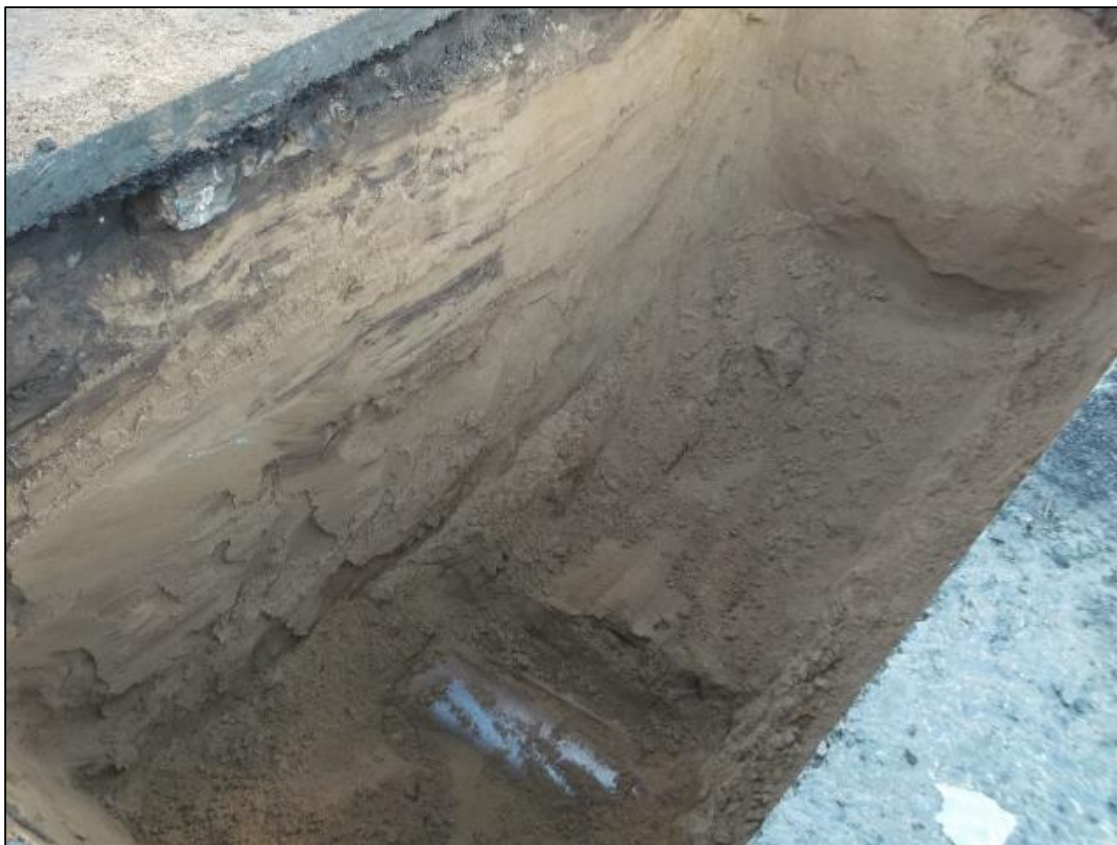
Figure 1a: ESE facing section of trench showing sewage pipe [5005] / (5006)
