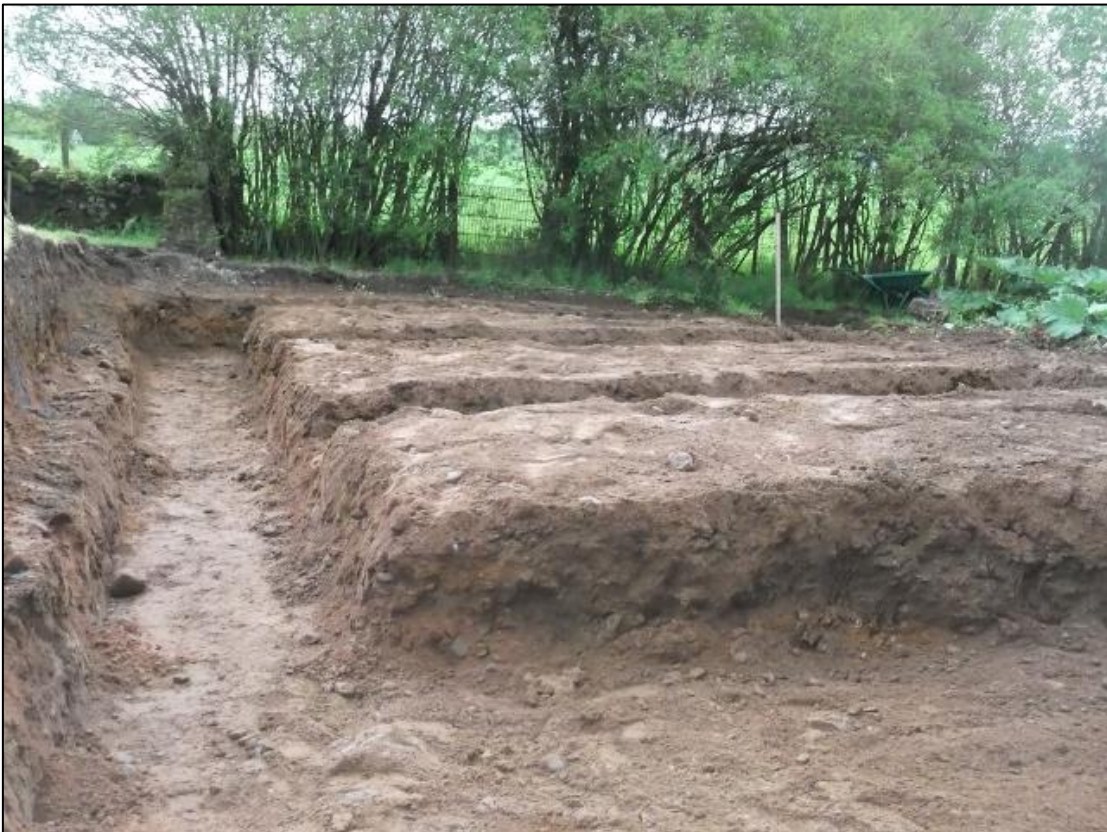
Figure 4b: View of the developments foundations fully excavated. Facing N.
