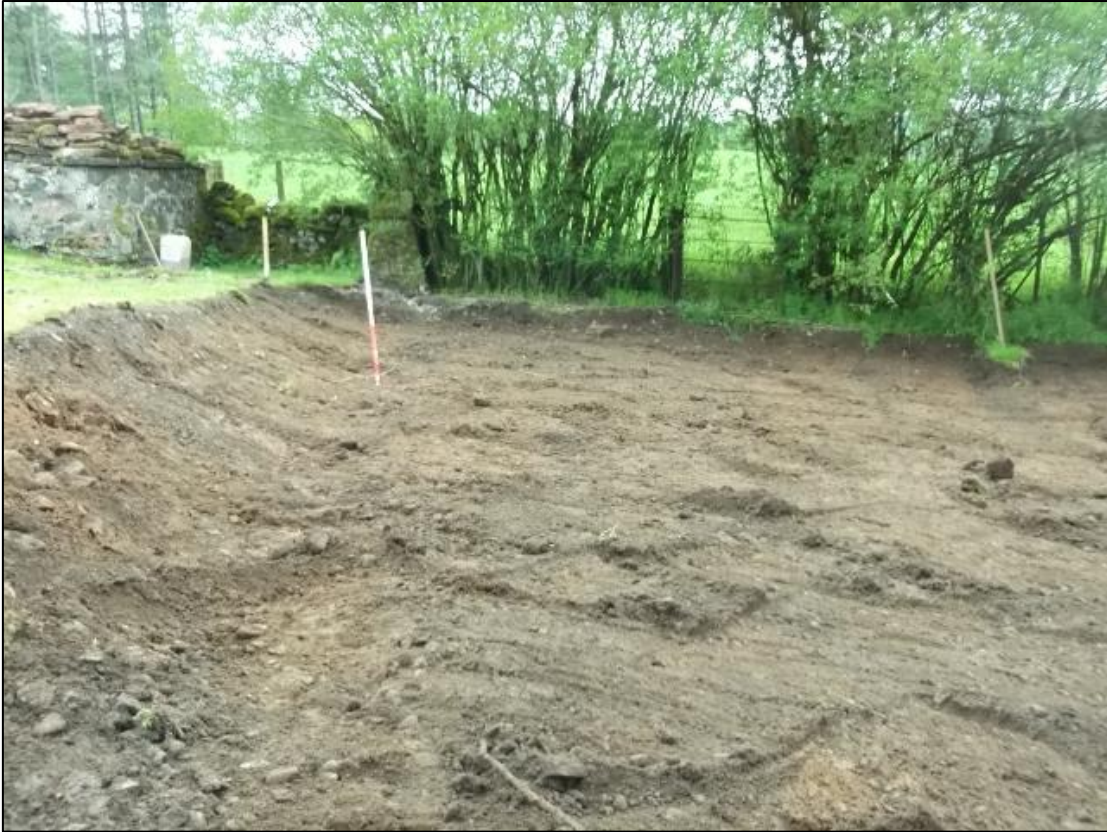
Figure 4a: Post excavation view of development area. Facing N.
