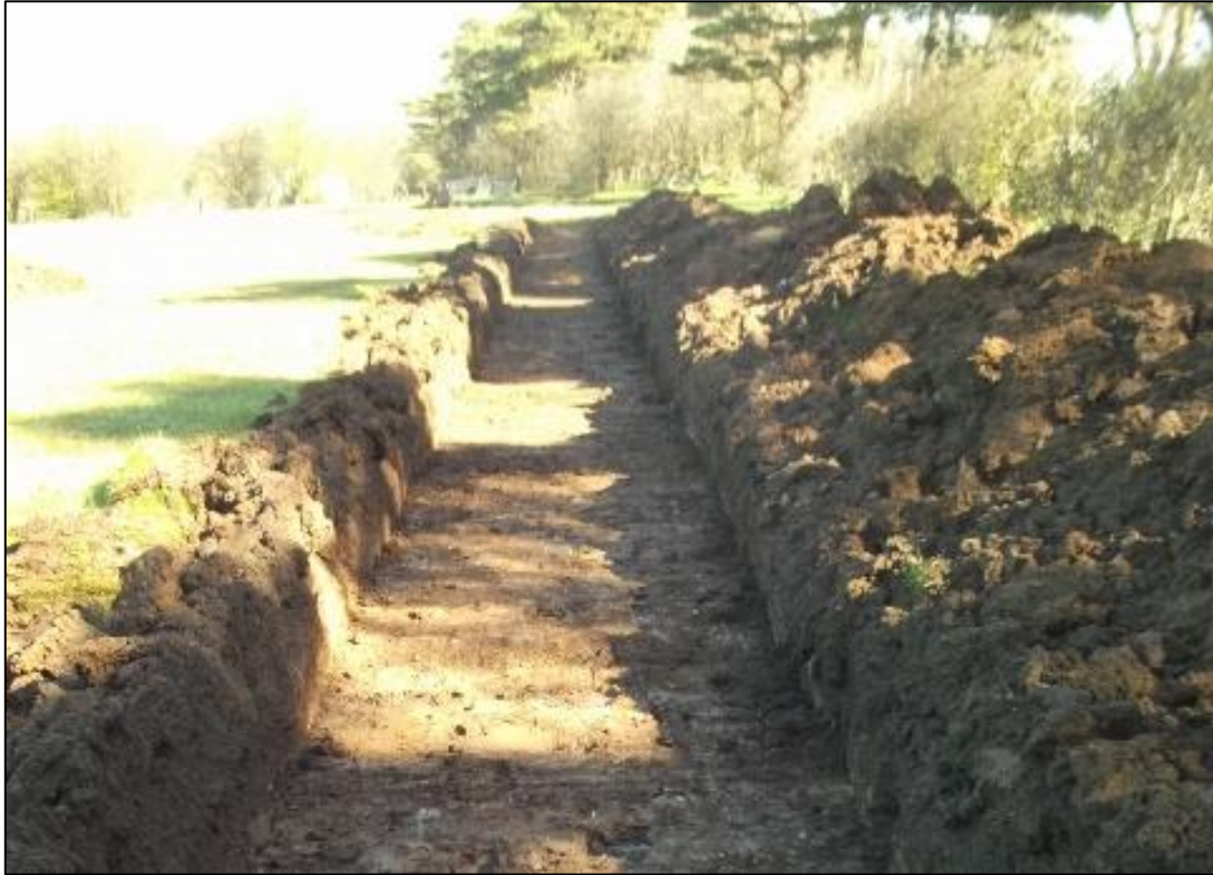
Figure 4a: View of Trench 13 from the S.
