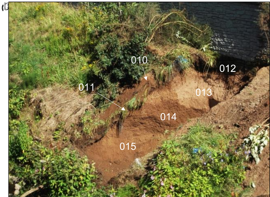
Figure 3b: Post excavation view of Outfall Trench, showing context numbers. From WSW
