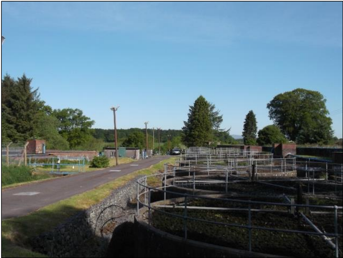
Figure 4a: View of the grounds & facilities within the WWTW. From the SE.
