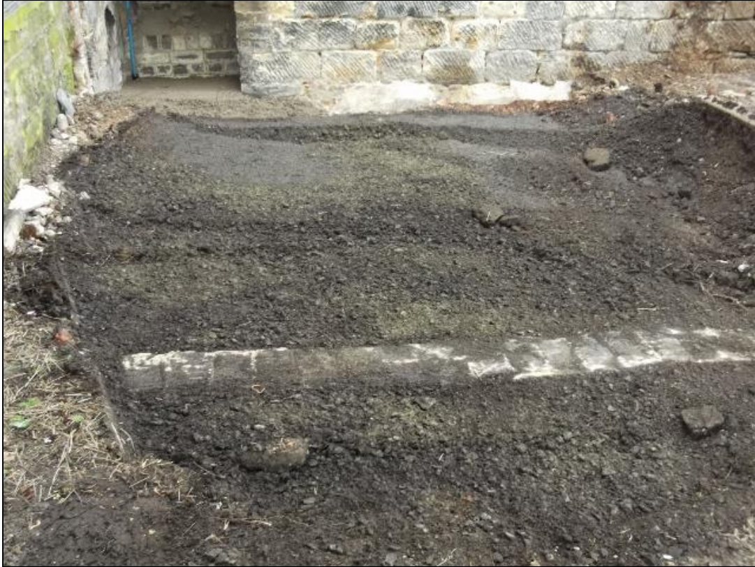
Figure 2a: View of wall (006) and backfill material (008) from the E.
