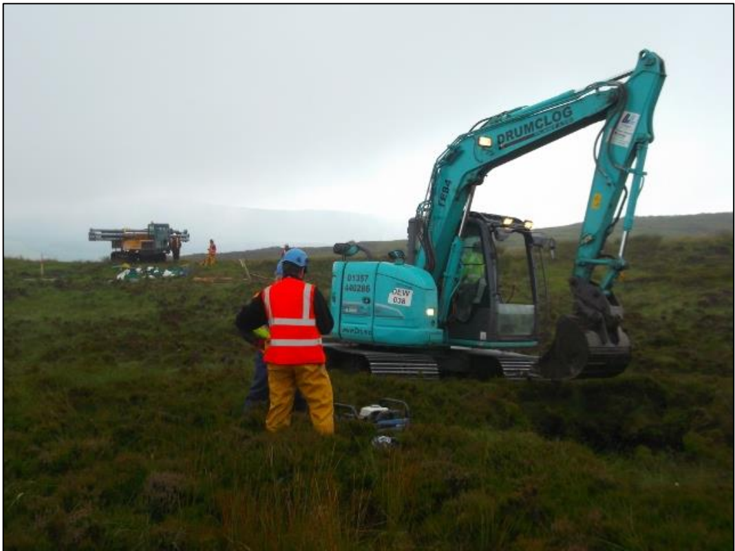
Figure 2b: Working shot of Trench 1 being excavated. From NNE
