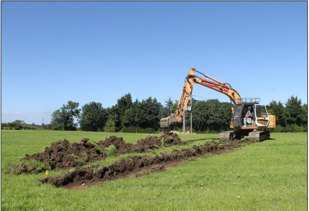
Figure 3a: A CASE 9013 was used to excavate the trenches
