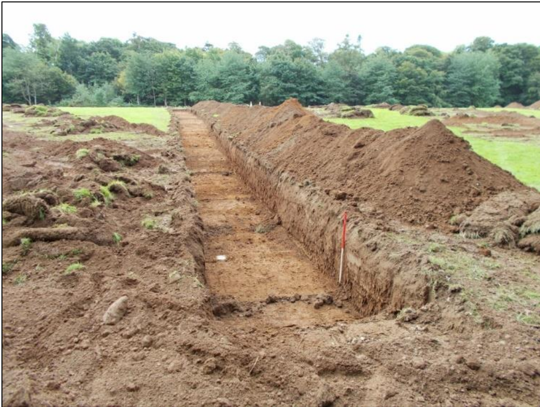
Figure 7b: Oblique view of Trench 5 from the SW.
