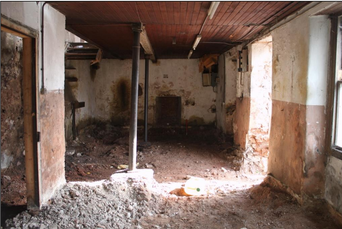
Figure 6b: View of Room 1, Ground Floor, 20a Swan St. From WSW
