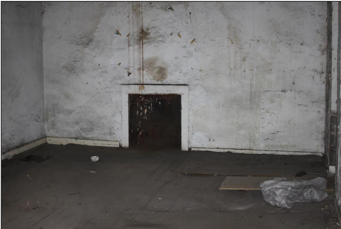
Figure 12b: View of Room 6, 1 st Floor, 20a Swan St. From WSW
