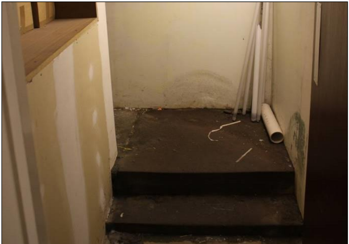
Figure 23b: View of stairs to Ground Floor, 20 Swan St. From E
