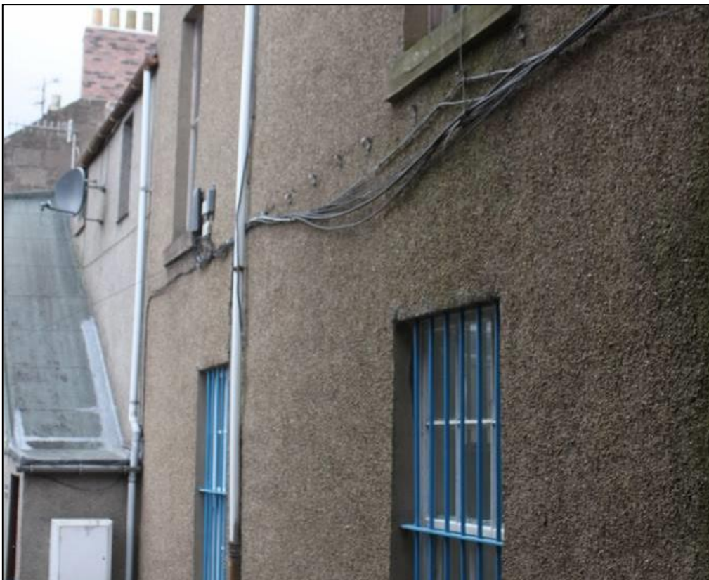
Figure 25b: Rear elevation of 14-18 Swan St. From the E
