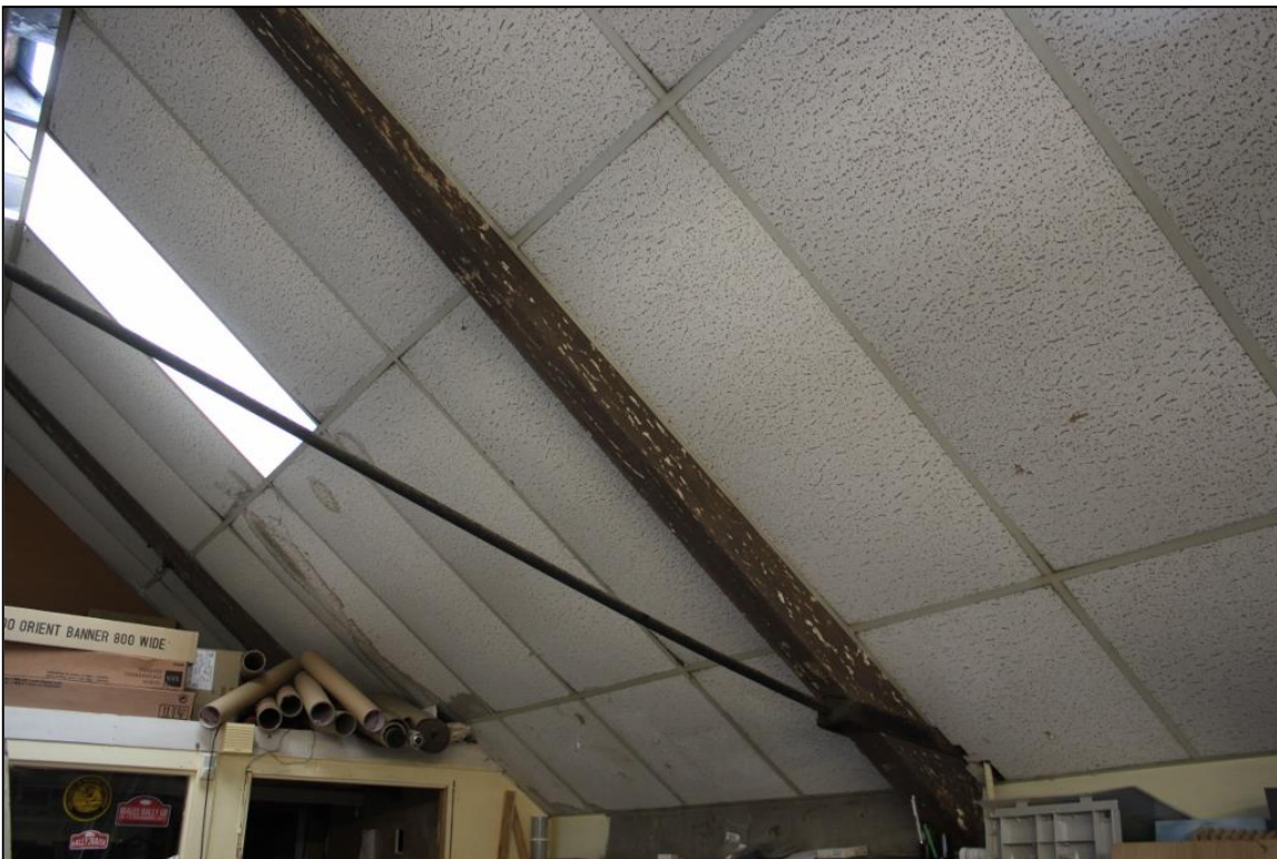
Figure 17b: Ceiling & roof beams, Room 1, 20 Swan St. From ENE
