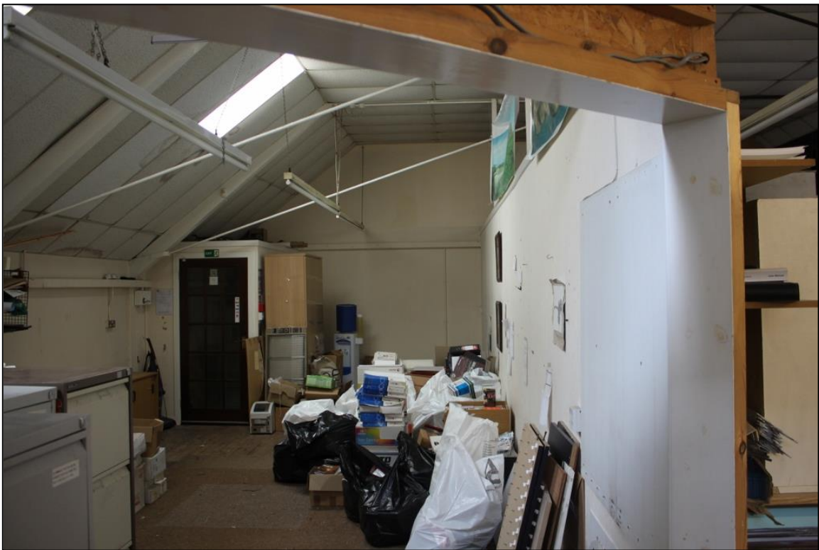
Figure 18b: View of Room 1, Ground Floor, 20 Swan St. From S
