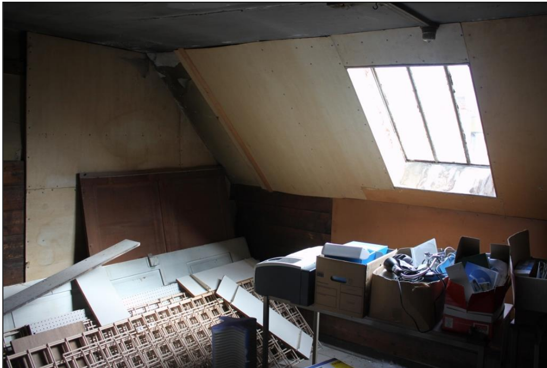
Figure 33b: View of Room 5, 2 nd Floor, 14-18 Swan St. From the WNW
