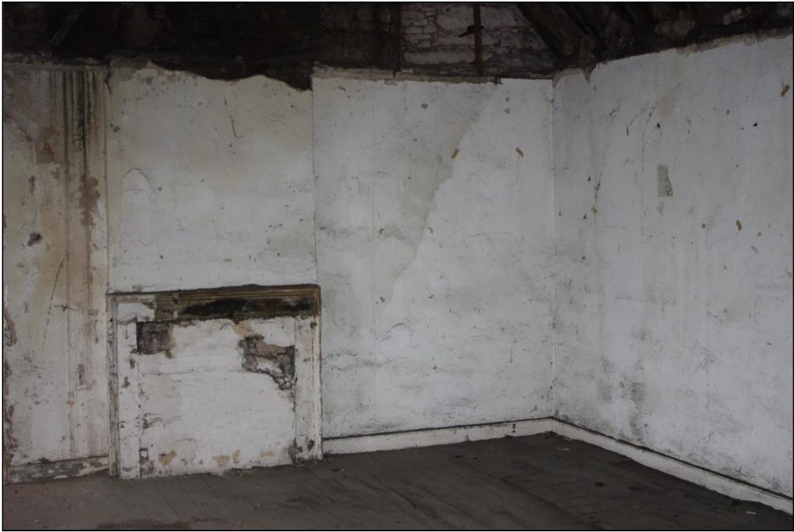
Figure 13a: View of Room 6, 1 st Floor, 20a Swan St. From ESE
