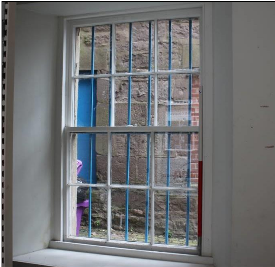
Figure 27a: Rear window, Room 1, Ground Floor, 14-18 Swan St. From the N
