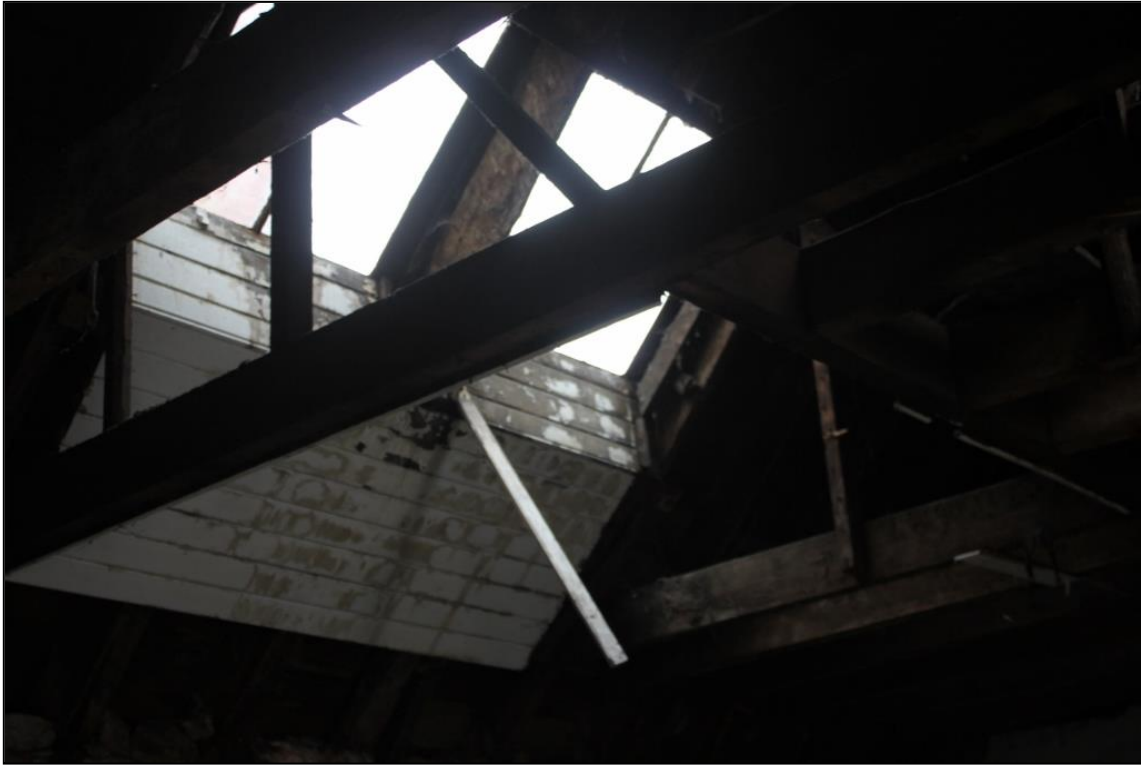
Figure 14a: View of Skylights within NNW ceiling of Room 6, 1 st Floor, 20a Swan St.
