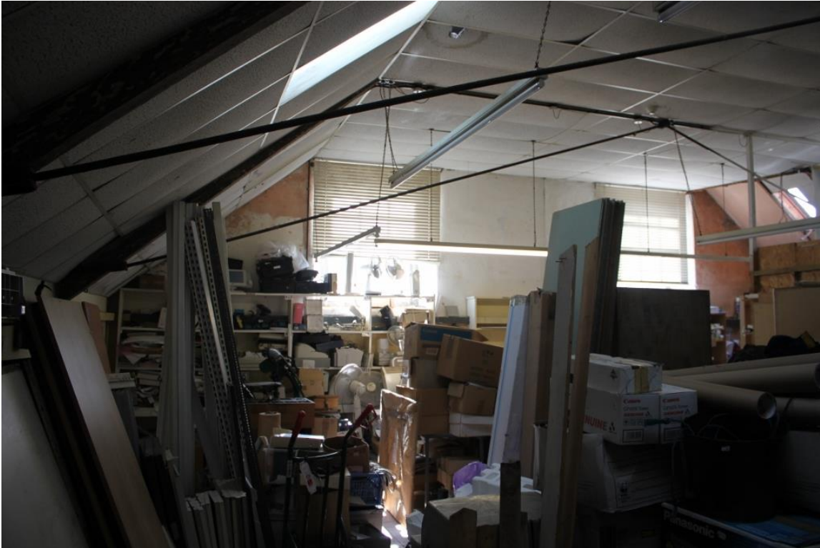
Figure 17a: View of Room 1, Ground Floor, 20 Swan St. From SSW
