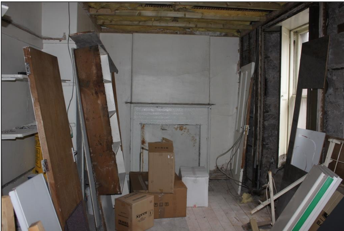
Figure 29b: View of Room 3, 1 st Floor, 14-18 Swan St. From the W
