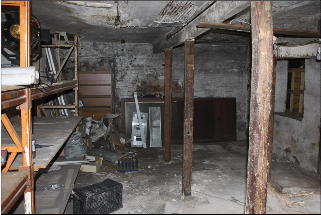
Figure 9a: View of Room 4, Ground Floor, 20a Swan St. From WSW
