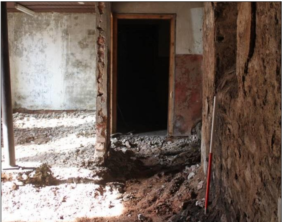
Figure 7b: View of Rooms 2 & 3, Ground Floor, 20a Swan St. From ENE
