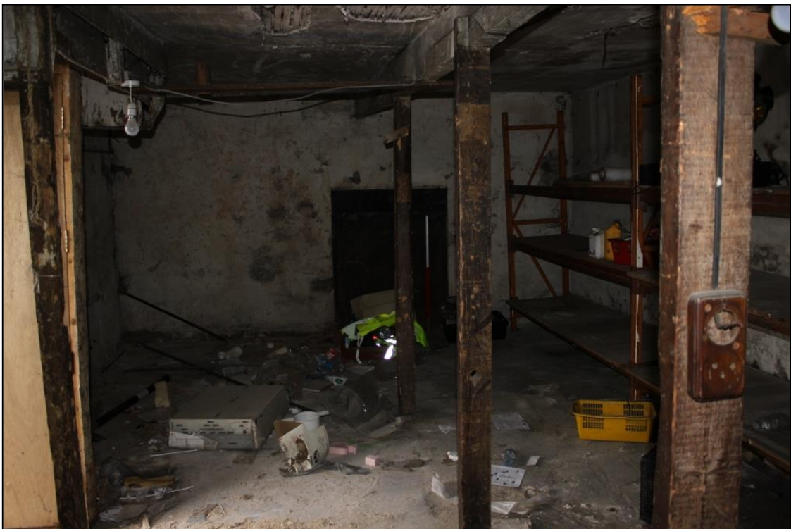
Figure 9b: View of Room 4, Ground Floor, 20a Swan St. From ENE
