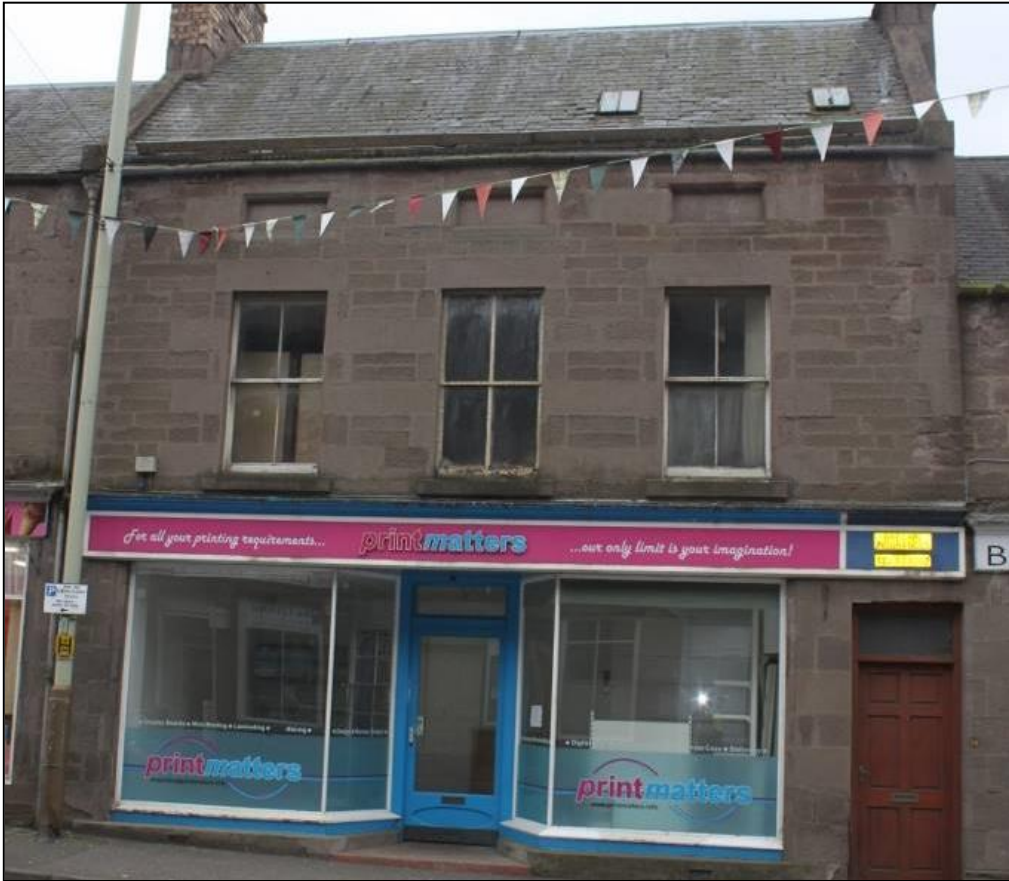
Figure 25a: Front elevation of 14-18 Swan St. From the N
