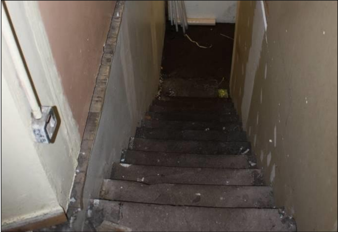
Figure 19a: View of stairs to Basement, Room 1, Swan St. From W
