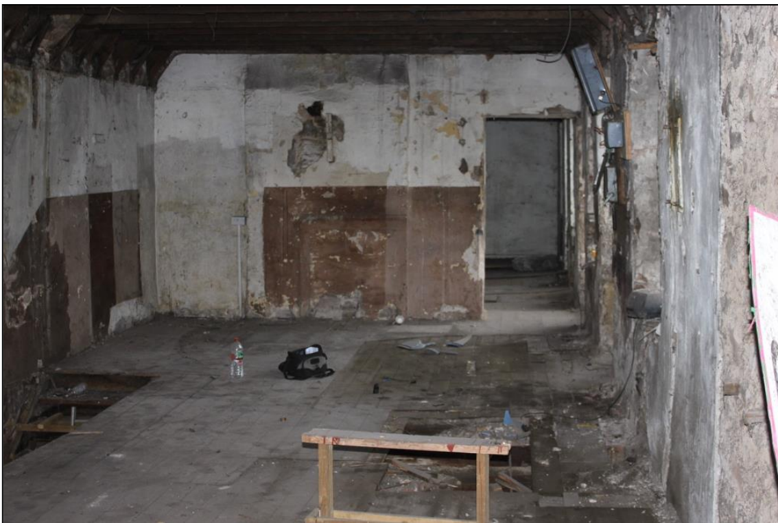
Figure 11b: View of Room 5, 1 st Floor, 20a Swan St. From WSW
