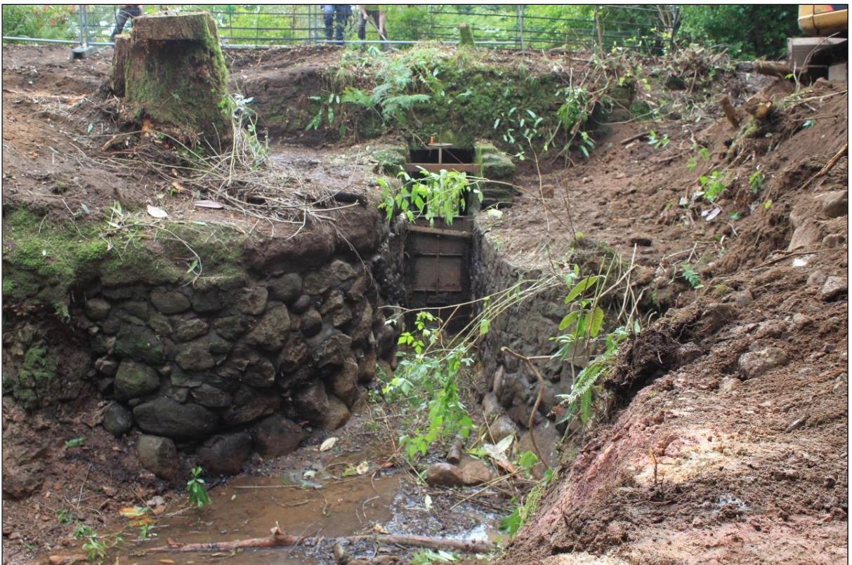
Figure 3: Sluice gate and retaining walls viewed from the north.
