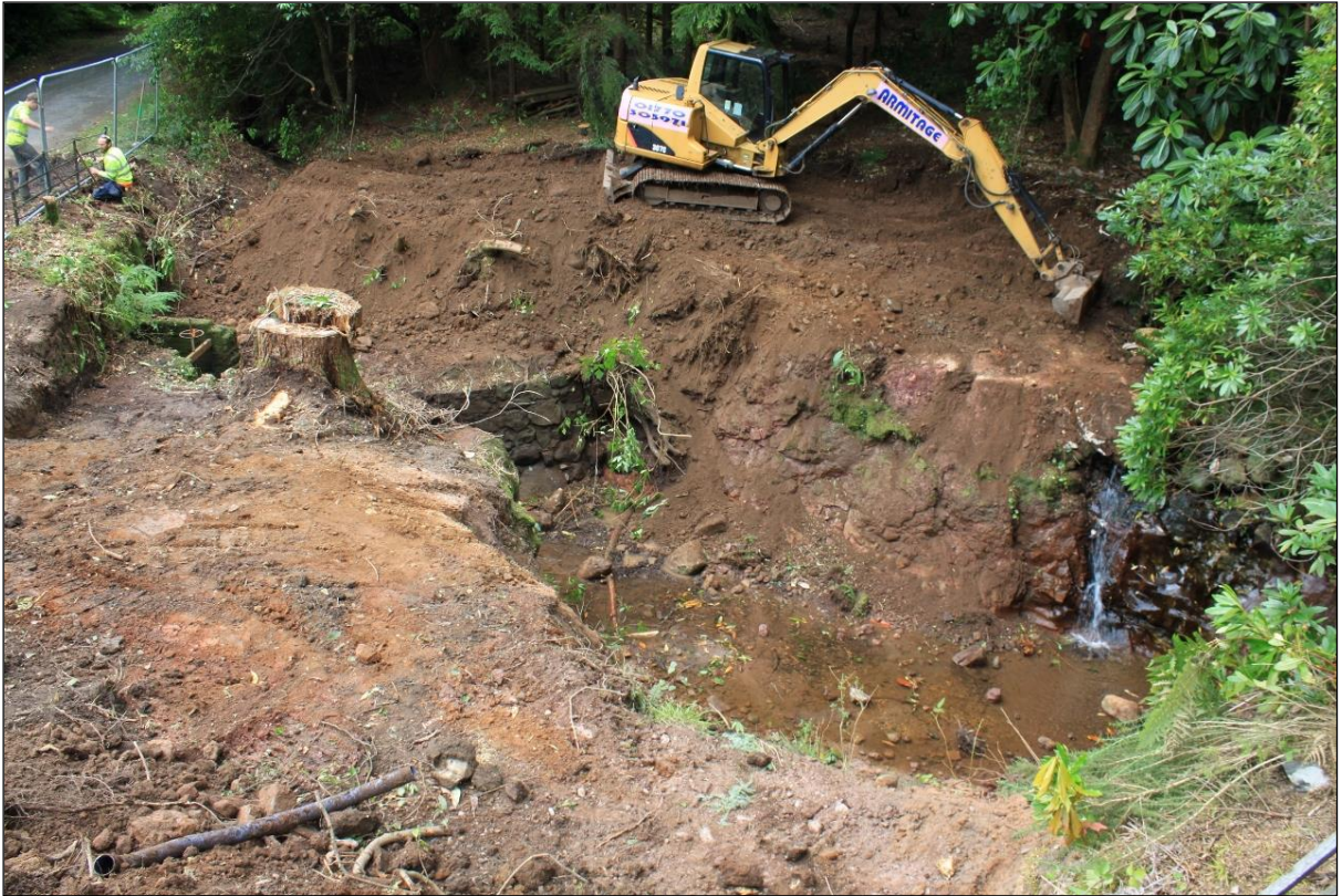
Figure 2: The fire pond viewed from the east during excavation.
