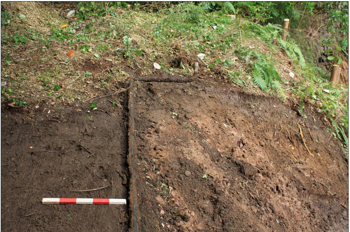
Figure 12: Defunct 2" water main in Area 3.
