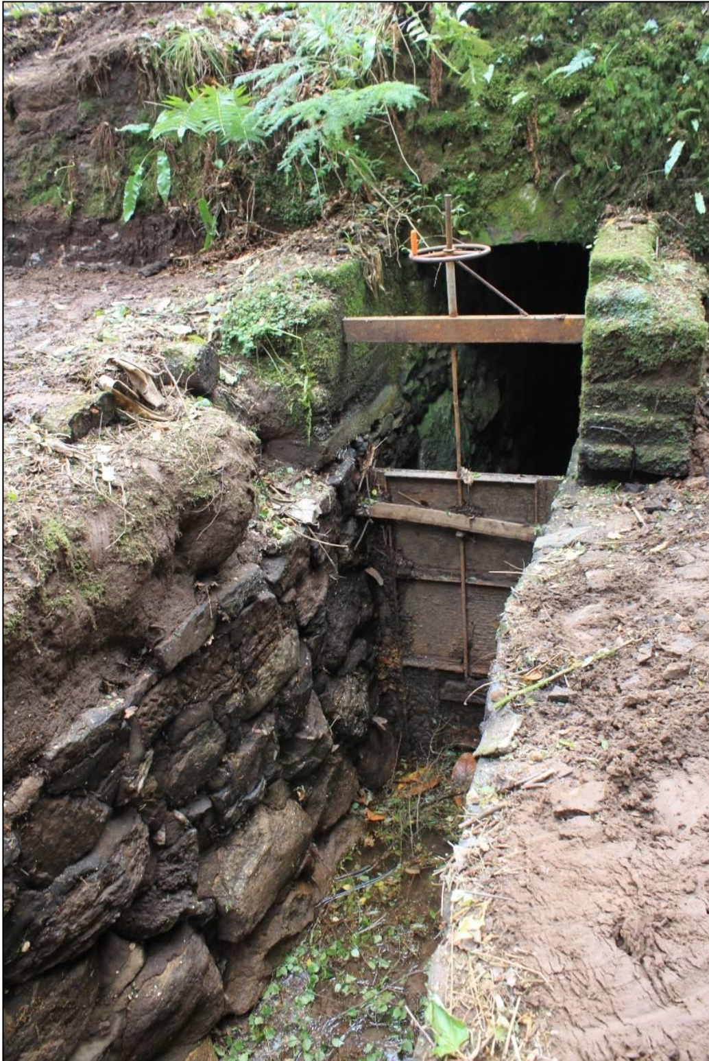
Figure 4: Sluice gate location in relation to the retaining walls.
