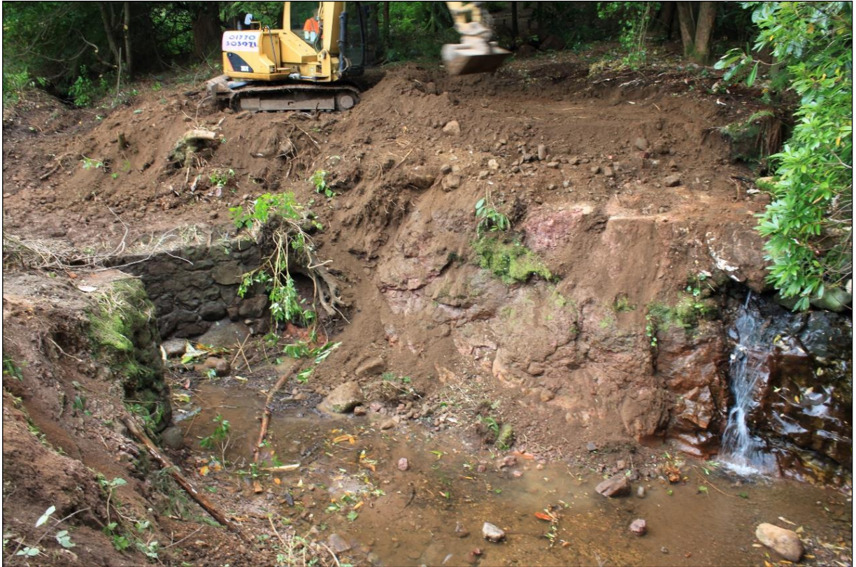
Figure 7: Area 3 during excavation.
