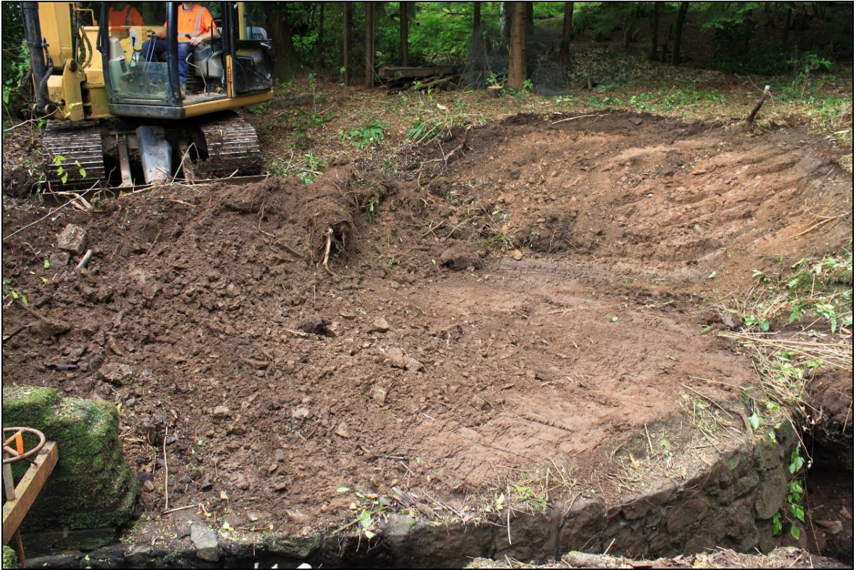
Figure 11: Context (005) during excavation.
