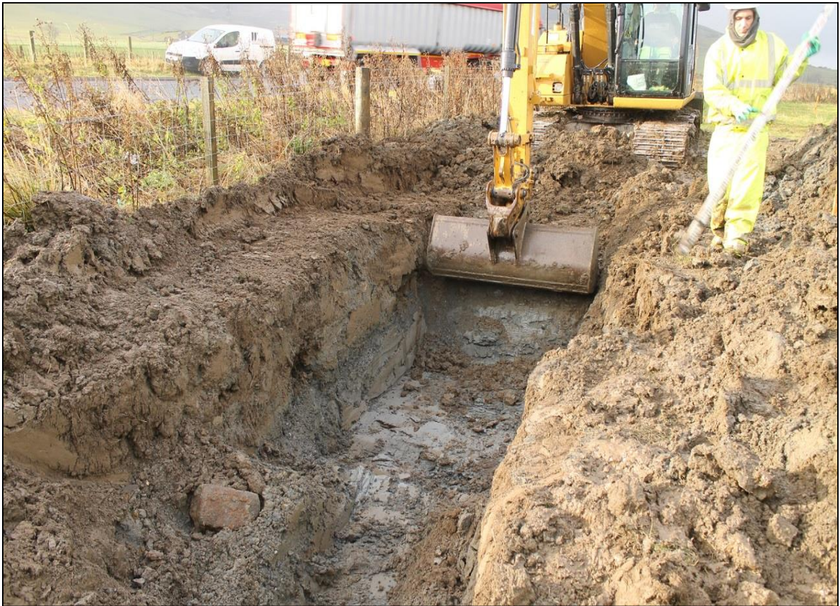
Figure 4a: AREA 1: Surface Water Sewer, working shot at east end
