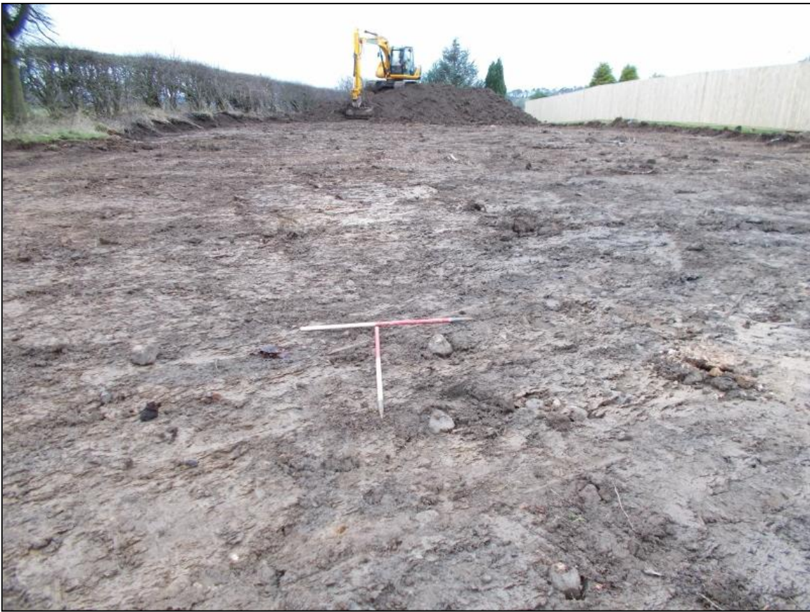
Figure 4a: Southwest plot after stripping from the southeast
