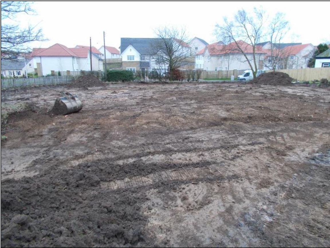
Figure 5a: Northeast plots after stripping from the northwest
