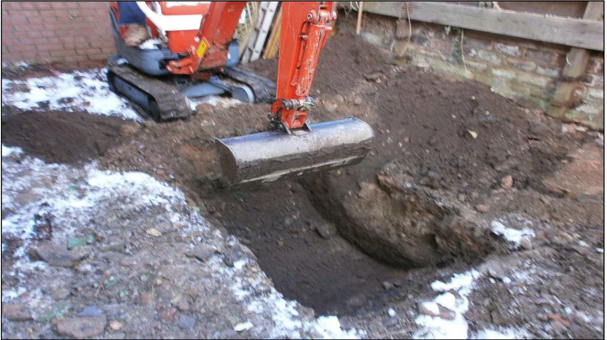
Figure 5a: Working shot of Trench 1
