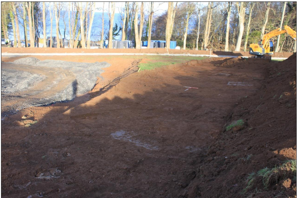
Figure 5b: Monitoring groundworks to the east of Home Farm excavation area.
