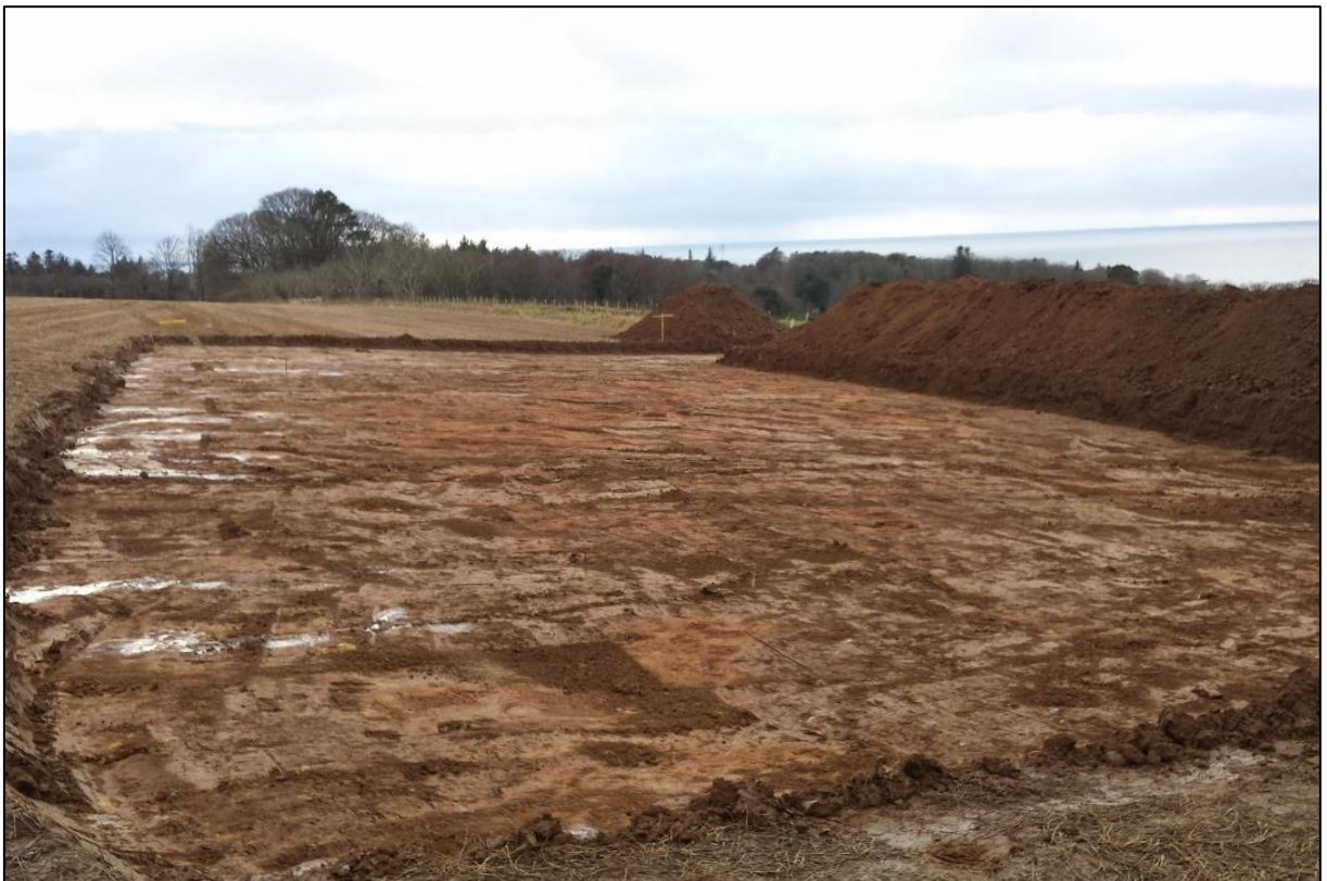
Figure 7b: Monitoring groundworks at Hillhead post-excitation
