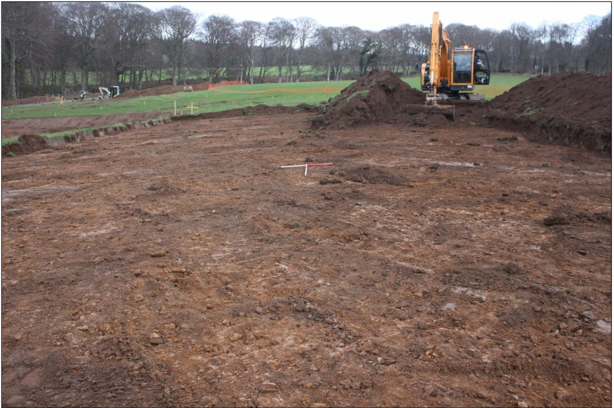
Figure 5a: Monitoring groundworks to the south of Home Farm excavation area.
