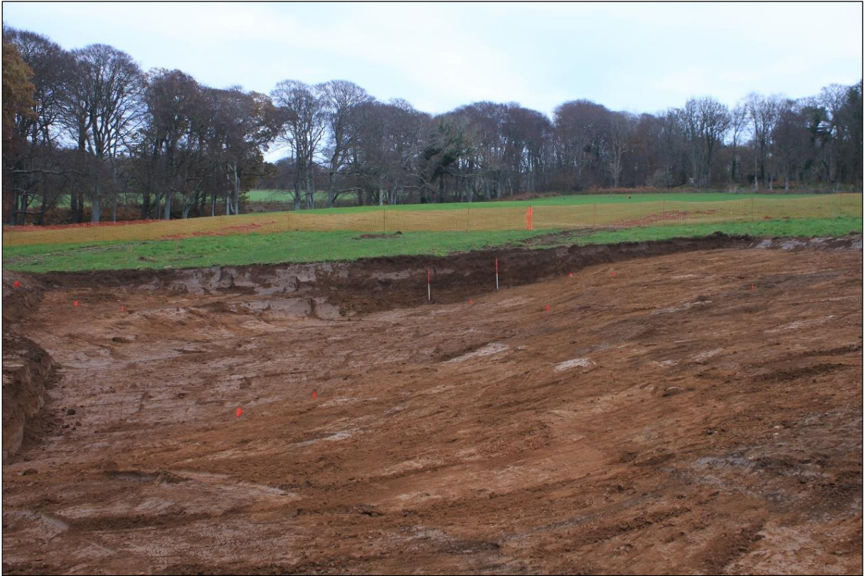
Figure 3a: Palaeochannel from the SW during excavation
