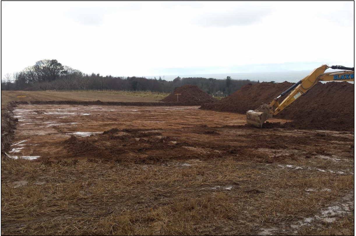
Figure 7a: Monitoring groundworks at Hillhead ongoing
