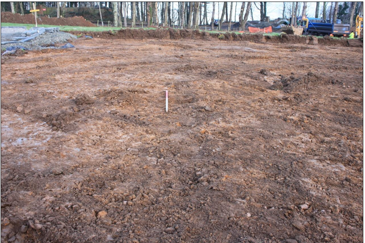
Figure 4b: Rubble field drain (011) revealed during Home Farm Monitoring
