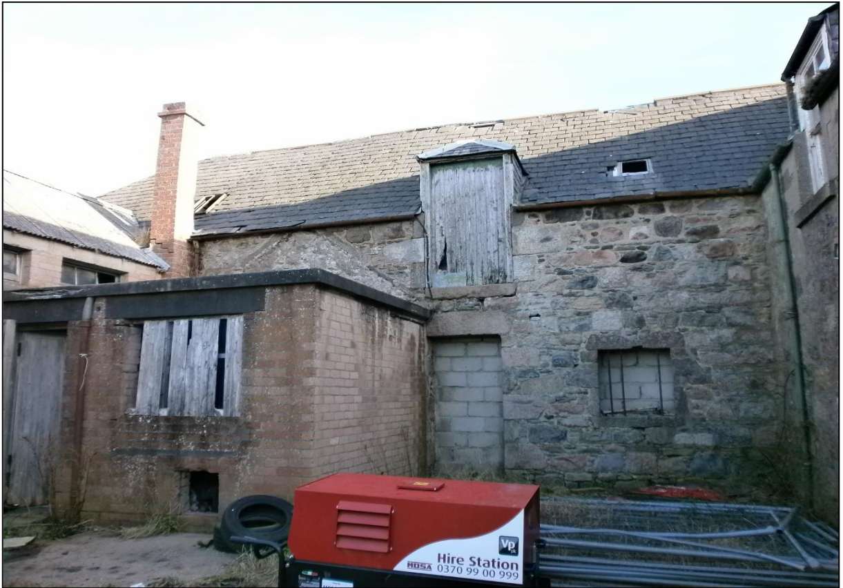
Figure 17a: Building L: exterior, southwest elevation
