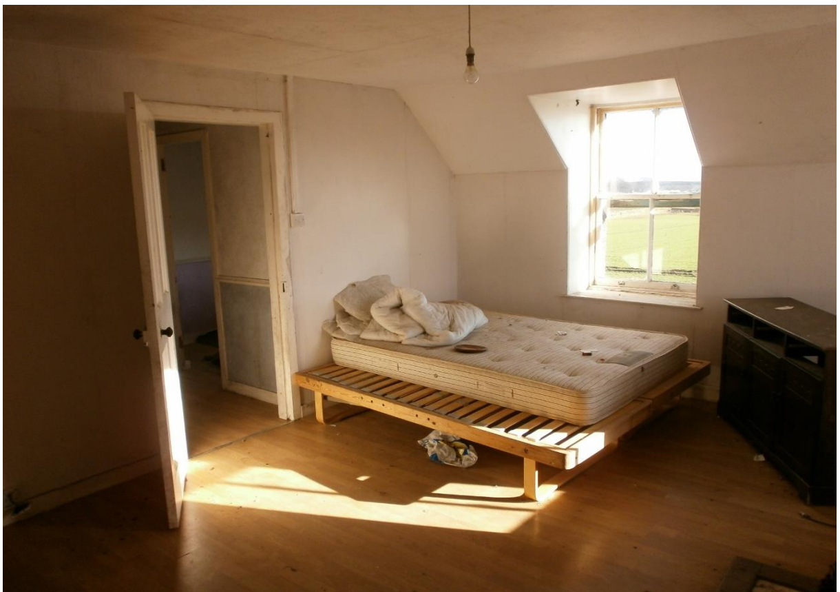
Figure 14b: Building J: Room 2, southeast and northeast walls
