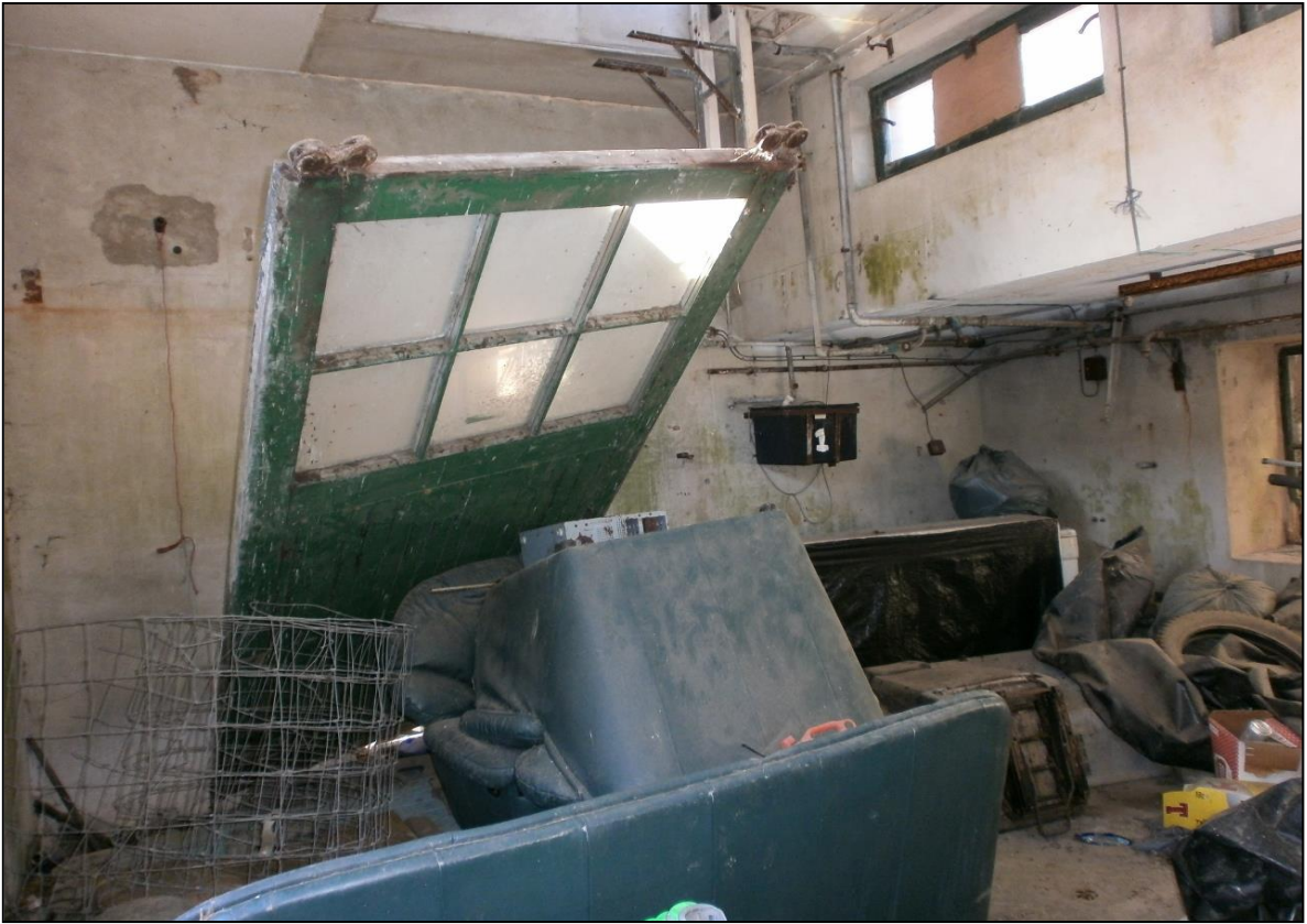
Figure 5a: Building K: Room b.
