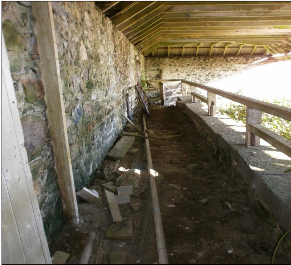
Figure 12a: Raised walkway in along the northwest side of Building H
