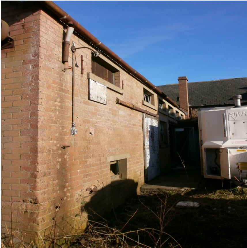
Figure 4a: Building K: southwest elevation modern 20 th century red brick.
