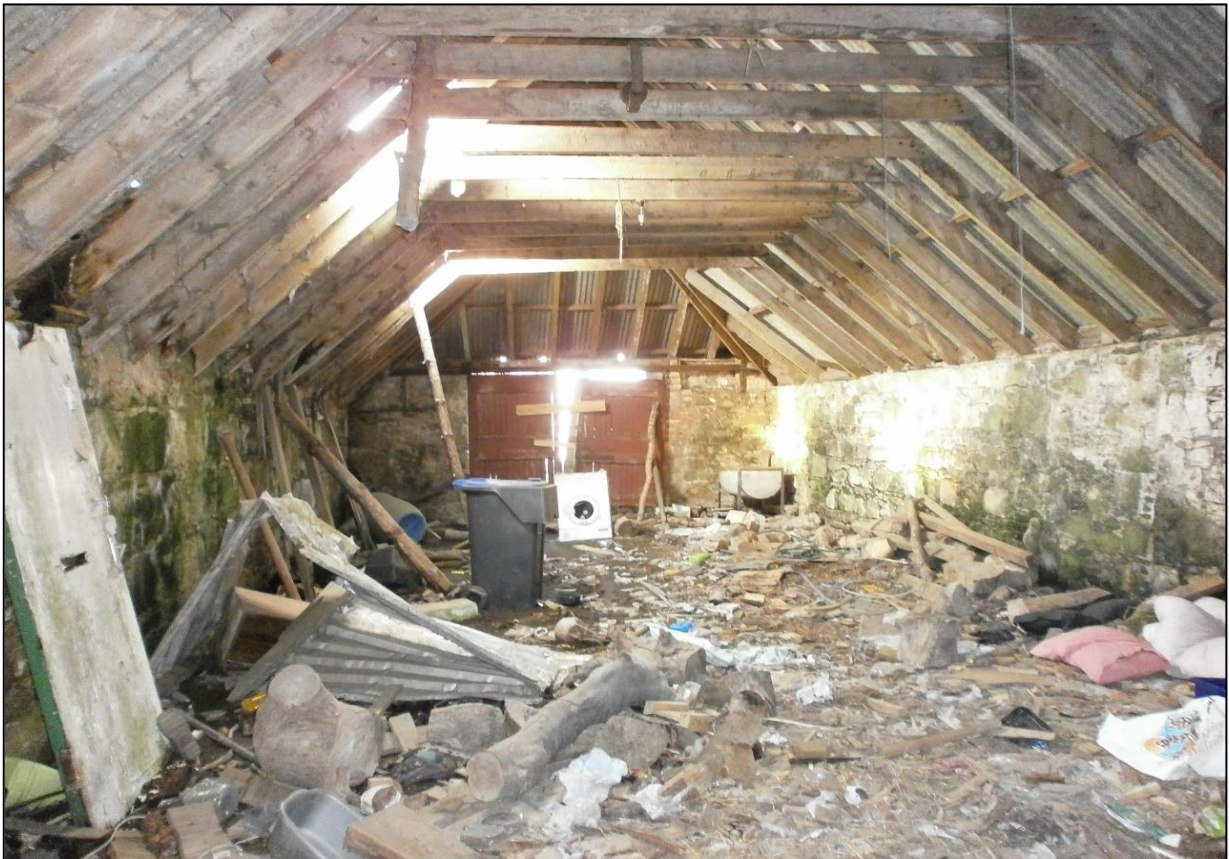
Figure 7b: Building A: showing the interior to the northwest
