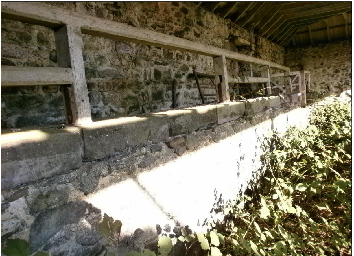
Figure 11b: Raised walkway in along the northwest side of Building H
