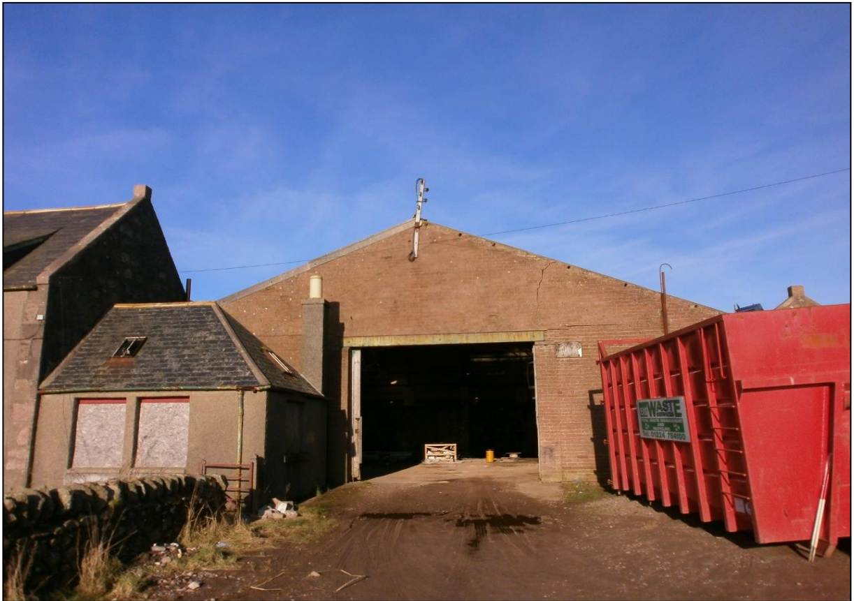
Figure 6a: Building M: exterior southeast elevation showing the modern 20 th century red brick extension.
