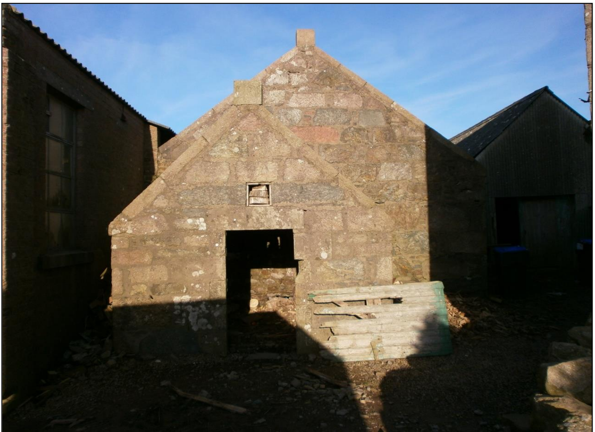
Figure 18b: Annexe on southeast side of Building N.
