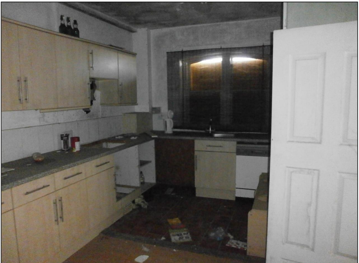
Figure 15b: Building J: Kitchen, southeast and northeast walls
