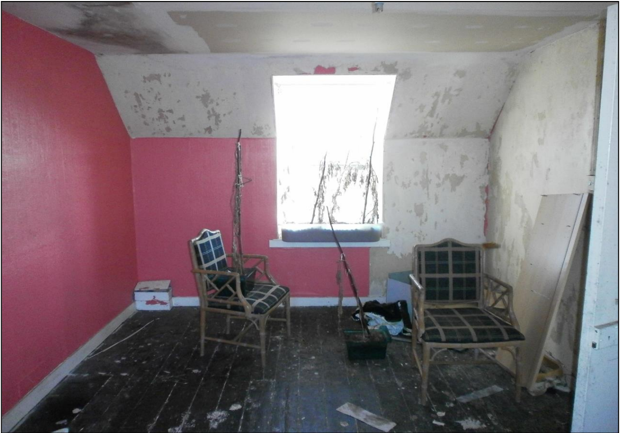
Figure 14a: Building J: Room 1, southeast and northeast walls
