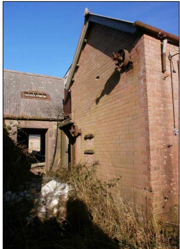
Figure 4b: Building K: Engine (left) and evidence for a former belt driven mechanism (right), suggesting building K was possibly used as a granary or threshing room.
