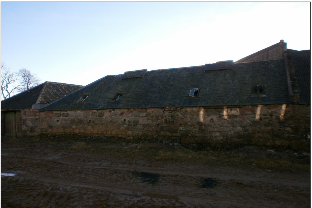
Figure 8b: Building B: exterior northwest elevation
