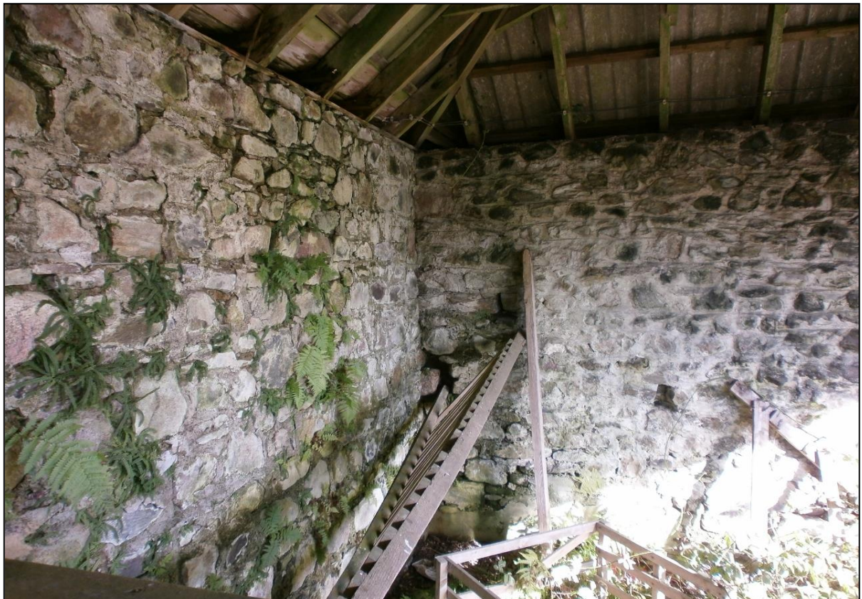
Figure 12b: Evidence for whitewash on the interior walls
