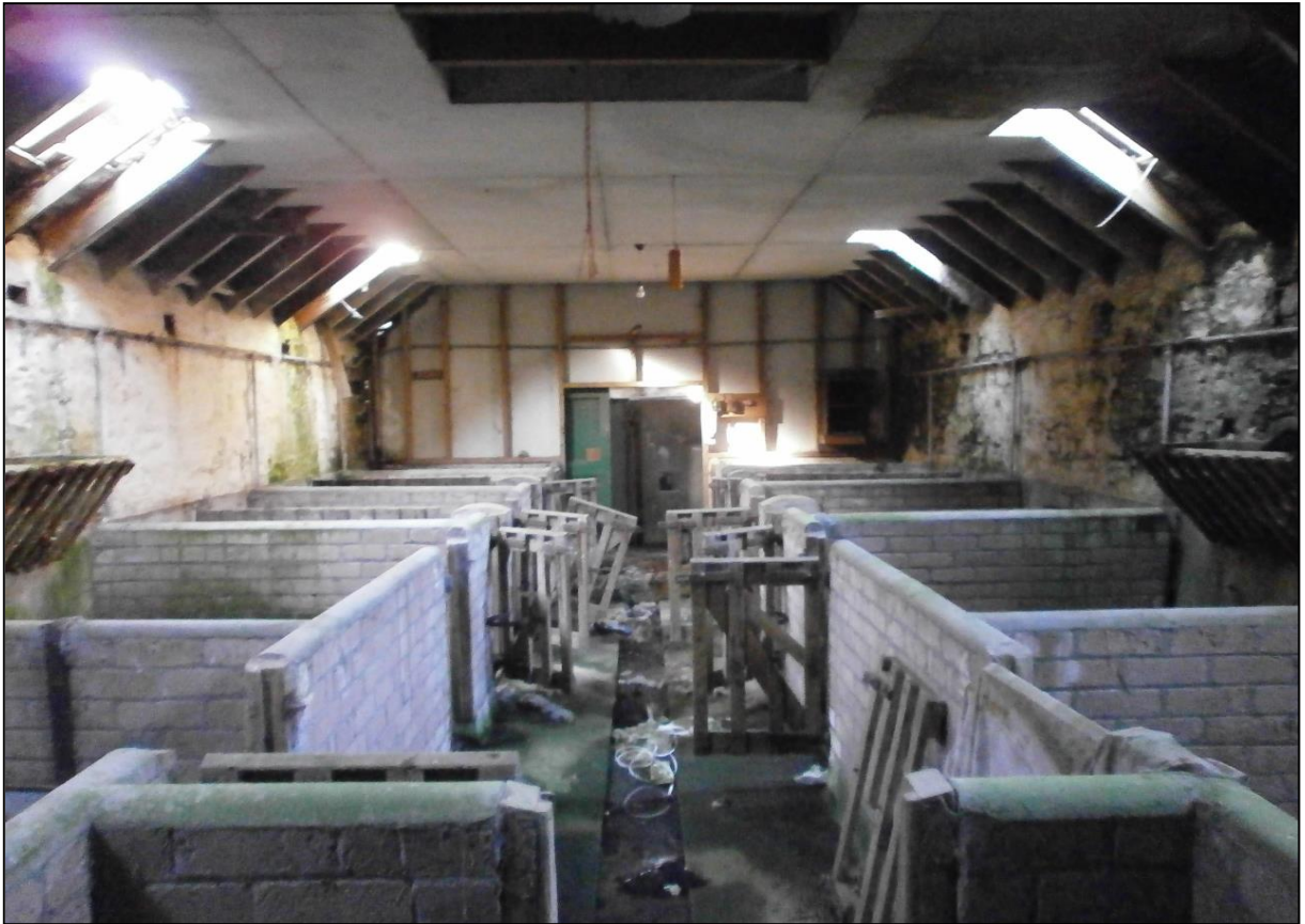
Figure 18a: Building N: view along the room to the northwest.
