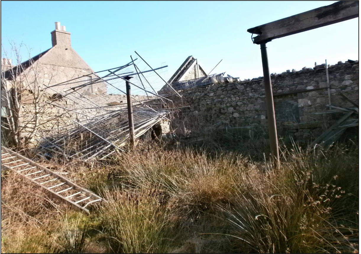
Figure 11a: Building H: southeast side
