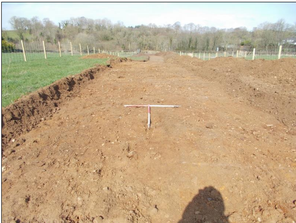
Figure 3b: Shot of pipeline route showing subsoil (003)
