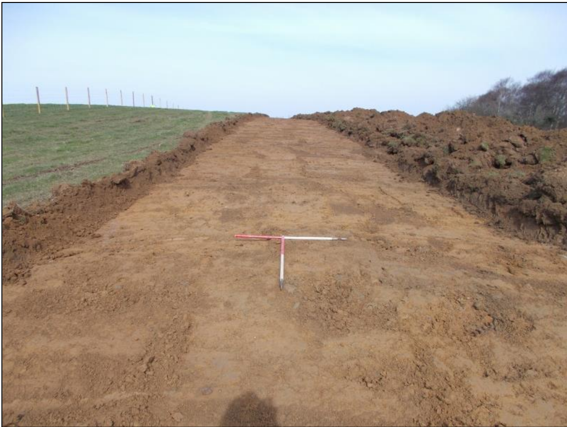
Figure 3a: Shot of pipeline route showing subsoil (002)
