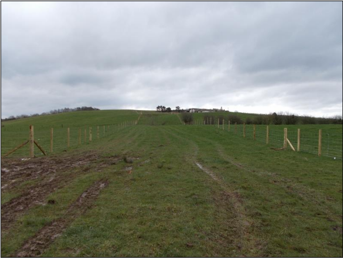
Figure 2a: Pre-excitation shot along route of pipeline from the north, with Barclaugh Farm visible at the top of the hill
